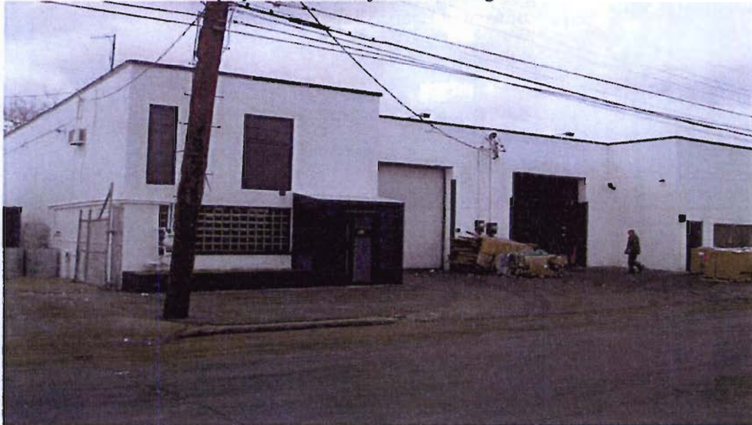
Display of front of adjacent building on Site F
