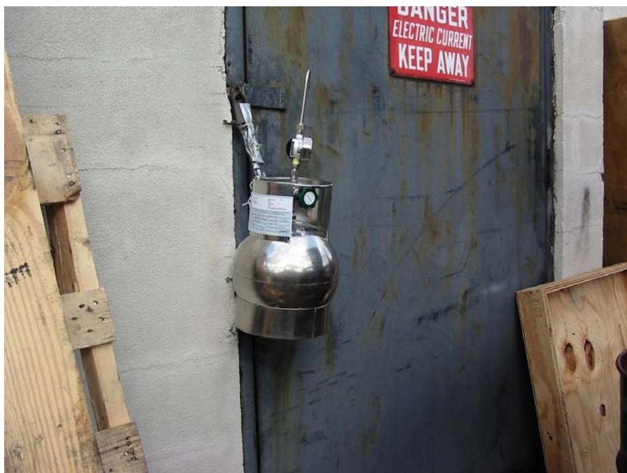
Sampling Structure 1 Outdoor Air
