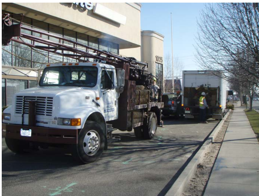
Monitoring Well Installation
