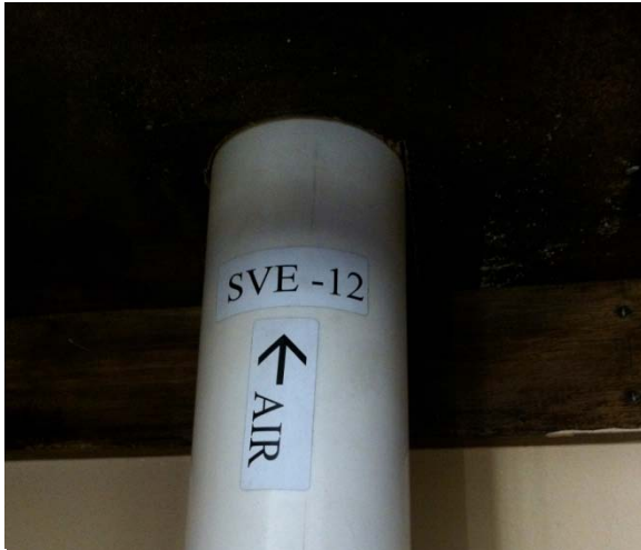
Typical label at suction point (SVE-12 shown)
