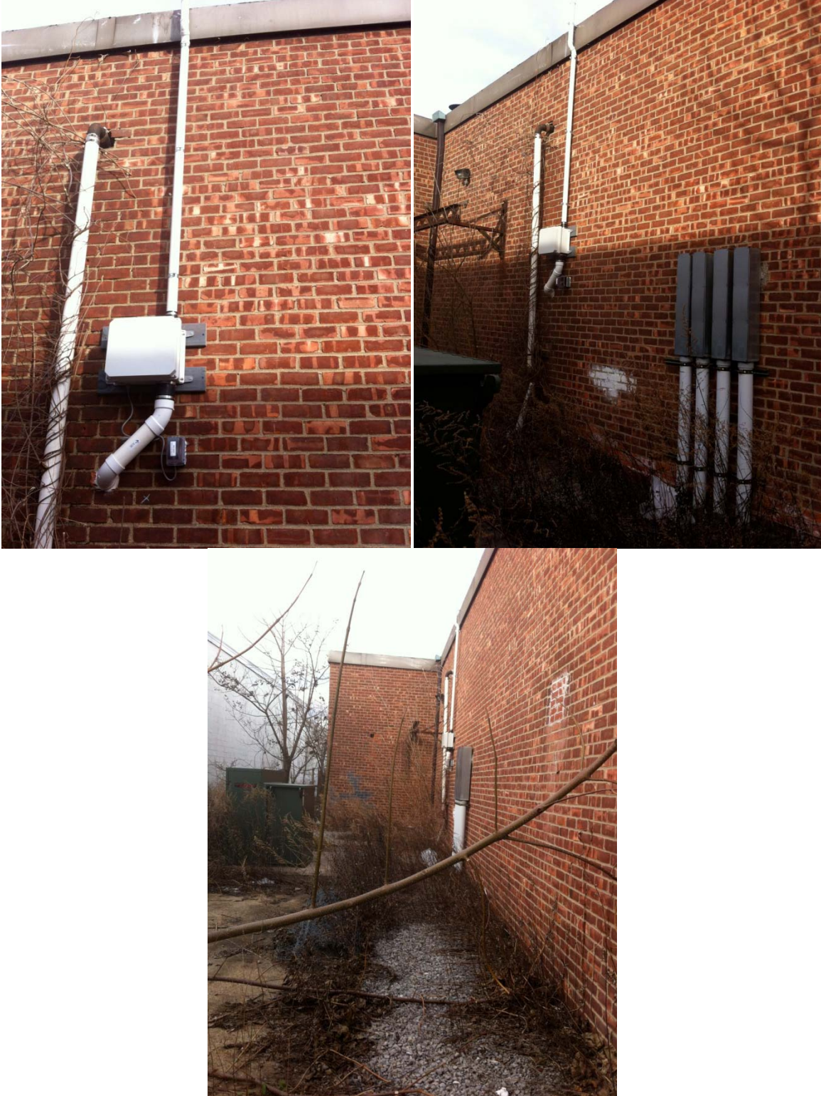
Typical fan, electrical outlet and exhaust mounting (System 1 shown.)
