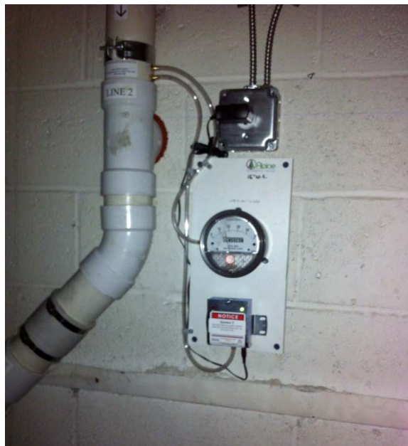
Typical pressure gauge, audible alarm (with outlet) and exterior wall protrusion (System 2 shown)
