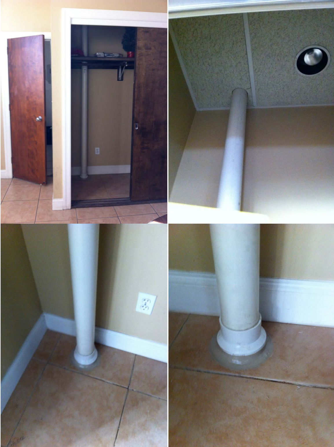
Typical vertical piping, with protrusion through drop ceiling, and suction point seal (SVE-12 shown )
