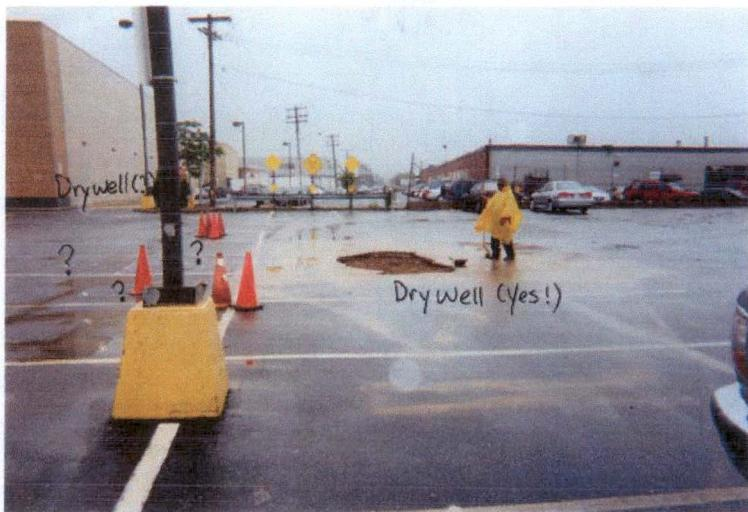
Photo 3. Two Drywell Location at 101 Frost Street, identified by Ground Penetration Radar and confirmed by surface excavation (just backfilled).
