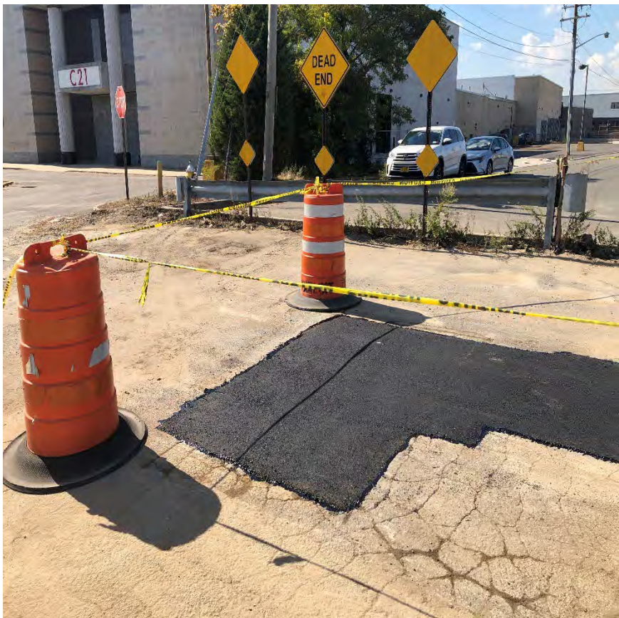
October 12, 2023 Backfilled excavation and restored asphalt
