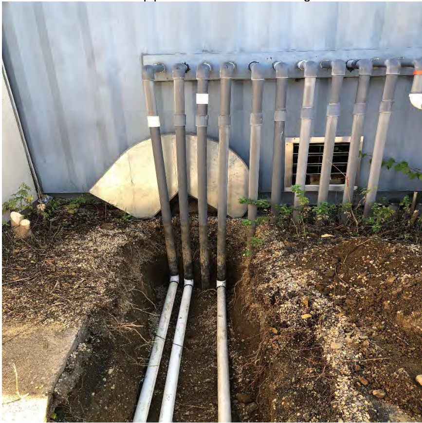
October 5, 2023 New pipes' connection at system
