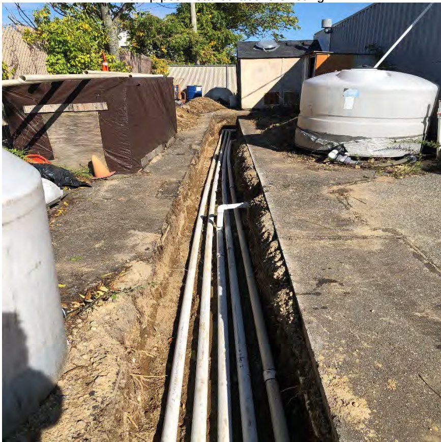
October 5, 2023 New pipes installed above existing
