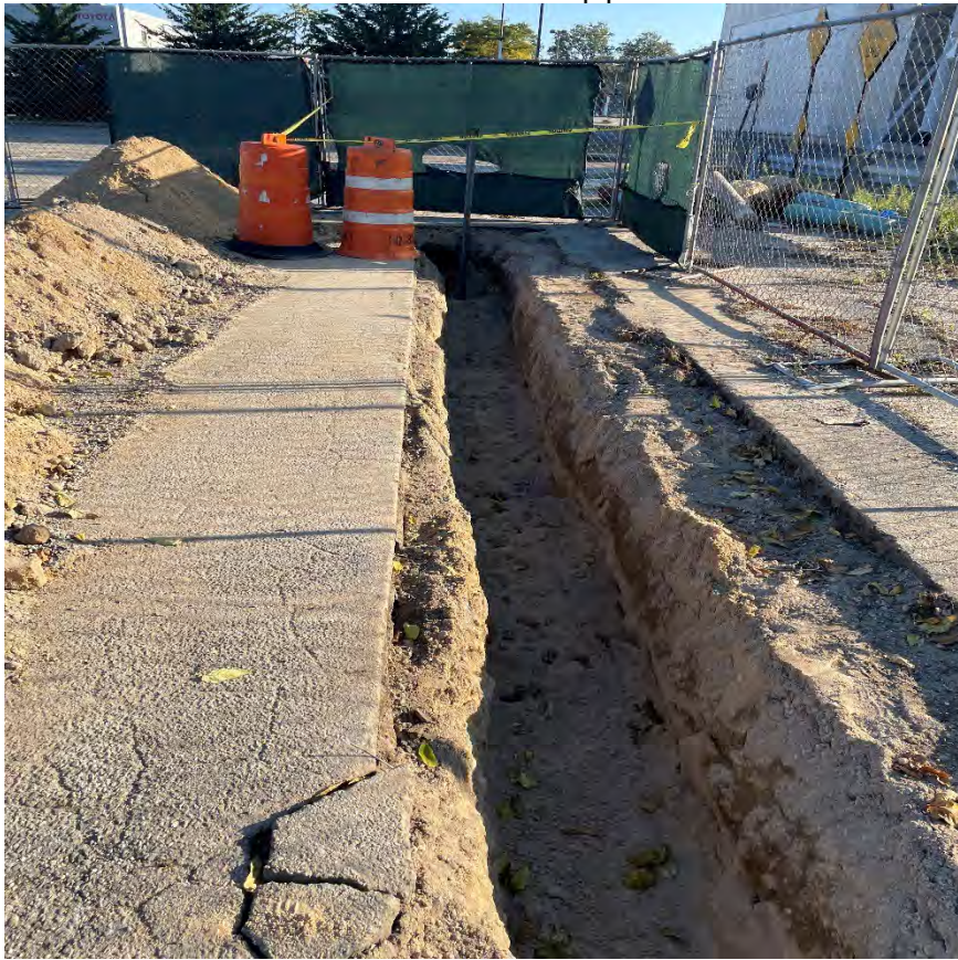
October 4, 2023 Excavation for new pipe
