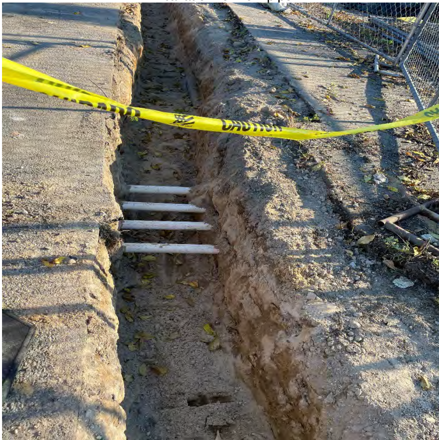
October 4, 2023 Excavation for new pipe
