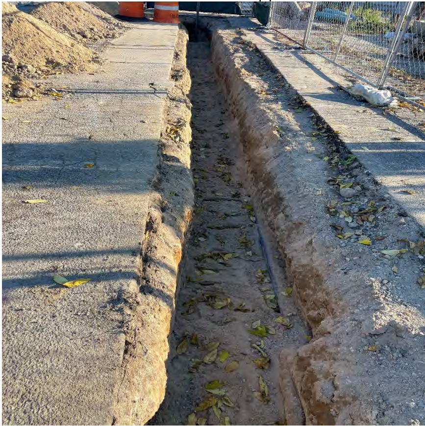
October 4, 2023 Excavation for new pipe
