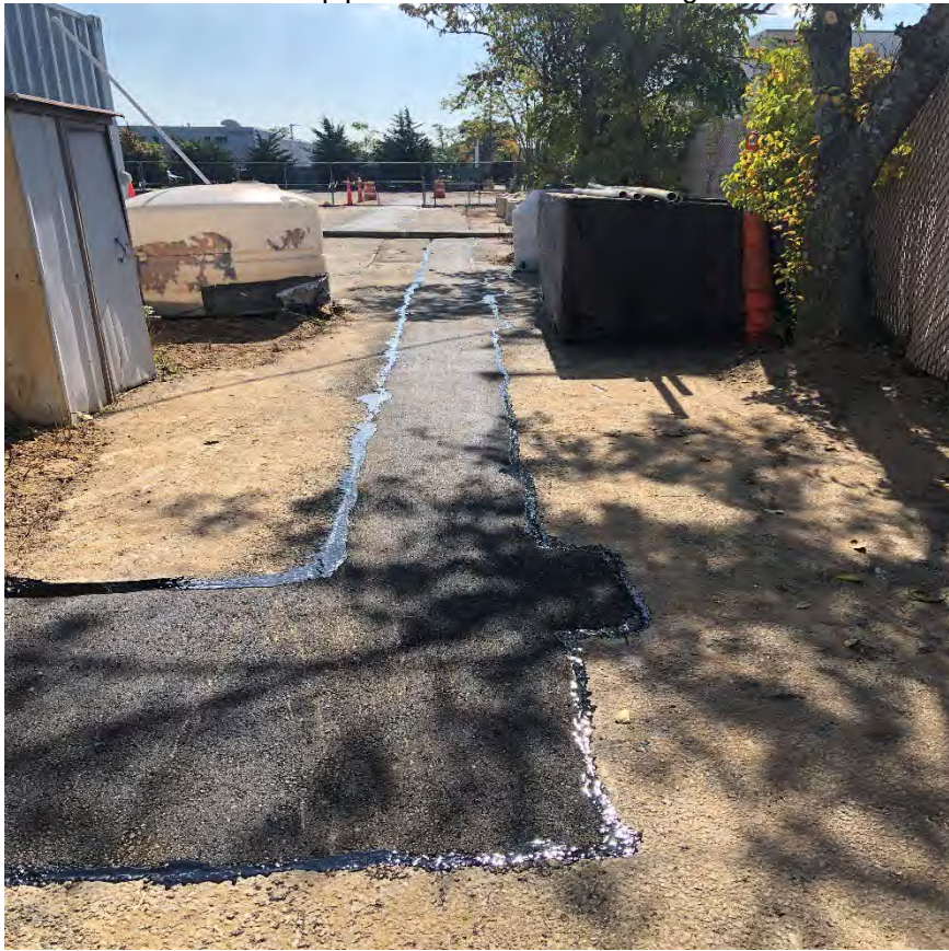
October 12, 2023 Backfilled excavation and restored asphalt
