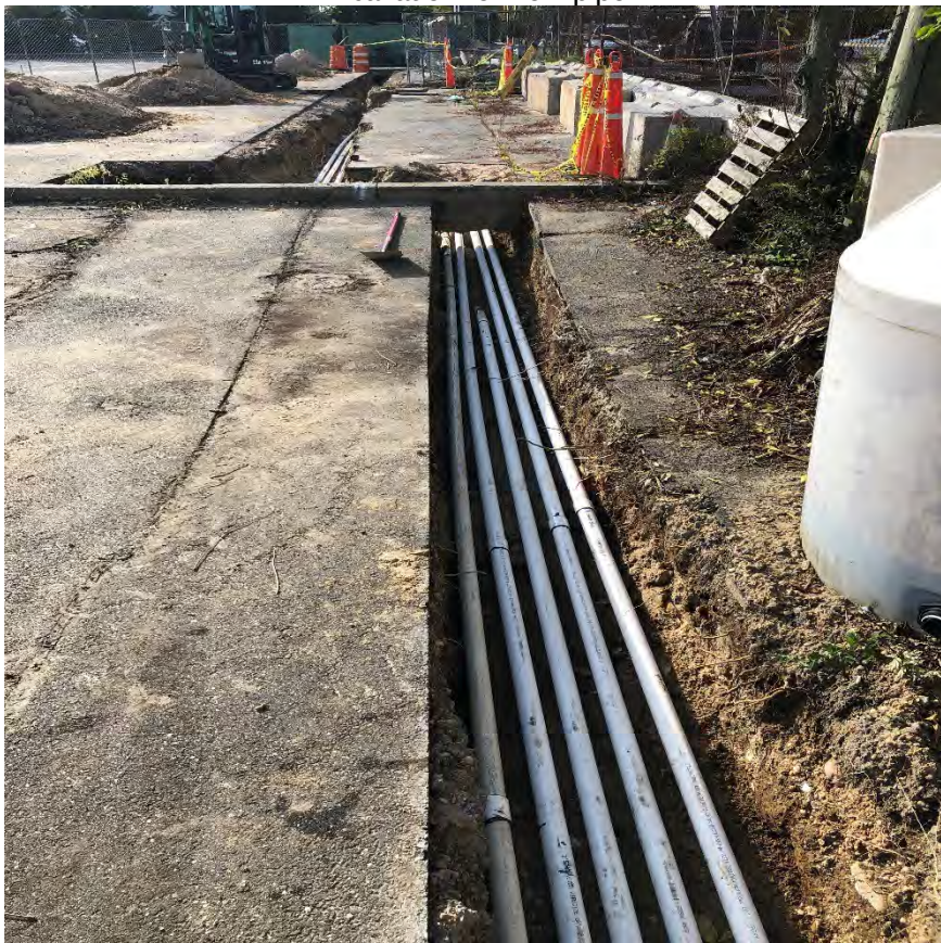
October 5, 2023 New pipes installed above existing
