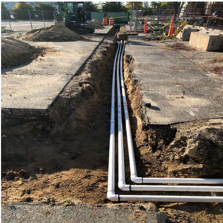
October 5, 2023 New pipes installed above existing
