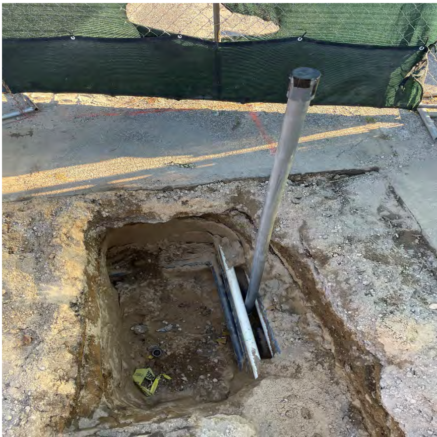
October 4, 2023 Excavation for new pipe
