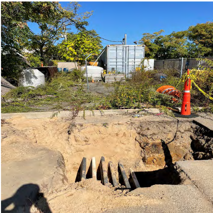
October 3, 2023 Test pits to find location of air leaks
