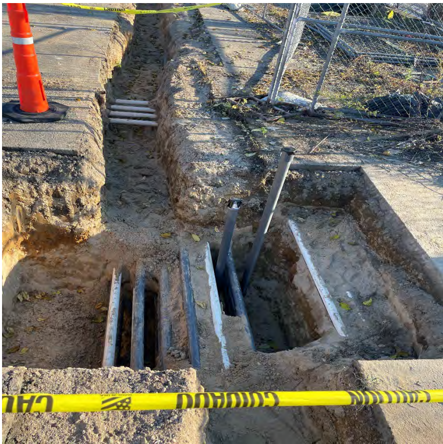
October 4, 2023 Excavation for new pipe
