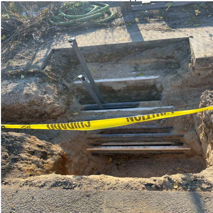
October 4, 2023 Excavation for new pipe
