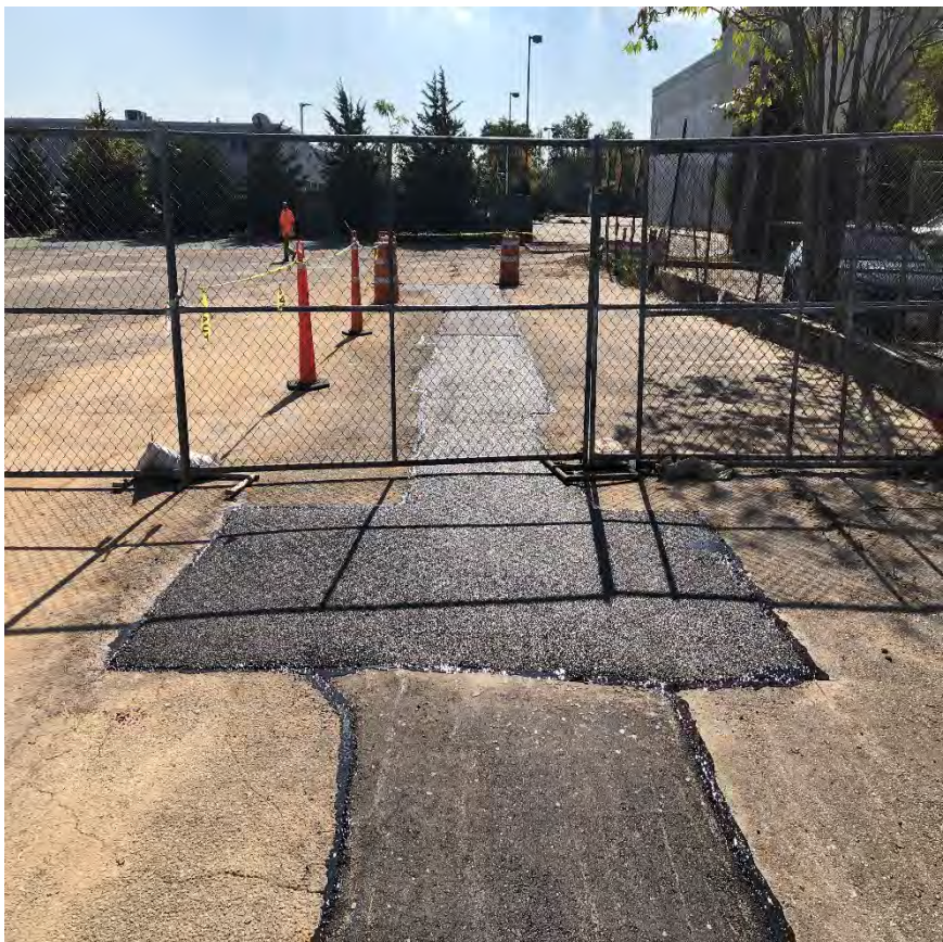
October 12, 2023 Backfilled excavation and restored asphalt
