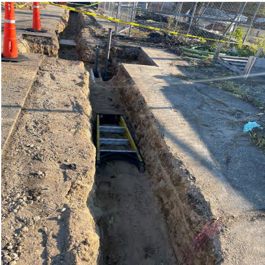
October 4, 2023 Excavation for new pipe
