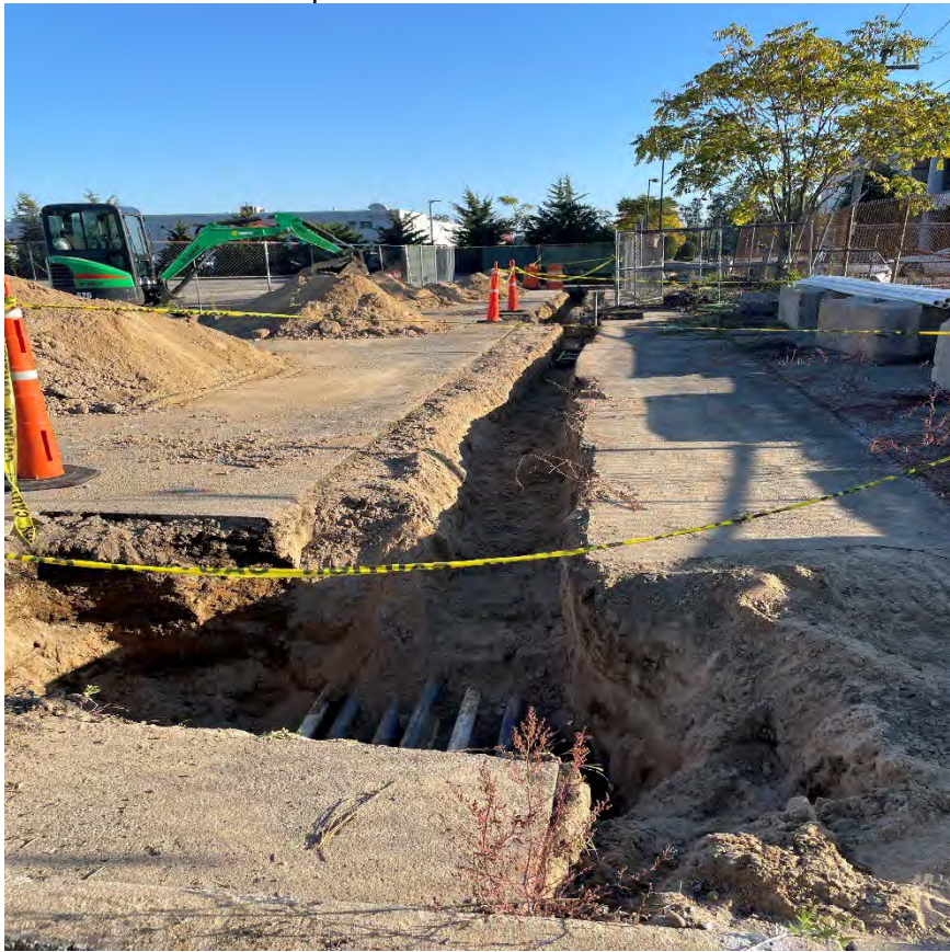
October 4, 2023 Excavation for new pipe
