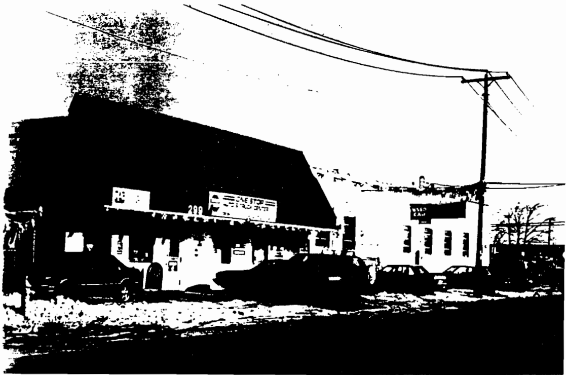
2. Close up view of front of subject building.
