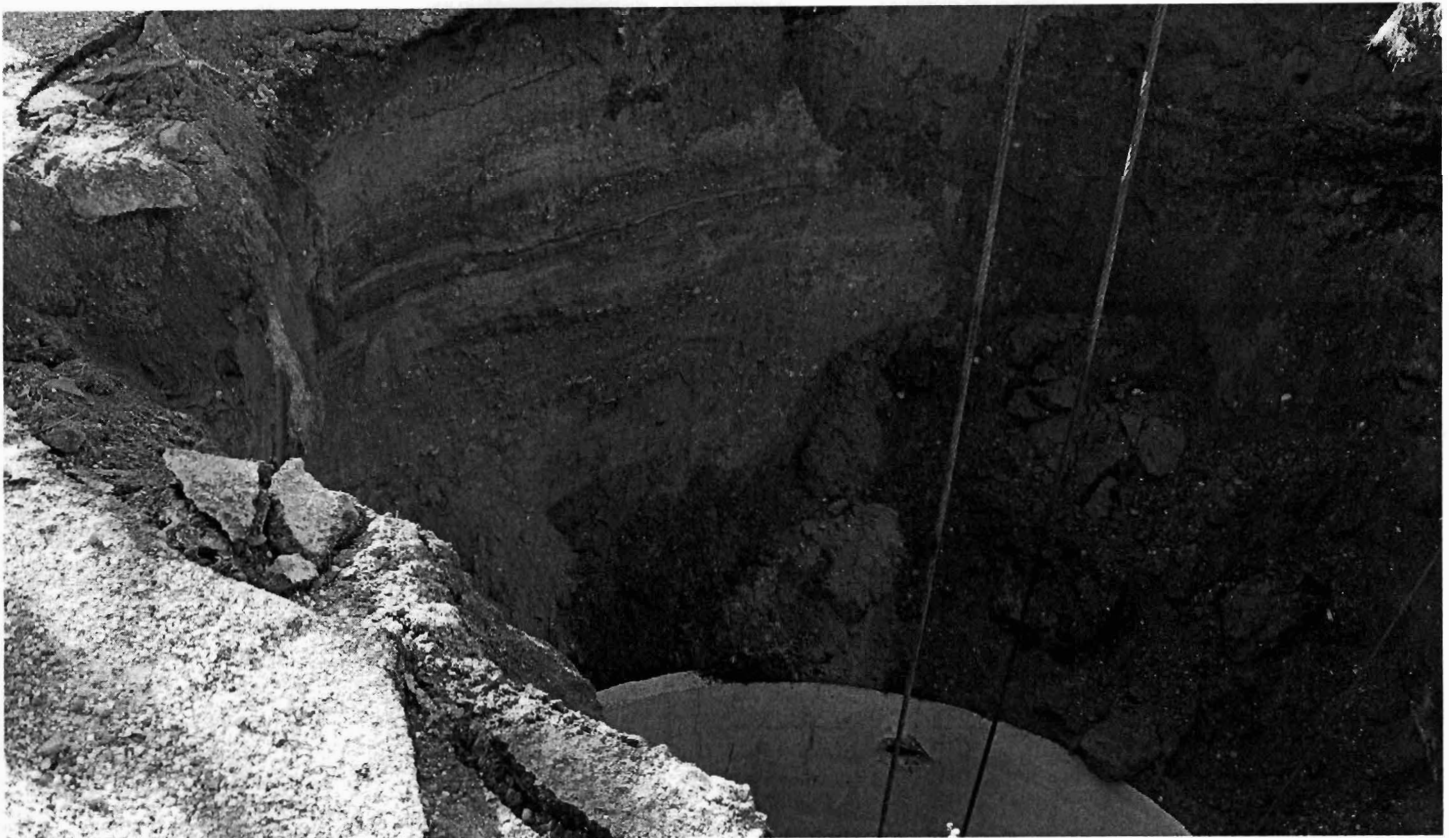
299 Main Street - Excavation of drywell OF-1.
