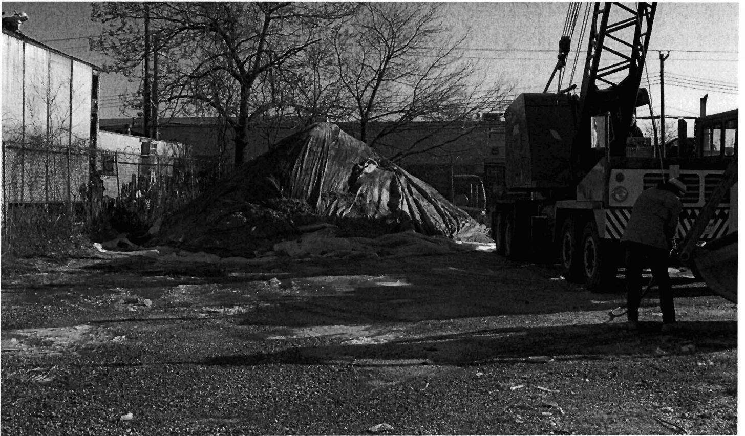
299 Main Street - Stockpile of excavated soil from drywell OF-1.
