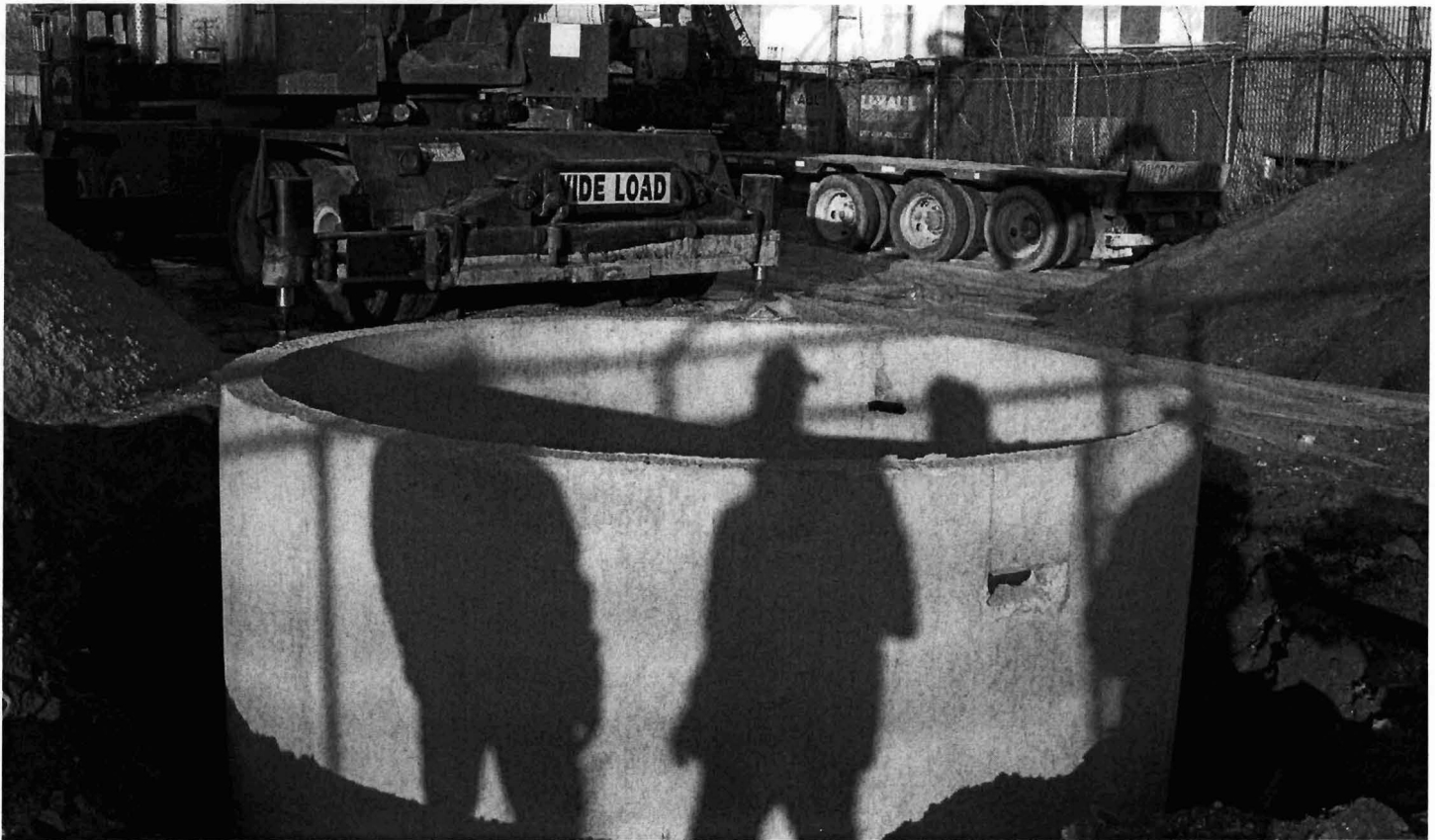
299 Main Street - Installation of oversized concrete rings during remediation drywell OF-1
