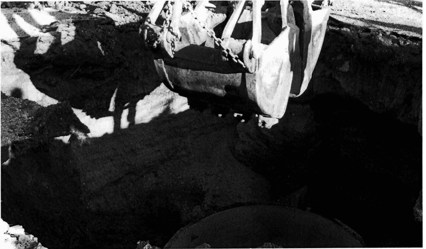
299 Main Street - Excavation of drywell OF-1.
