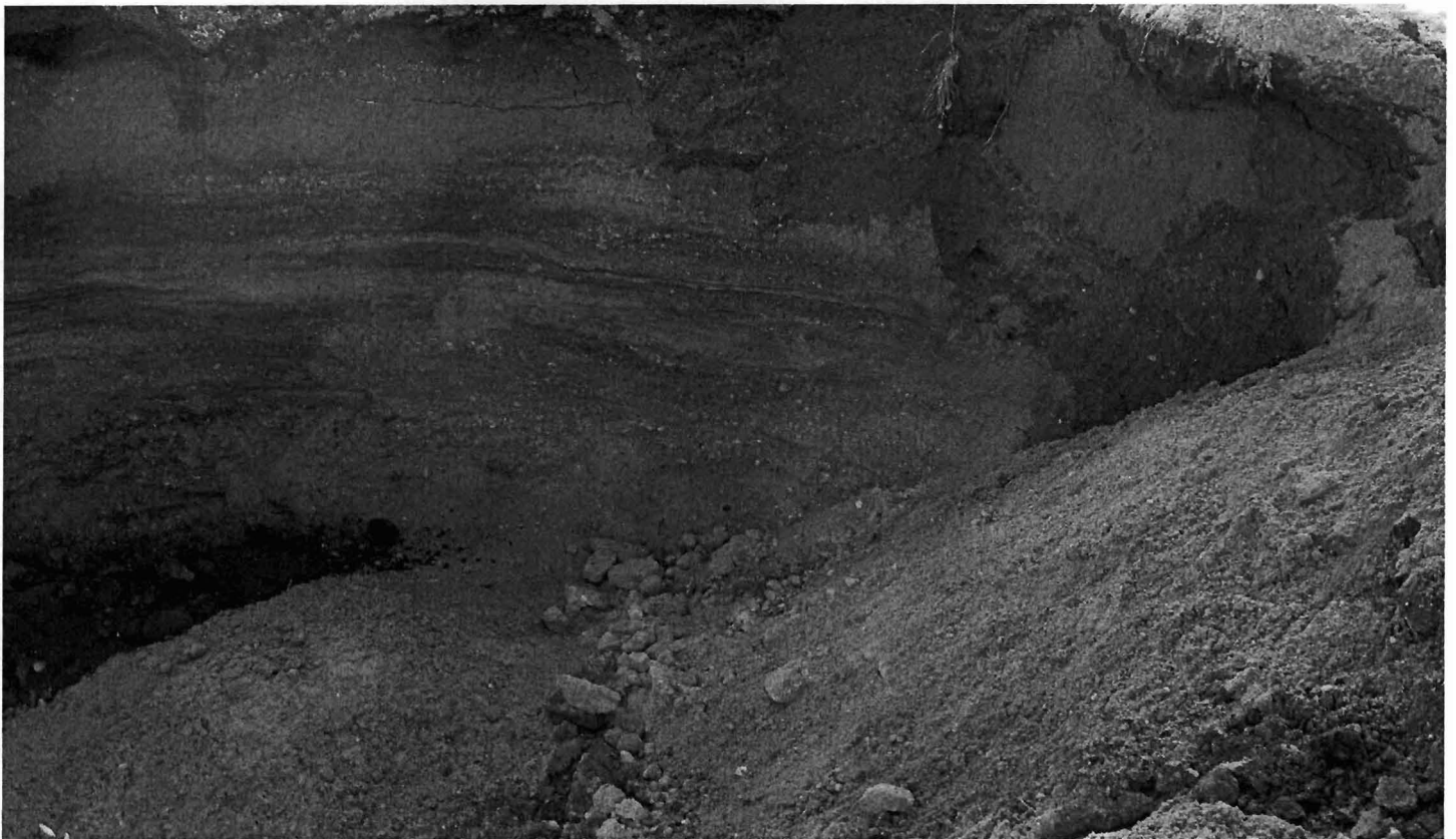
299 Main Street - Backfilling of drywell OF-1.
