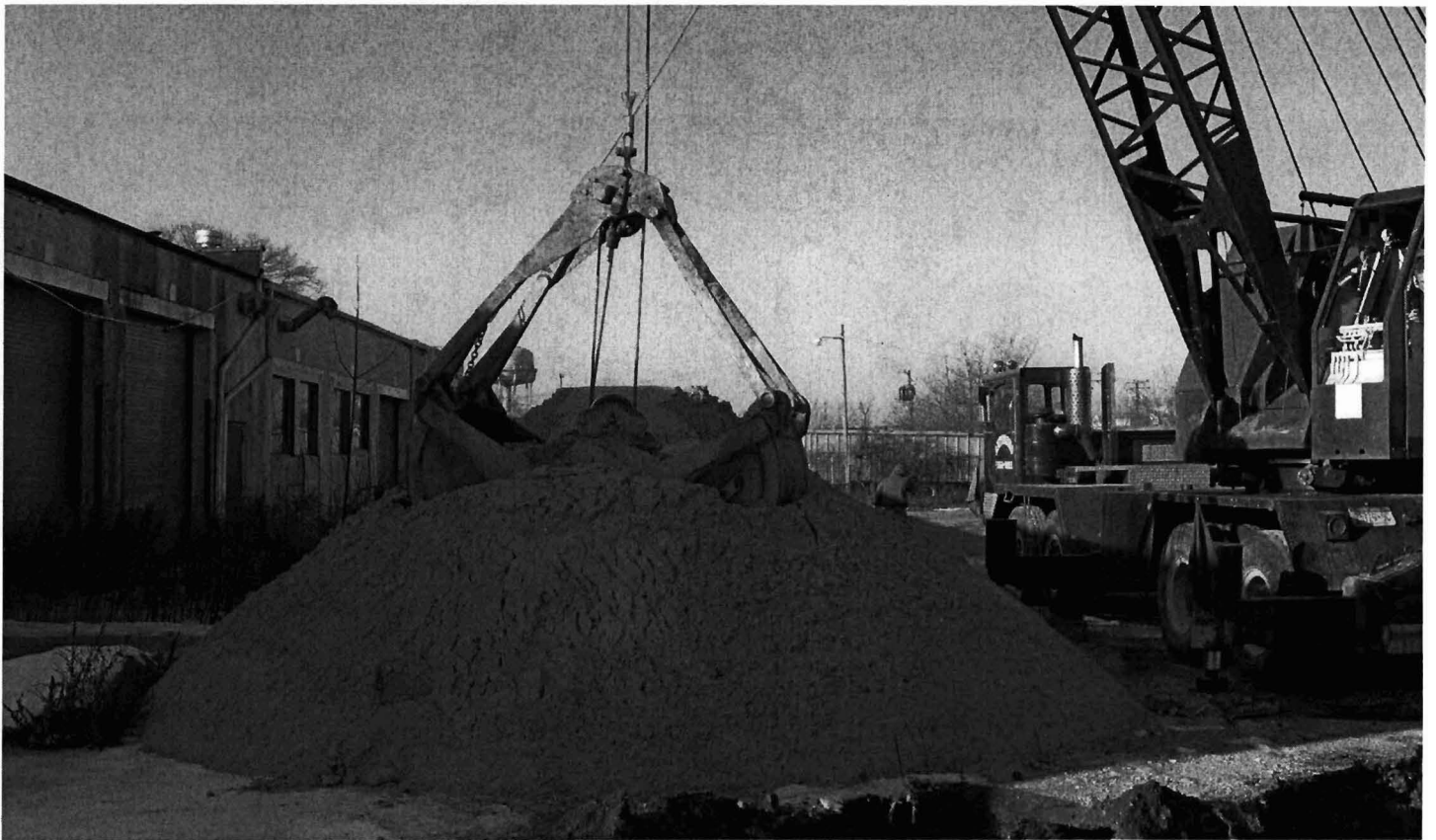
299 Main Street - Installation of clean imported sand during the backfilling of drywell OF-1
