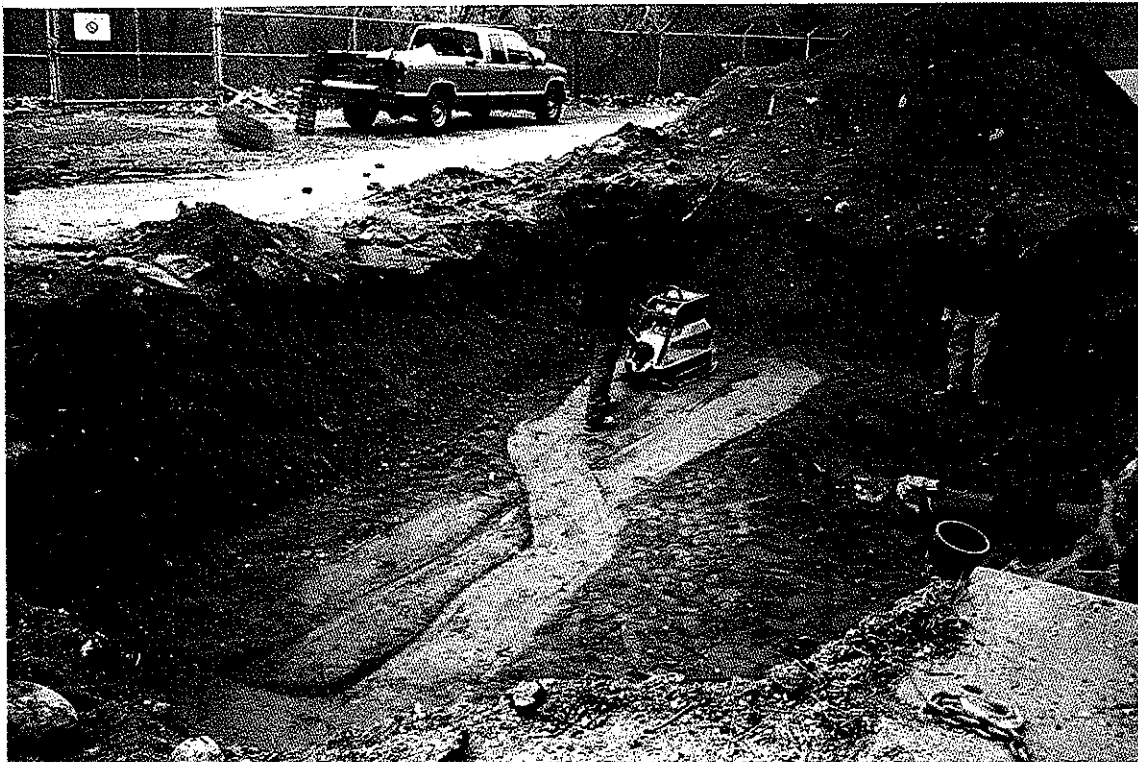
Compacting of Soil Prior to Pouring of Concrete
