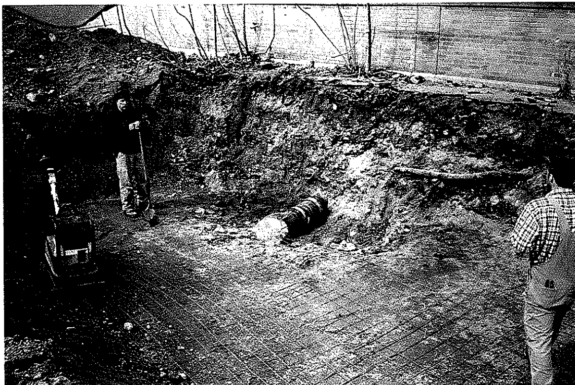
Installation of Wire Mesh
