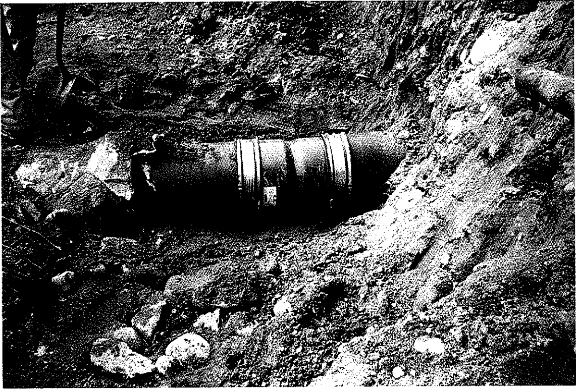
Repair To Drain Pipe
