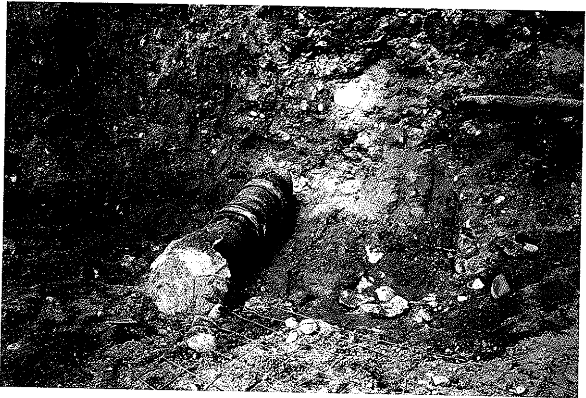
Repair To Drain Pipe
