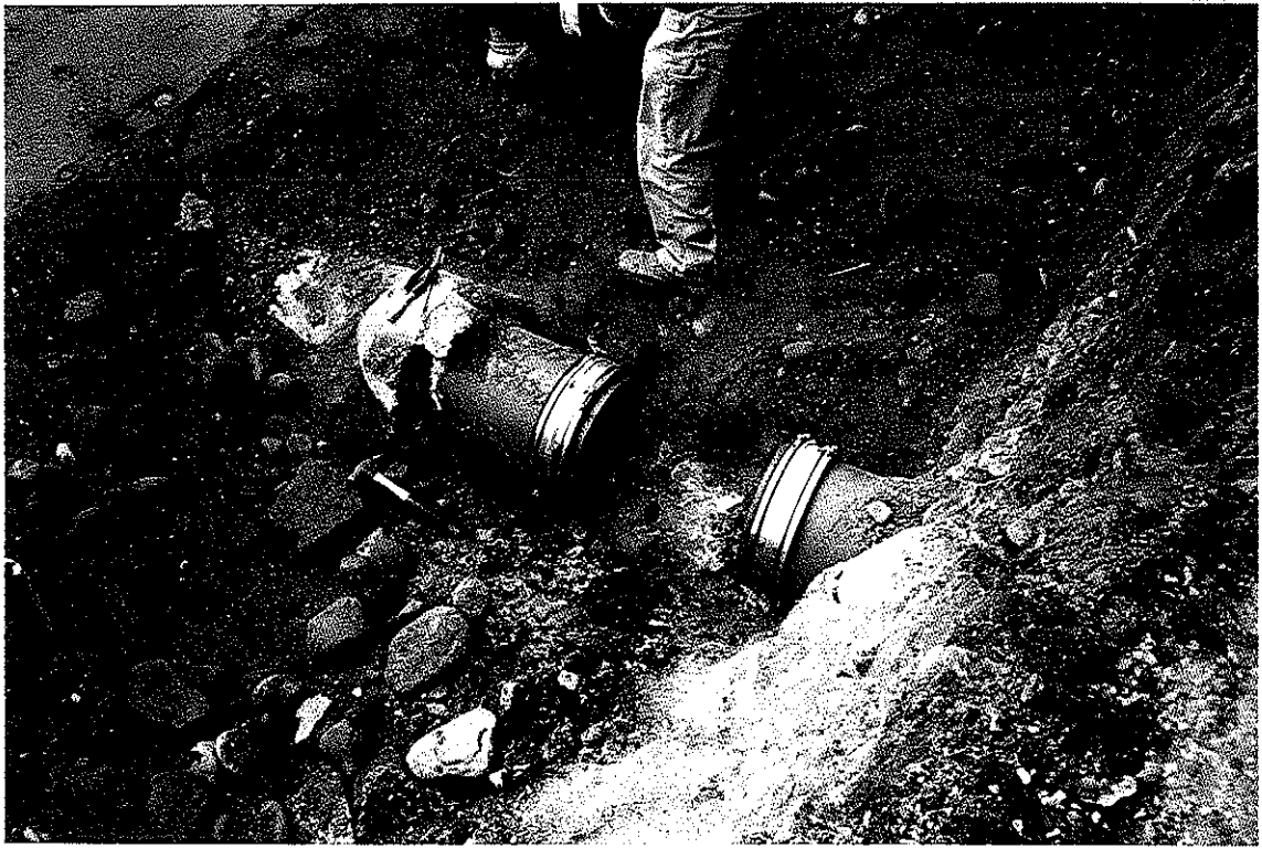
Repair To Drain Pipe
