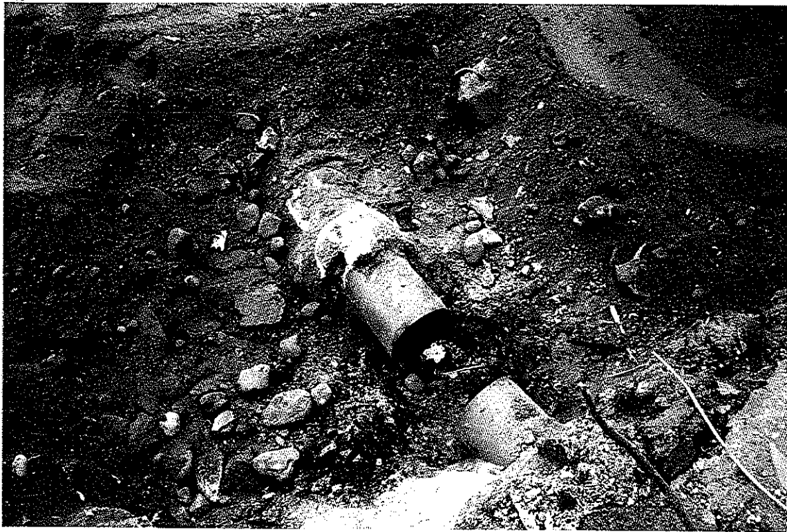
Repair To Drain Pipe
