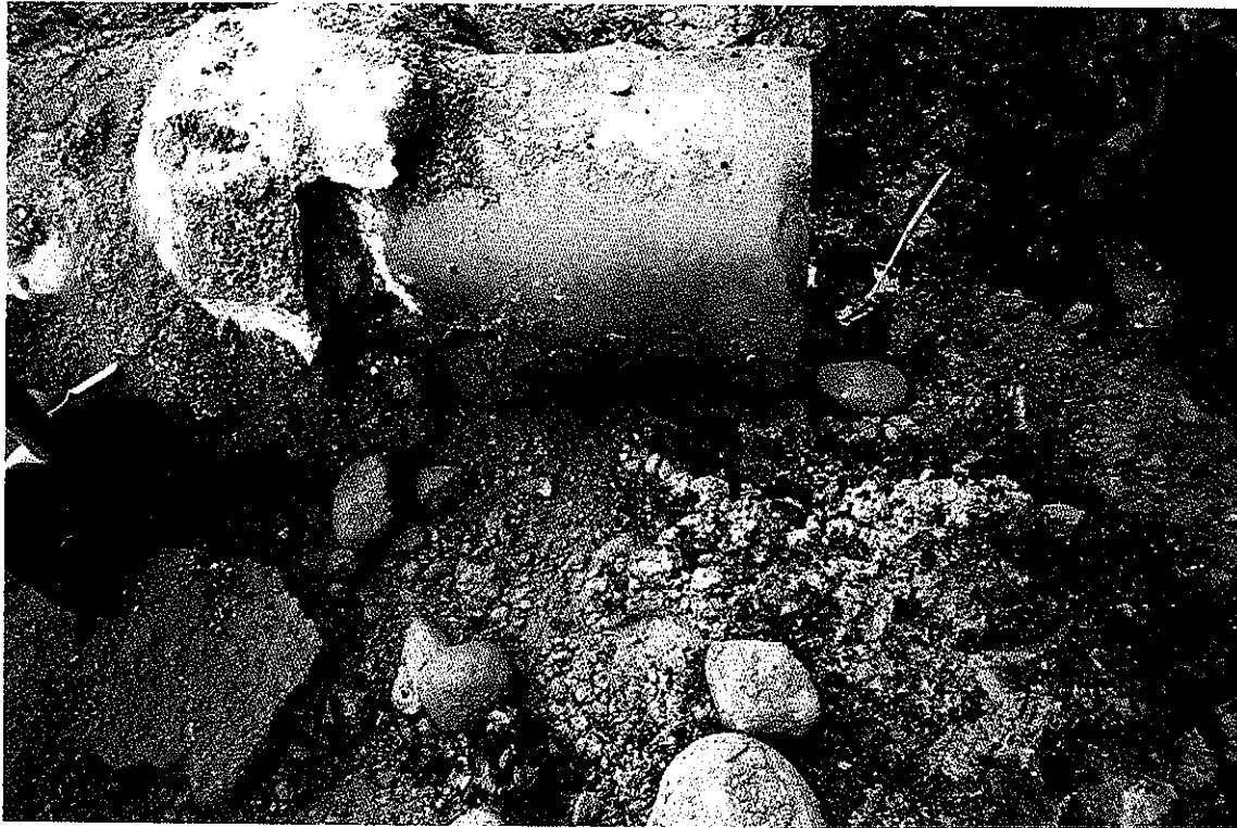
Repair To Drain Pipe
