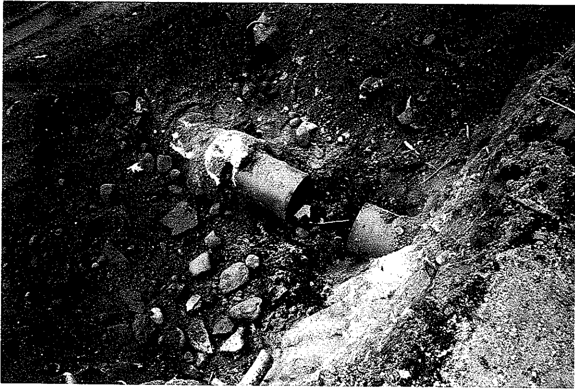
Repair To Drain Pipe
