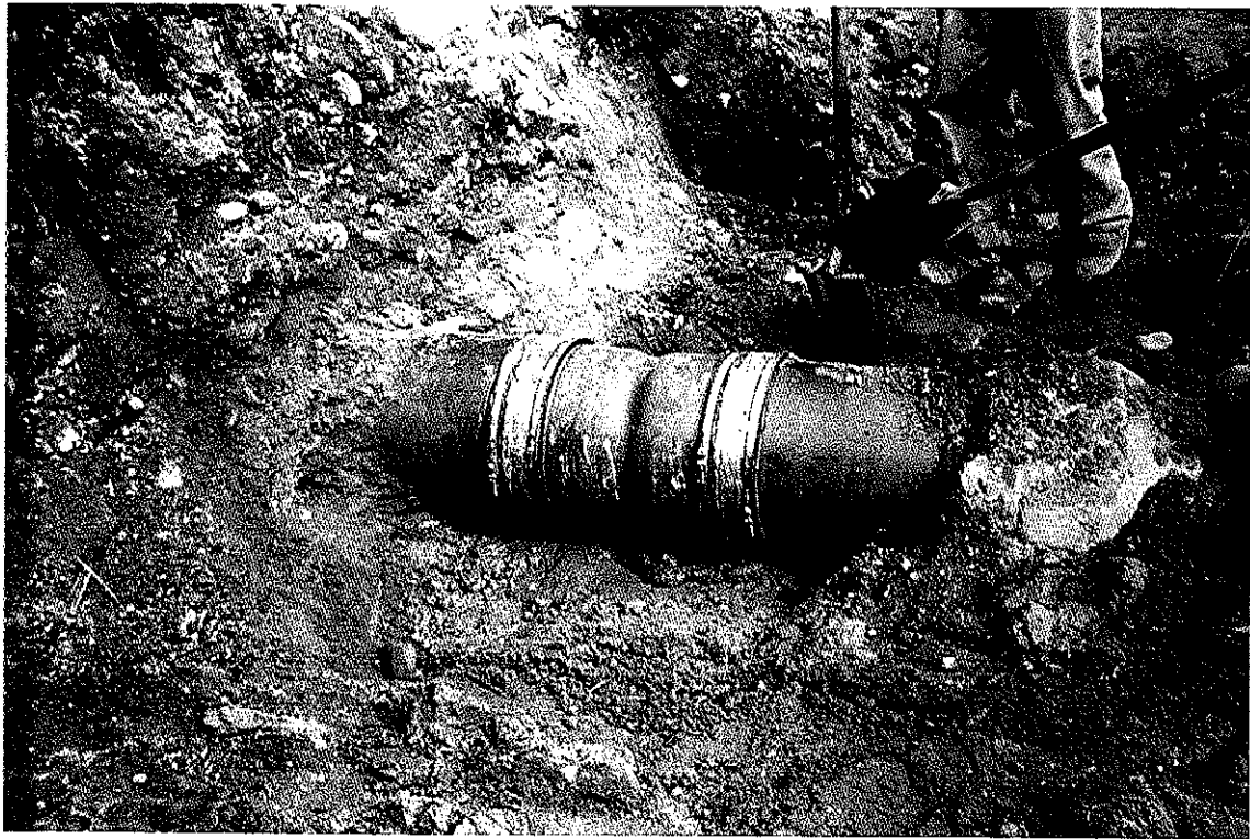
Repair To Drain Pipe
