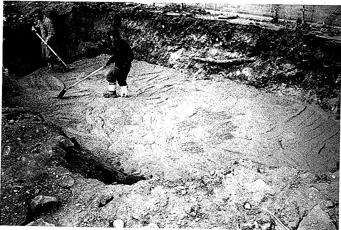
Working of Concrete Pad
