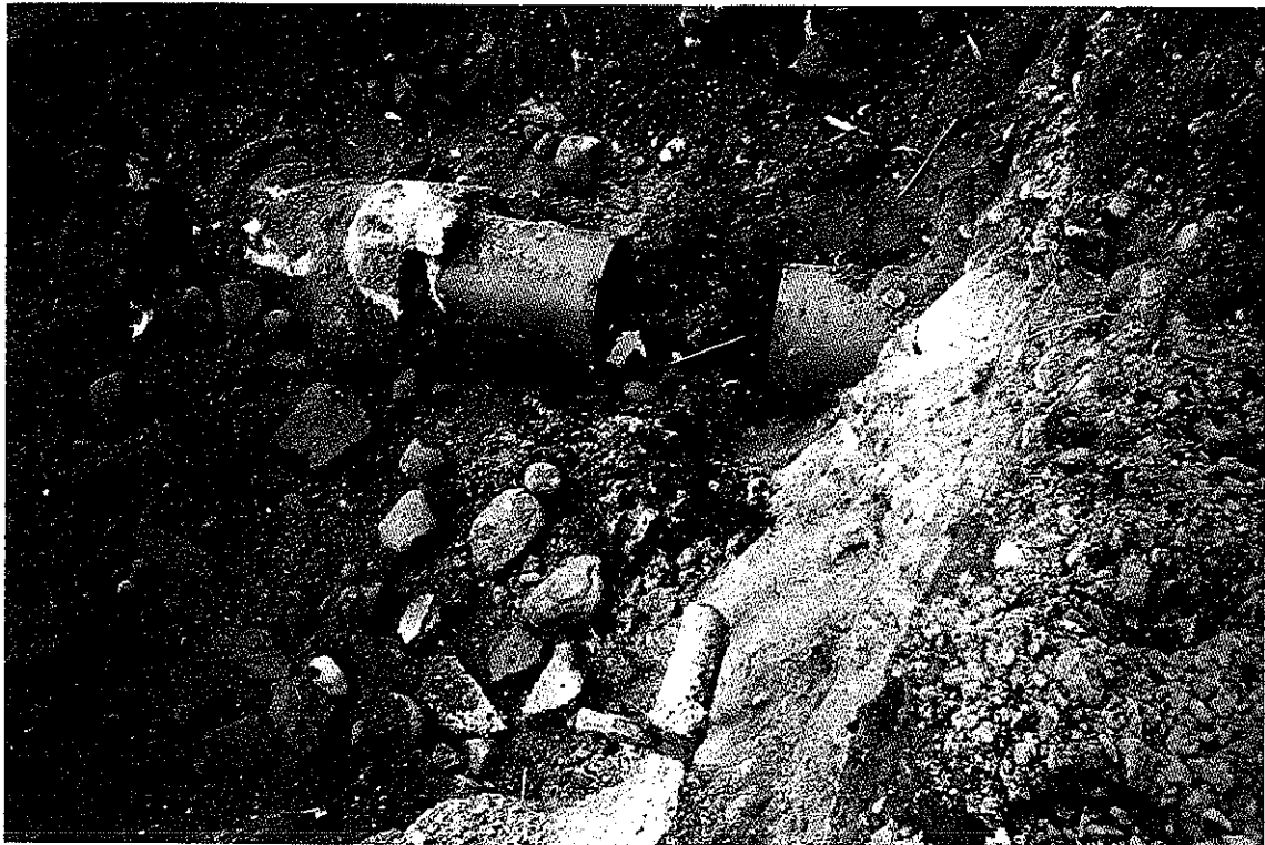
Repair To Drain Pipe
