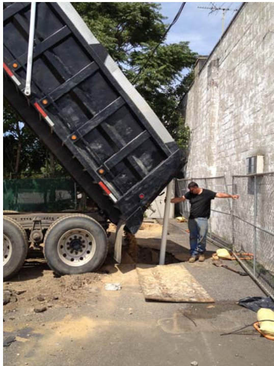
Photo 6 – Backfilling of Southern Cesspool (CP-S)
