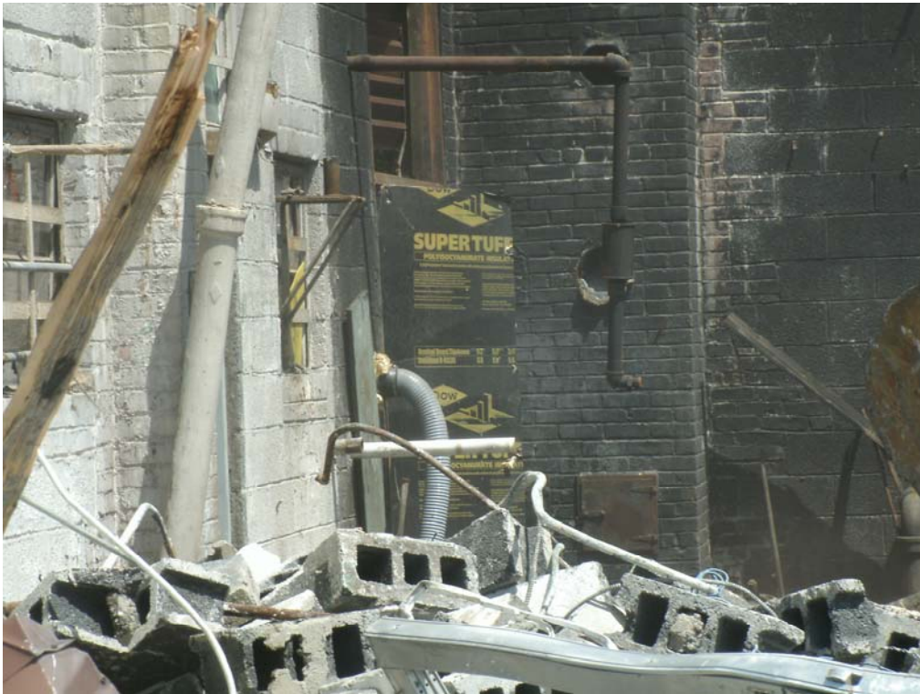
Photo 4 - Demolition waste from foundation removal (Post demolition)
