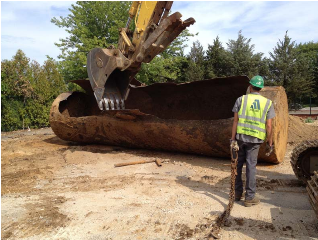
Photo 7 – Preparing tank for transportation to disposal facility
