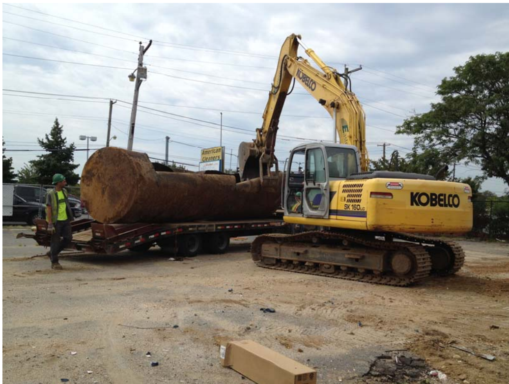
Photo 7 – Preparing tank for transportation to disposal facility
