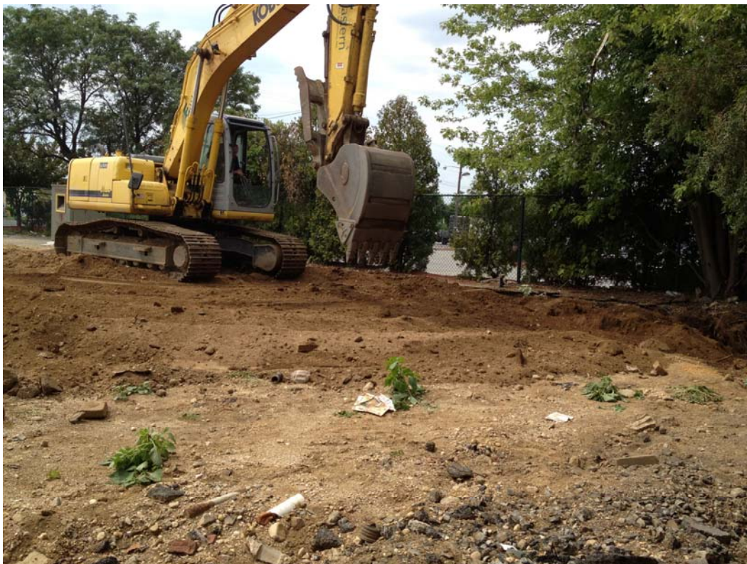
Photo 11 – Backfilling excavation
