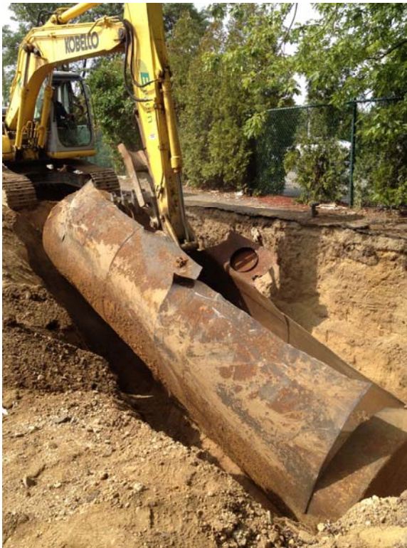
Photo 4 and 5 – Tank removal
