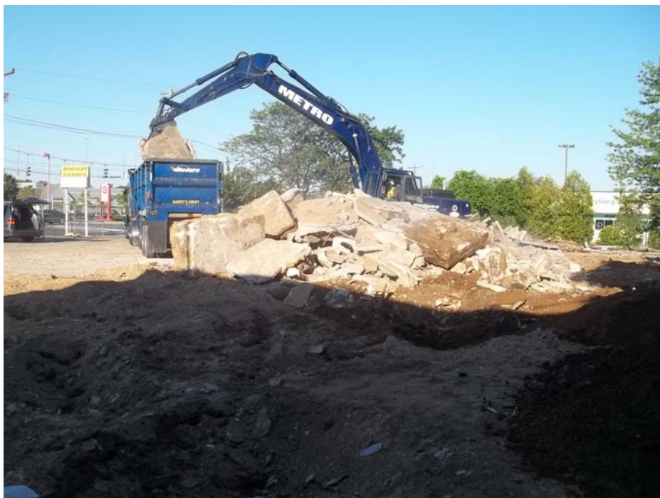
Picture 2 –Removal of concrete debris
