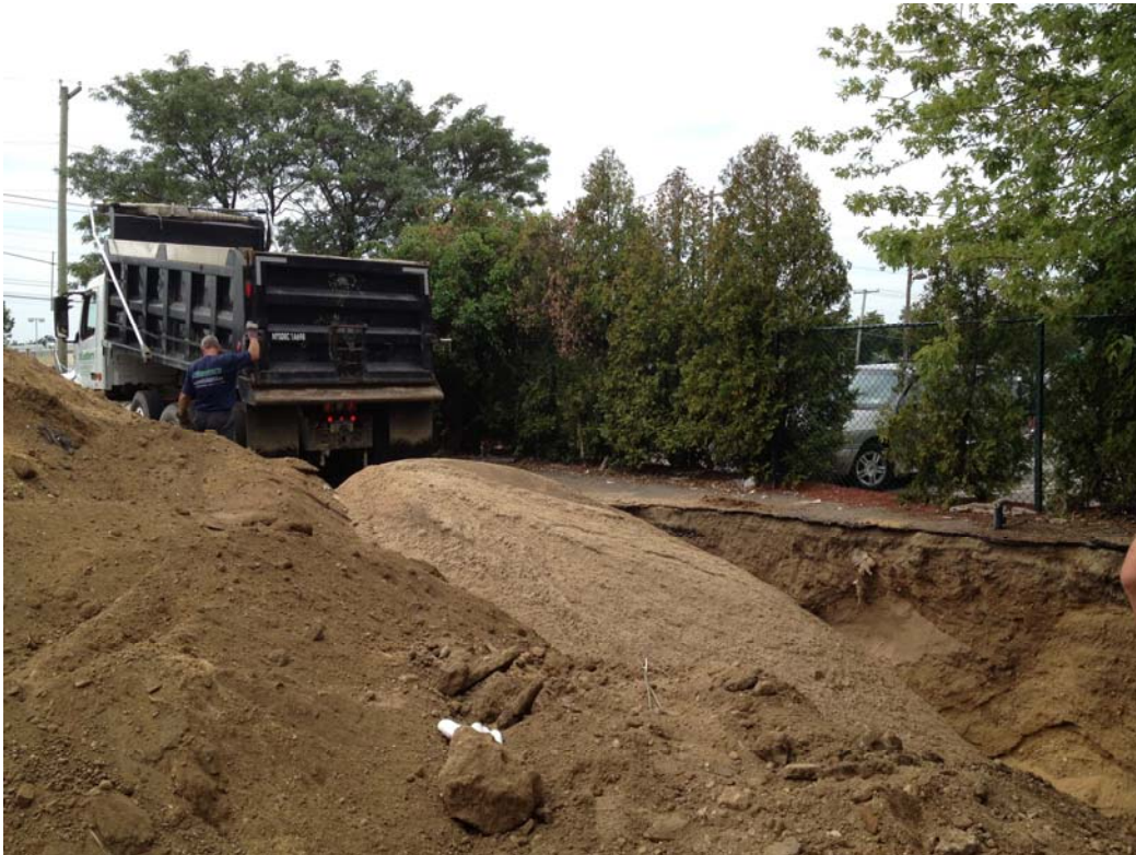
Photo 11 – Backfilling excavation
