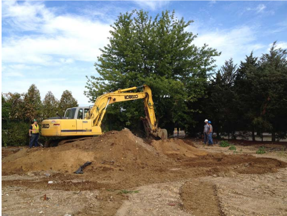
Picture 2 –Tank excavation
