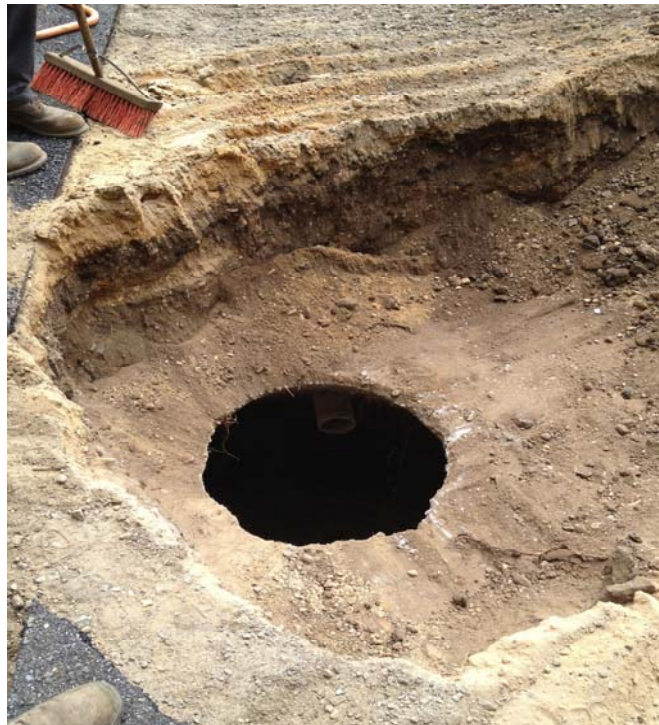
Picture 2 – Uncovering of Cesspools (August 20, 2012)
