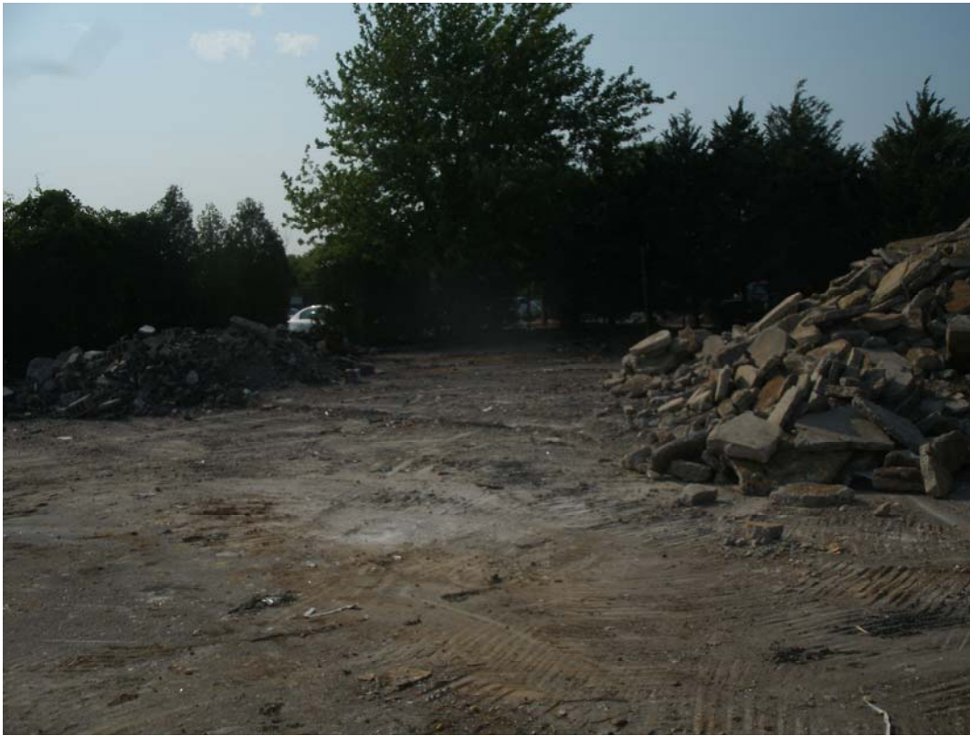
Photo 13 – Site post building demolition
