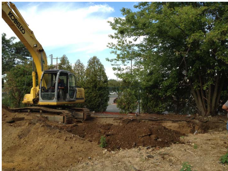
Picture 2 –Tank excavation
