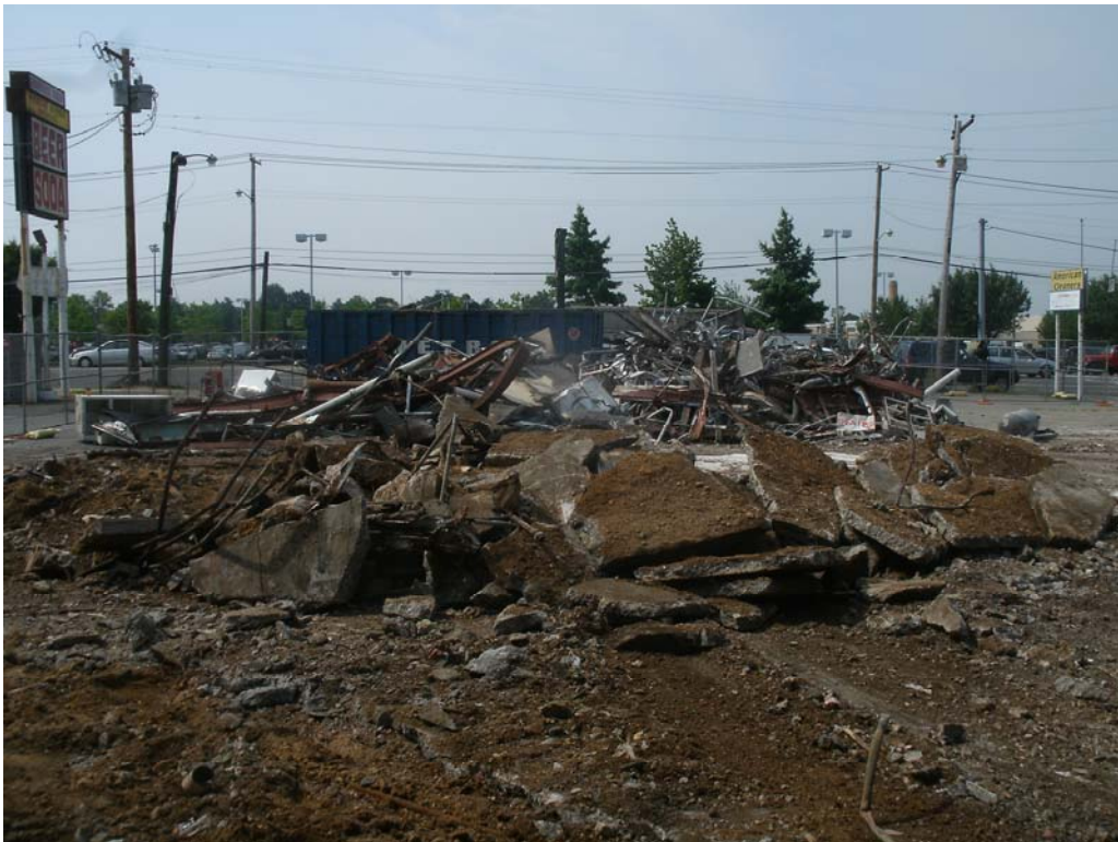
Photo 4 - Demolition waste from foundation removal (Post demolition)
