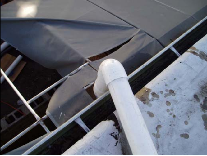
Site Name: Franklin Cleaners Site (on-site) Site No.: 1-30-050 Description of View: 4" PVC discharge piping installed on roof through awning. Date Taken: 01/11/07
