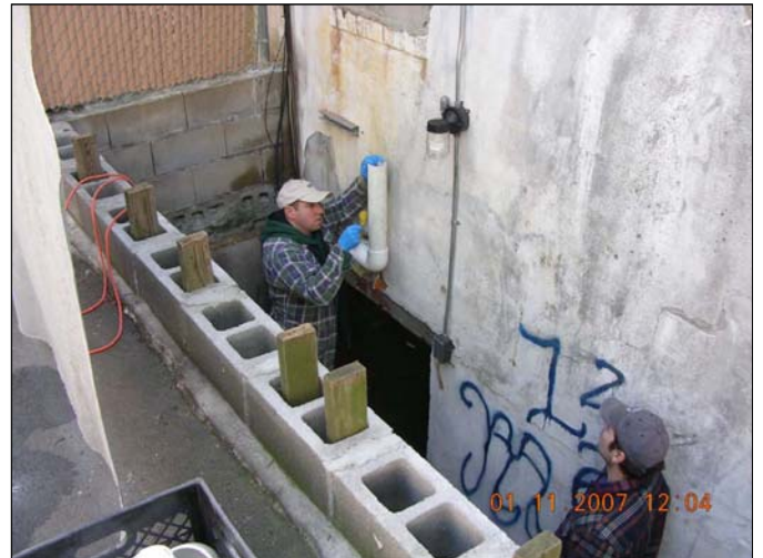
Site Name: Franklin Cleaners Site (on-site) Site No.: 1-30-050 Description of View: Installation of discharge piping on exterior rear wall.
