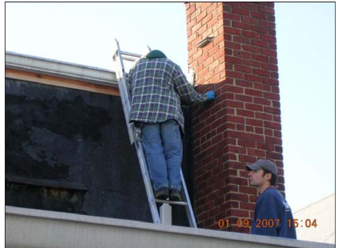
Site Name: Franklin Cleaners Site (on-site) Site No.: 1-30-050 Description of View: Installation of pipe supports on chimney for discharge piping. Photograph No.: 24
