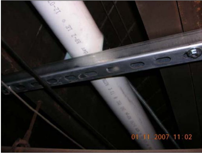
Site Name: Franklin Cleaners Site (on-site) Site No.: 1-30-050 Description of View: Pipe support for horizontal discharge pipe in floor joists (typical throughout basement).
