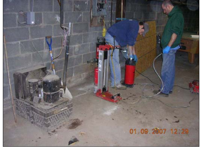
Site Name: Franklin Cleaners Site (on-site) Site No.: 1-30-050 Description of View: Installation of suction point SDP-4.
