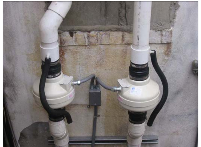
Site Name: Franklin Cleaners Site (on-site) Site No.: 1-30-050 Description of View: Fans installed on rear of building with condensate bypass. Date Taken: 03/01/07
