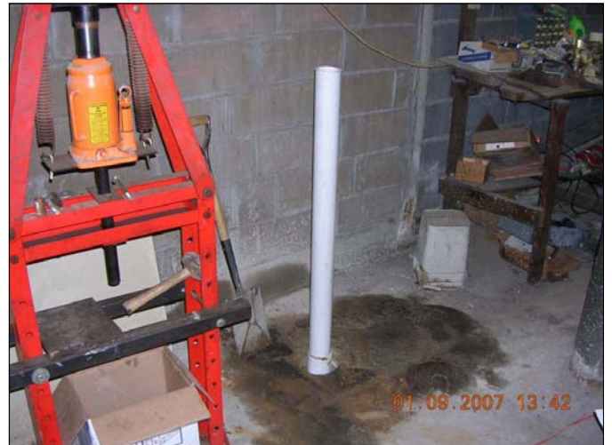
Site Name: Franklin Cleaners Site (on-site) Site No.: 1-30-050 Description of View: Suction point SDP-1 and associated piping.
