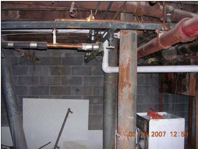
Site Name: Franklin Cleaners Site (on-site) Site No.: 1-30-050 Description of View: Discharge piping from SDP-2. Photograph No.: 31
