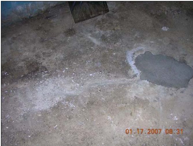
Site Name: Franklin Cleaners Site (on-site) Site No.: 1-30-050 Description of View: Patched concrete in deli basement. Photograph No.: 59
