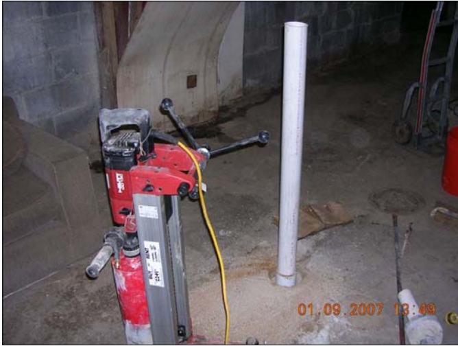
Site Name: Franklin Cleaners Site (on-site) Site No.: 1-30-050 Description of View: Suction point SDP-3 and associated piping. Photograph No.: 21
