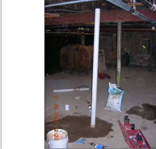
Site Name: Franklin Cleaners Site (on-site) Site No.: 1-30-050 Description of View: Suction point SDP-2 and associated suction point piping.
