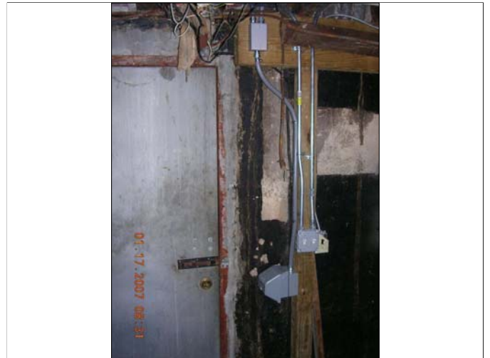
Site Name: Franklin Cleaners Site (on-site) Site No.: 1-30-050 Description of View: Electric disconnect switch for SSD fans installed near rear basement door. Photograph No.: 60
