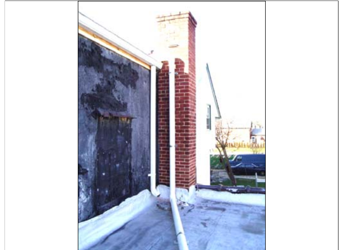
Site Name: Franklin Cleaners Site (on-site) Site No.: 1-30-050 Description of View: 4" PVC discharge piping installed on roof and along chimney. Date Taken: 01/11/07
