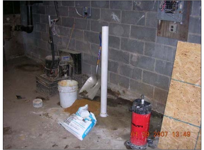
Site Name: Franklin Cleaners Site (on-site) Site No.: 1-30-050 Description of View: Suction point SDP-4 and associated piping. Photograph No.: 22
