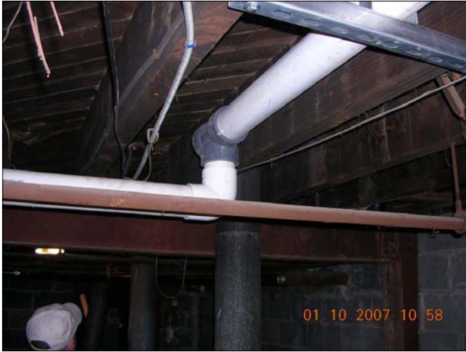
Site Name: Franklin Cleaners Site (on-site) Site No.: 1-30-050 Description of View: Discharge piping from SDP-1. Photograph No.: 29
