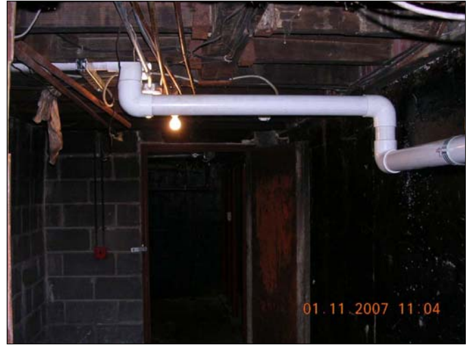
Site Name: Franklin Cleaners Site (on-site) Site No.: 1-30-050 Description of View: Discharge piping from SDP-1 and SDP-2 near rear of basement. Photograph No.: 46
