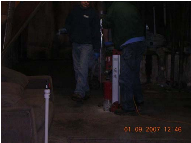
Site Name: Franklin Cleaners Site (on-site) Site No.: 1-30-050 Description of View: Installation of suction point SDP-3..
