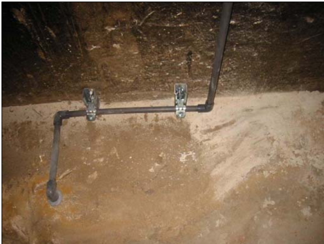
Site Name: Franklin Cleaners Site (on-site) Site No.: 1-30-050 Description of View: Condensate trap penetration through concrete floor. Date Taken: 03/01/07
