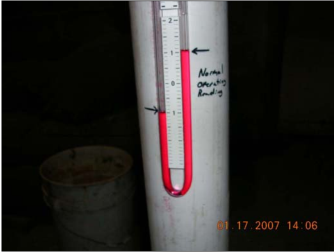
Site Name: Franklin Cleaners Site (on-site) Site No.: 1-30-050 Description of View: Manometer installed on suction point and starting vacuum label (typical for all suction points).
