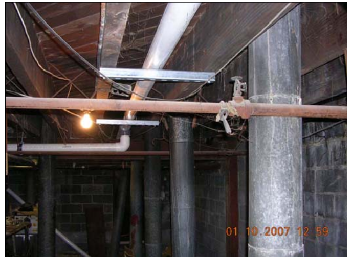
Site Name: Franklin Cleaners Site (on-site) Site No.: 1-30-050 Description of View: Discharge piping from SDP-2 and junction with discharge piping from SDP-1. Photograph No.: 32
