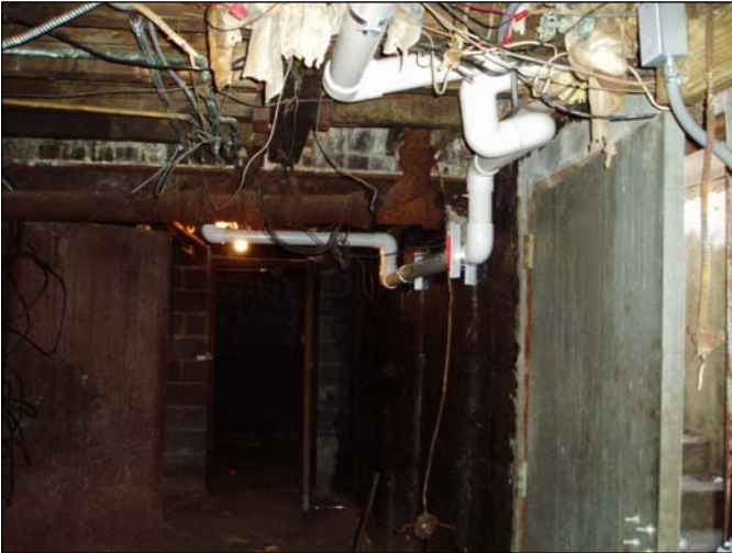
Site Name: Franklin Cleaners Site (on-site) Site No.: 1-30-050 Description of View: Discharge piping from SDP-3 and SDP-4 and manometer installed to monitor fan vacuum. Date Taken: 01/17/07
