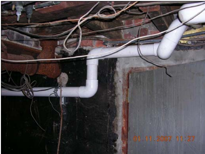
Site Name: Franklin Cleaners Site (on-site) Site No.: 1-30-050 Description of View: Discharge piping from SDP-1 and SDP-2 and penetration through rear basement wall.
