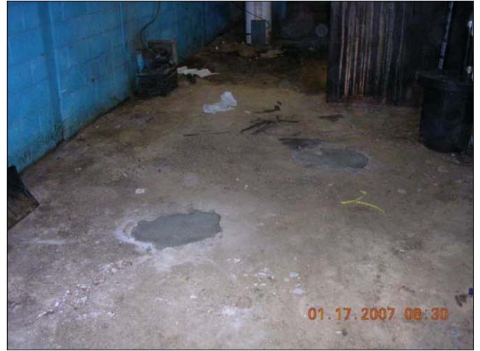
Site Name: Franklin Cleaners Site (on-site) Site No.: 1-30-050 Description of View: Patched concrete in deli basement. Photograph No.: 58
