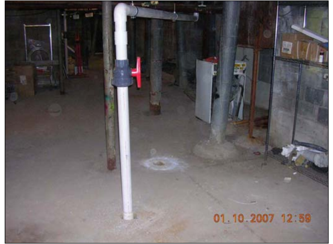
Site Name: Franklin Cleaners Site (on-site) Site No.: 1-30-050 Description of View: Suction point SDP-2 and associated piping. Photograph No.: 30
