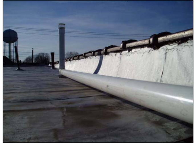
Site Name: Franklin Cleaners Site (on-site) Site No.: 1-30-050 Description of View: 4" PVC discharge piping installed on roof and effluent stack with rain cap. Date Taken: 01/11/07
