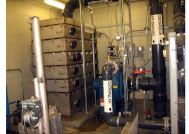
The GWE&TS was designed to recover and treat a chlorinated solvent groundwater contamination plume emanating from the Site and discharge the treated groundwater to a Nassau County Department of Public Works storm sewer manhole in accordance with all applicable discharge standards. Refer to [Figure 1-1](#) for a Site Location Map depicting the Site and associated GWE&TS location.
