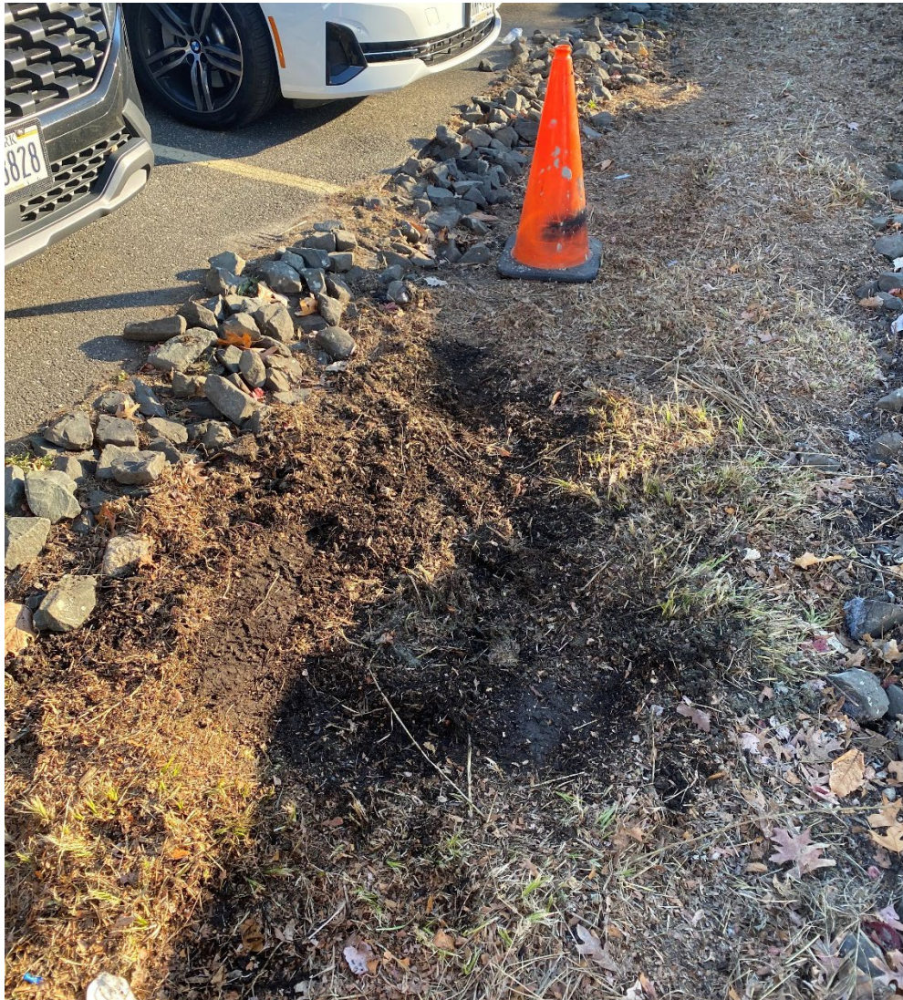
ASMW-6 following monitoring well abandonment
