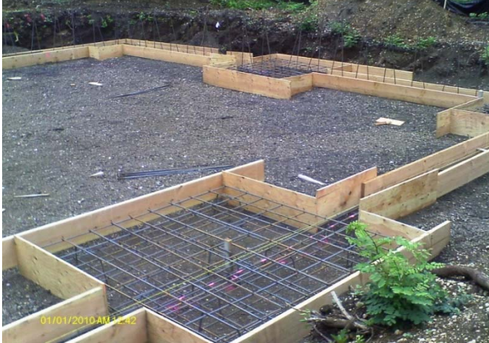
Photograph 3-10: View of treatment building footings facing northeast.
