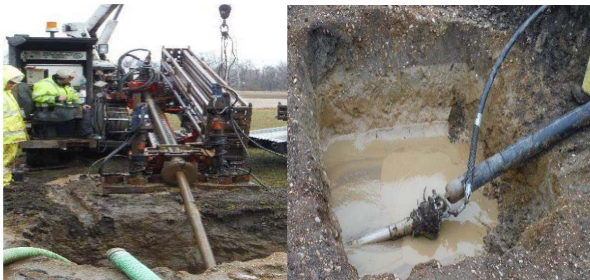
Photographs 3-19 and 3-20: HDD rig (left), and 2-inch and 6-inch HDPE pipe pulled by drill rig.
