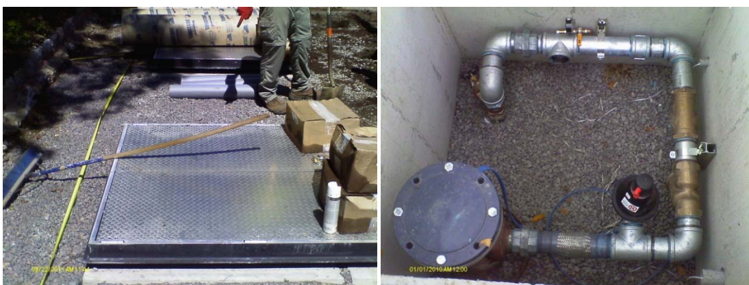
Photographs 3-12 and 3-13: Extraction well vault cover (left) and the typical piping inside the vault (right).
