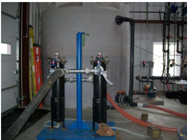
Photograph 3-18: Portable filter housing system.
