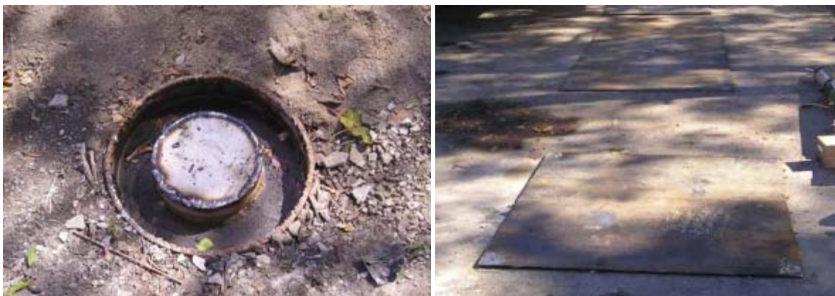
Photographs 3-5 and 3-6: Extraction well welded stainless steel cover (left) and steel plates (right).
