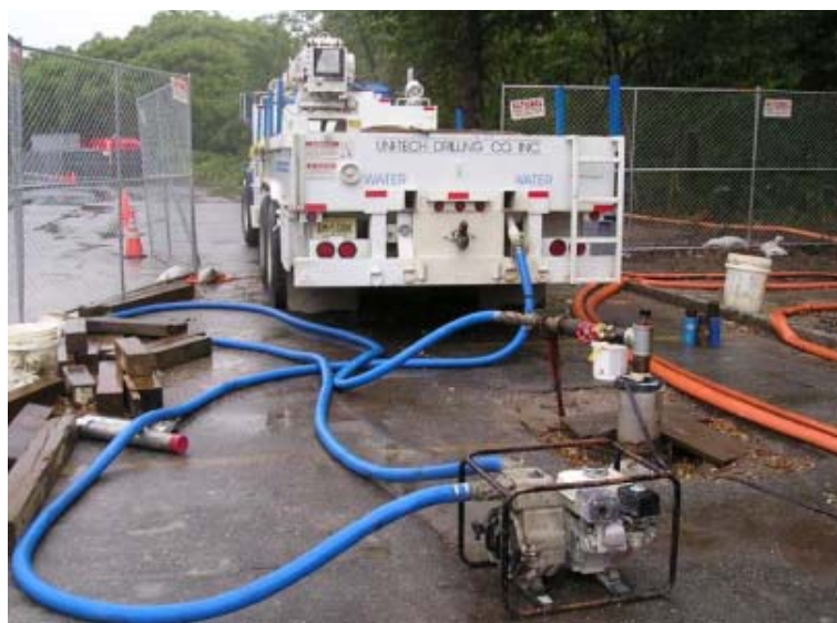
Photograph 3-7: Well disinfection setup.
