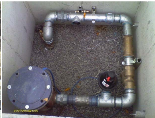
Photographs 3-12 and 3-13: Extraction well vault cover (left) and the typical piping inside the vault (right).
