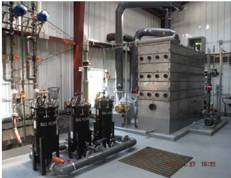
Photograph 3-23: Upgraded air stripper, bag filter housing, and duct pipe.
