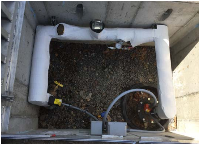
Photograph 3-22: Southern extraction well vault.
