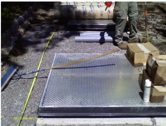
Photographs 3-12 and 3-13: Extraction well vault cover (left) and the typical piping inside the vault (right).
