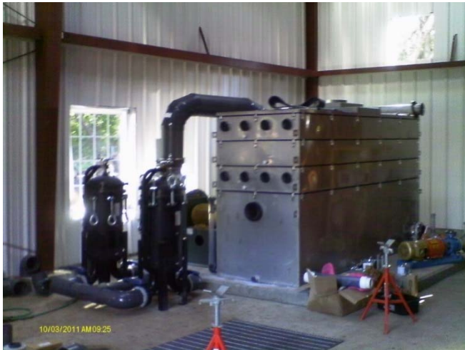
Photograph 3-14: Bag filter housing and air stripper in place, facing northeast.
