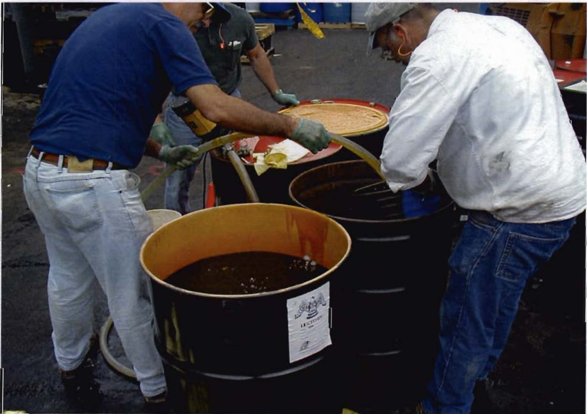
Preparation of soybean oil/lecithin emulsion for injection at Bioremediation Pilot Study location (31 Sea Cliff Ave).
