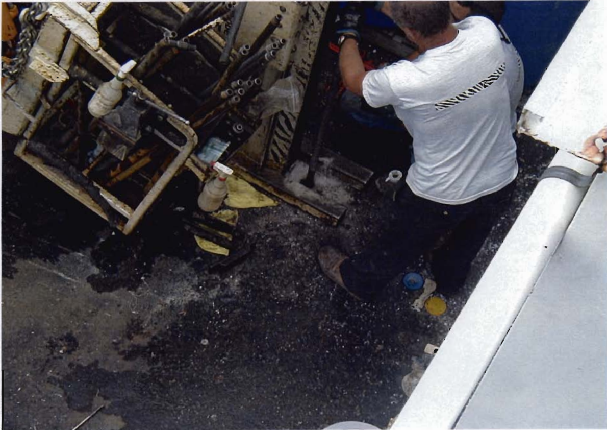
Injection of soybean oil/lecithin emulsion into a borehole.
