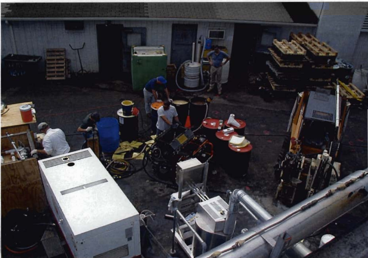
Charging of injection pump with emulsion. Note the stainless steel crossover exhaust between Catalytic Oxidizer and acid scrubber in lower right corner. The corrosion caused by the acidic exhaust stream resulted in the replacement of this section of exhaust with PVC pipe (as discussed in Section 2.1 of this report).
