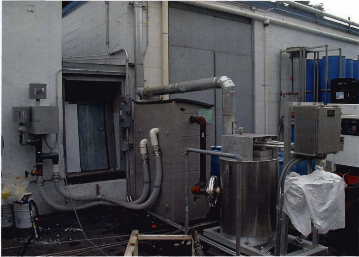
Soil Vapor Extraction System and associated Catalytic Oxidizer installed at 31 Sea Cliff Avenue site.
