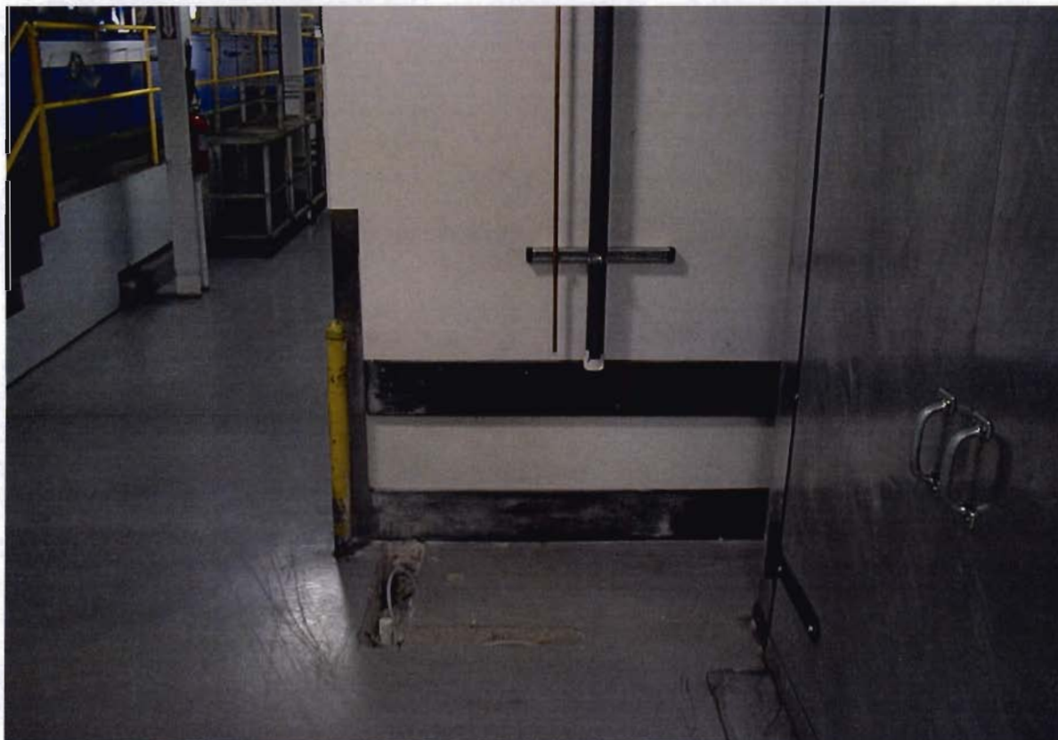
Installation of SVE/AS-4 inside Building 7 at 45 Sea Cliff Avenue site. Note the channel cut that was required through the production floor. The PVC SVE well riser is evident within the channel cut. The polyethylene tubing inside the channel cut connects to the air sparge point. A vehicle-mounted Geoprobe unit (Mule) had to be pushed by hand through the narrow aisle to access this location.
