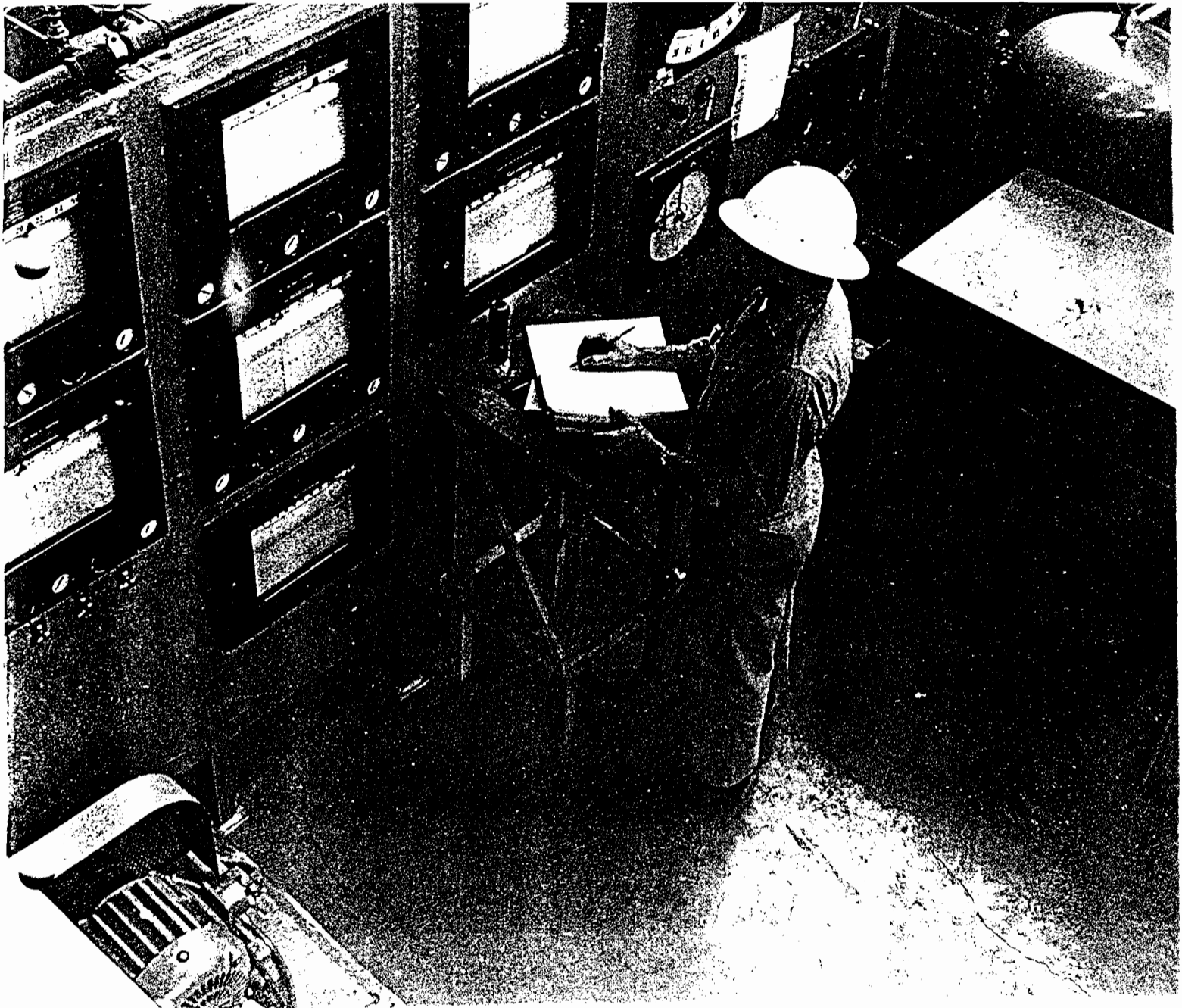
Instrument control panel for automated operation of Fibrous Glass plant. Sand, borax and other raw materials are put in at one end of the assembly line. Finished material or products ready for packaging come out the other end.
