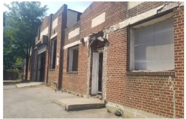
Area of building where abatement of asbestos materials is complete.
