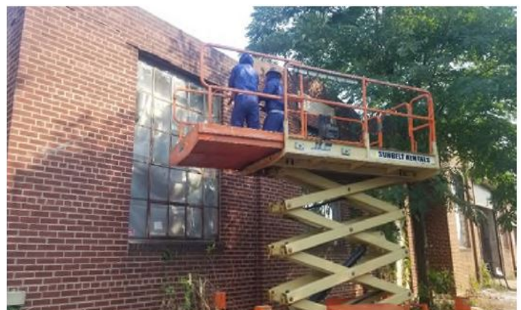
Active abatement of asbestos material.
