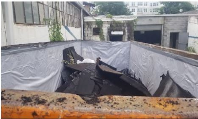
Abated asbestos materials placed in poly-lined container for proper removal from the site.
