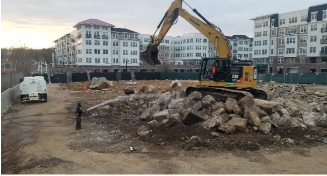
Breaking up concrete from former building floor slab and foundation. Materials were removed from the site and recycled into aggregate
