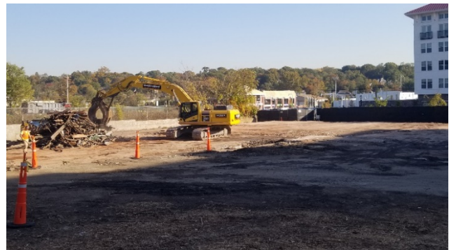
Former site building demolished and debris being removed from site.
