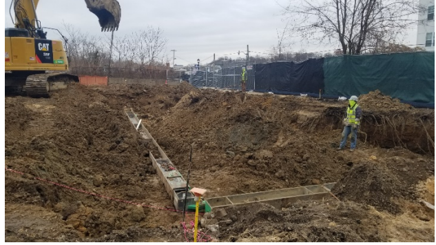
Installing sheeting at the start of source area soil excavation.
