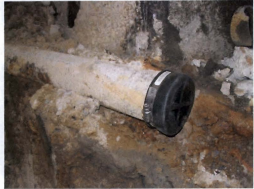
Photo 14: Cap of Former Drain Pipe
