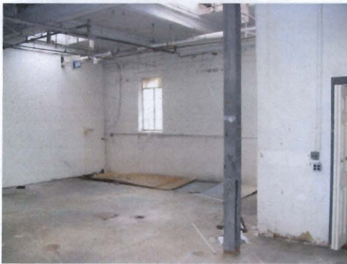
Photo 3: Dividing and West Walls, view SW
