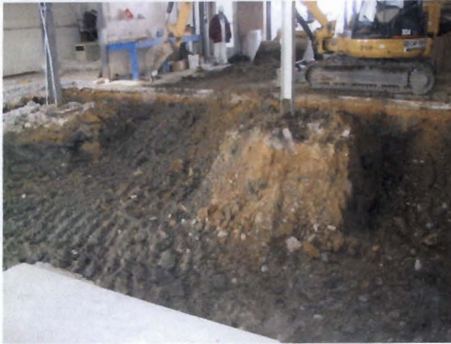
Photo 13: North End of Excavation
