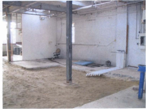
Photo 26: Compacted Sand w/ Stubs
