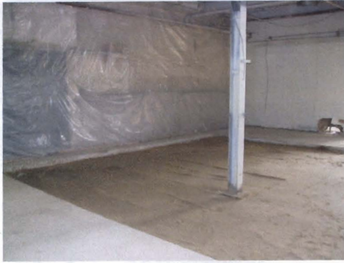
Photo 25: Compacted Sand
