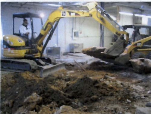
Photo 11: Progressive Removal of Concrete
