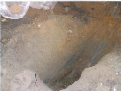
Photo 17: Typical Pit into Groundwater in Hotspots
