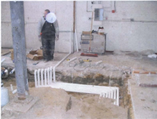
Photo 21: West Wall with Piping
