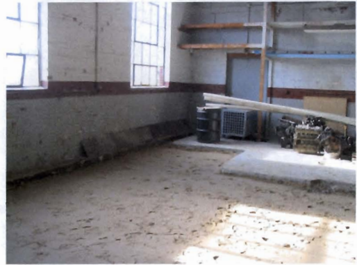
Photo 28: Compacted Sand, view SW
