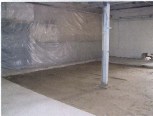
Photo 27: Compacted Sand, view SE
