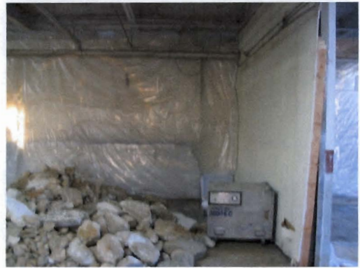
Photo 9, 10: Sealed Partition and Opened Dividing Wall
