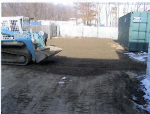
Photo 33: Driveway Restoration, view N
