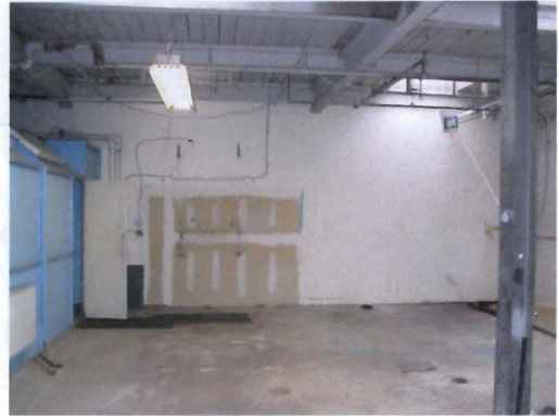
Photo 2: Dividing Wall to be Opened, view S
