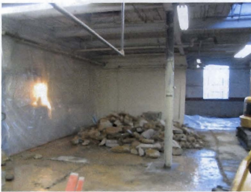
Photo 9, 10: Sealed Partition and Opened Dividing Wall
