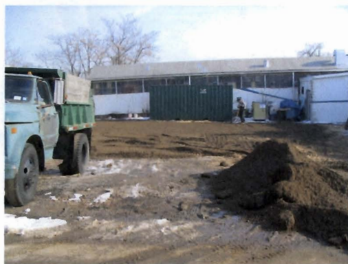
Photo 34: Driveway Restoration, view E
