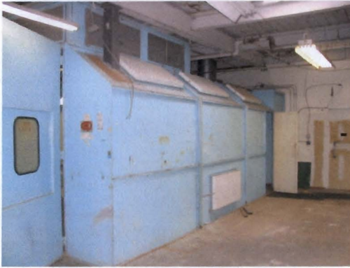
Photo 1: Spraybooth, view SE
