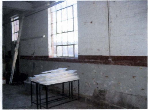
Photo 8: South Wall with Ditch
