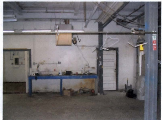
Photo 4: West Wall, Laundry
