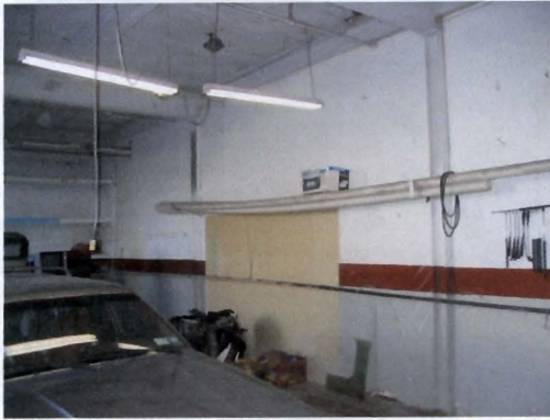
Photo 7: Dividing Wall to be Opened, view NW
