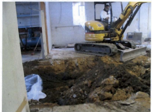
Photo 12: Progressive Removal of Soil
