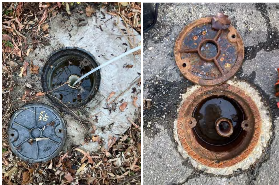
MW-7D (left) and MW-4R
