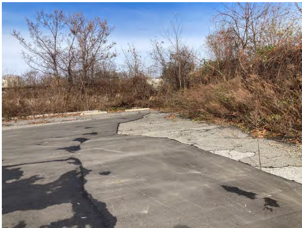
NE Corner of Site
