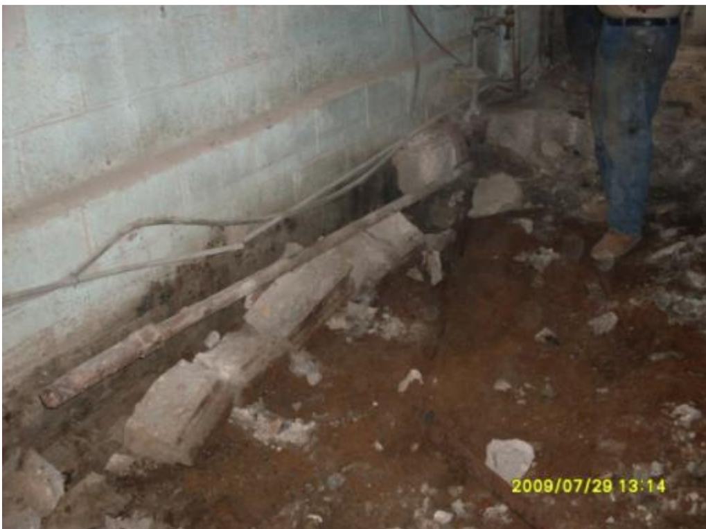
Below Grade Piping Discovered while Demolishing Machine Room floor (July 2009)
