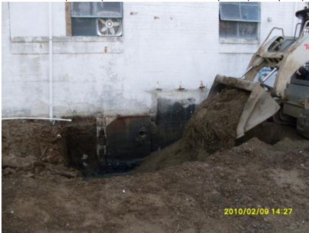
Backfilling oil-water separator excavation (February 2010)
