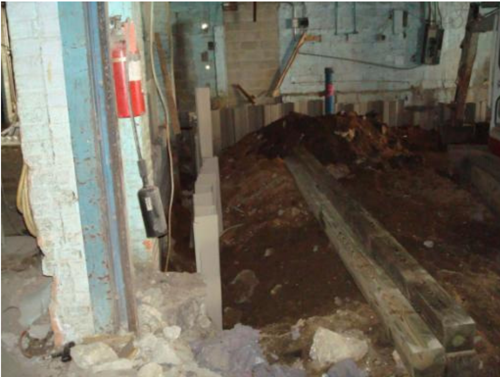
Shoring installed around Load Bearing Walls in Machine Room (September 2009)
