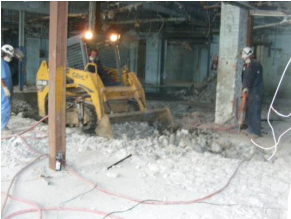
Removing the Top Layer of Concrete in the Machine Room (July 2009)
