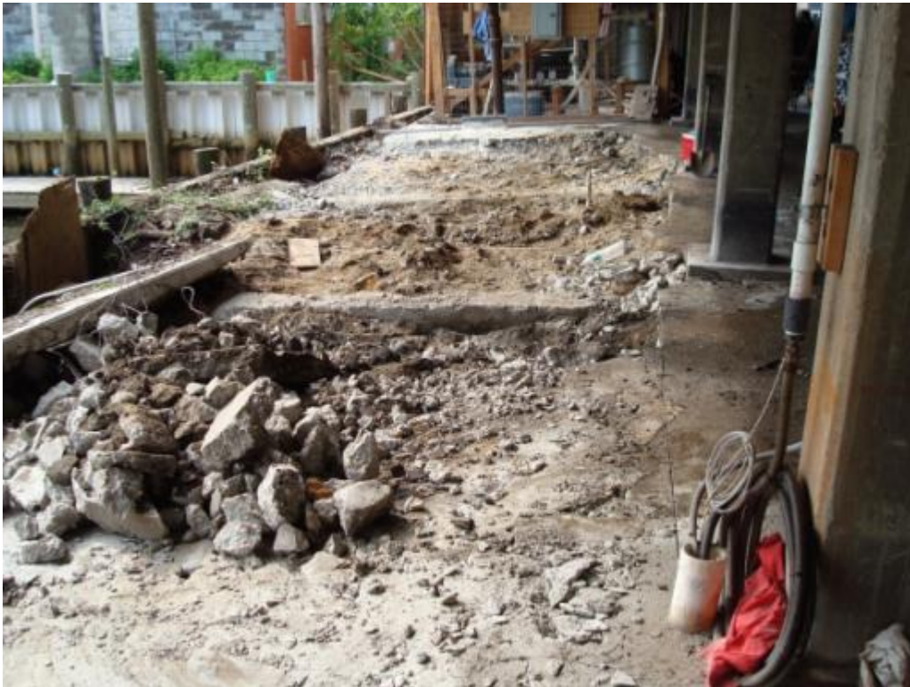
Initial breakup of concrete floor adjacent to old bulkheading (June 2009)
