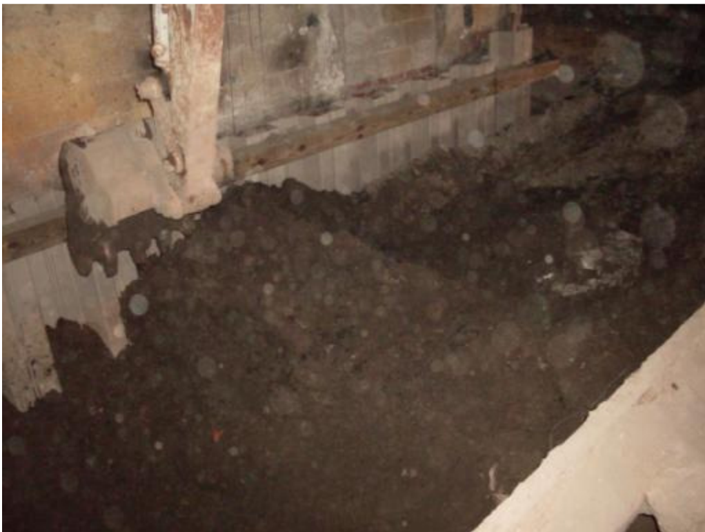
Shoring along the Compressor Room Wall during Excavation (October 2009)
