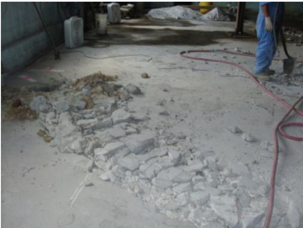
Broken concrete in the machine room to chase pipes connected to oil-water separator (July 2009)
