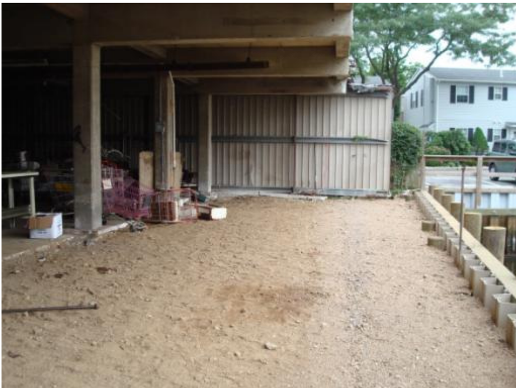
Replaced bulkhead and backfilled ground surface (June 2009)
