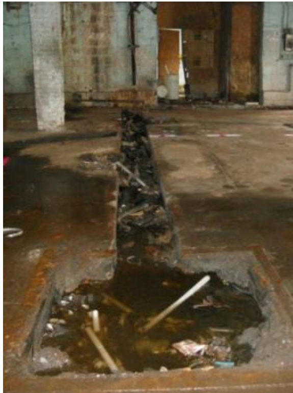
Floor Drain in Machine Room Pre-Demolition (June 2009)
