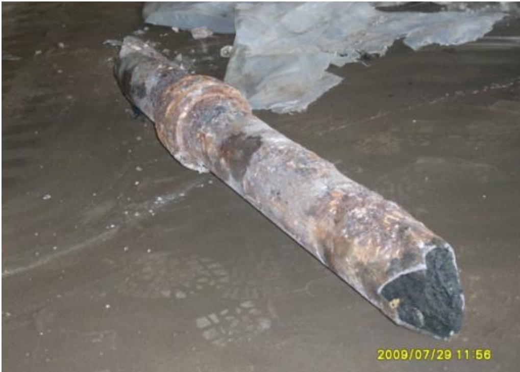
Removal of a former pipe from the machine room floor connected to the oil-water separator (July 2009)
