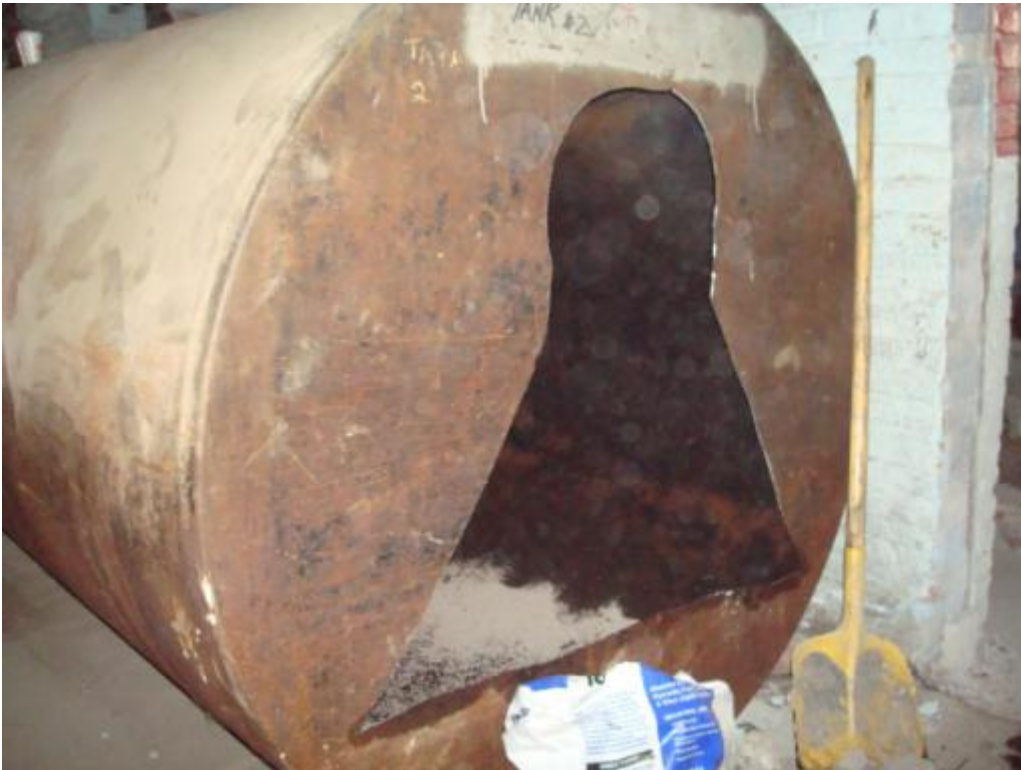
One 2,000 gallon tank following removal and cleanout (October 2009)
