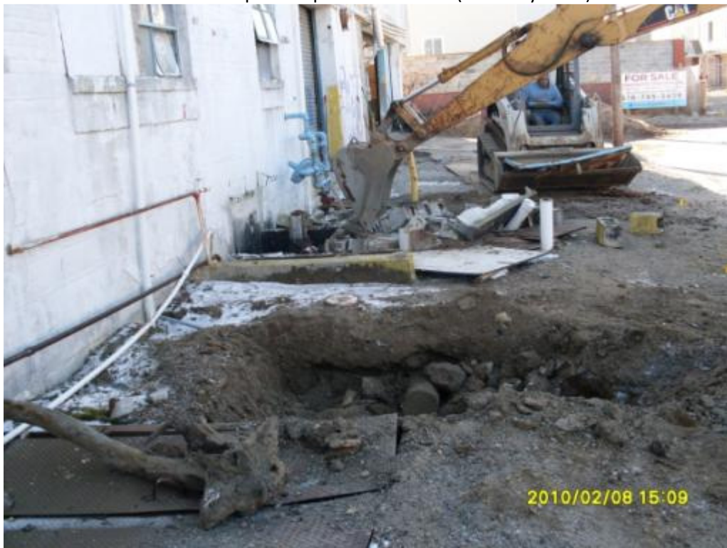
Destruction of the oil-water separator (February 2010)
