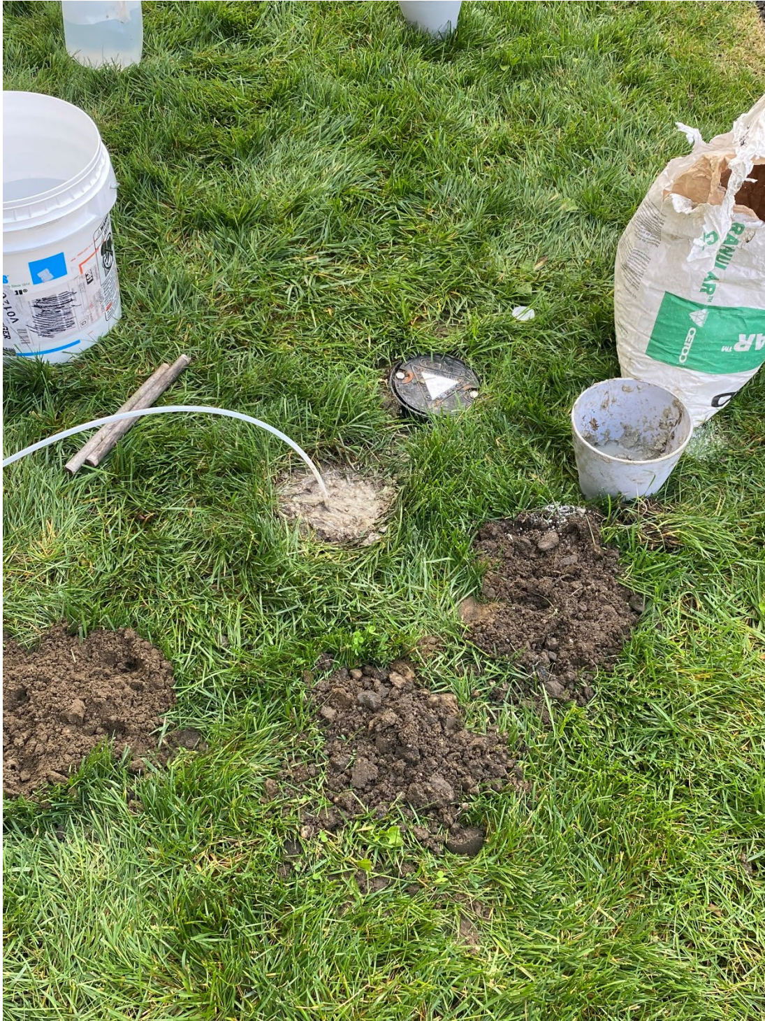
Figure 2: Finished temporary soil vapor point near VMP-5.
