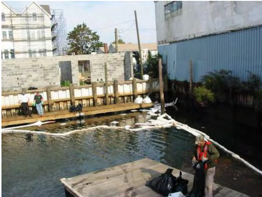
October 23, 2007- Absorbent socks set up as a levee along the canal to prevent fuel oil impacts (southwest side of building)
