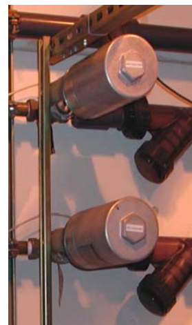
Figure 13.4 Jordan Control Valves and Sediment Strainers
