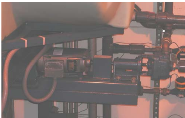
Figure 21.2 Holding Tank Transfer Pump
