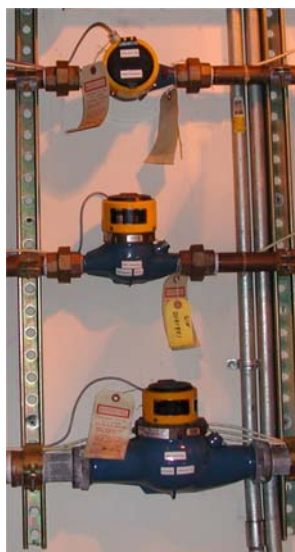
Figure 14.4 Niagara Series MTX Recovery Well Flow Meters
