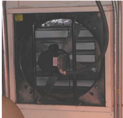
Figure 23.1 Treatment Room Exhaust Fan
