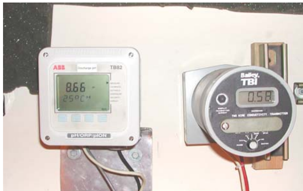
Figure 18.5 Discharge pH and Conductivity Transmitter
