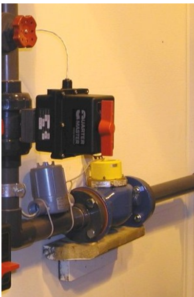
Figure 19.1 Discharge Valve and Water Flow Meter
