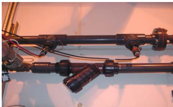
Figure 15.5 pH and Conductivity Meters Installed in Influent Water Line
