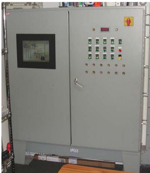
Figure 22.1 Treatment System Control Panel - Exterior
