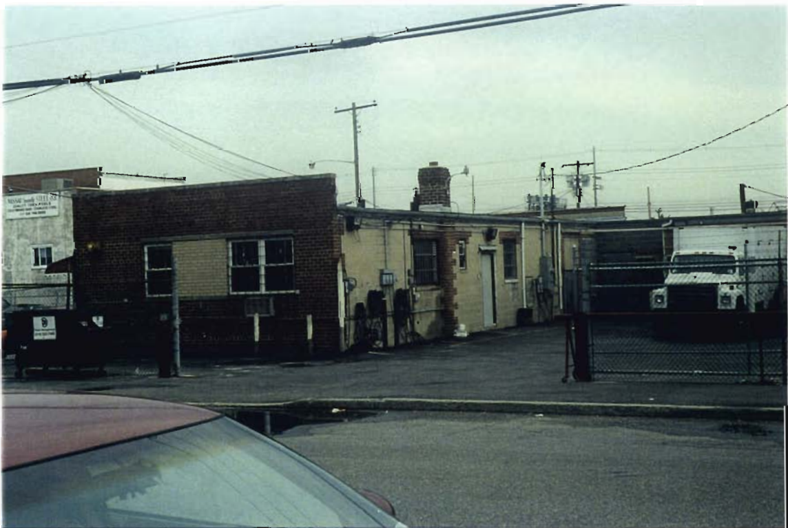
SKS Industries building, looking south from Broadway
