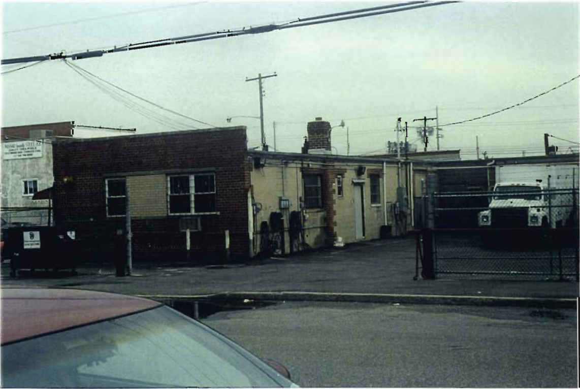
SKS Industries building, looking south from Broadway
