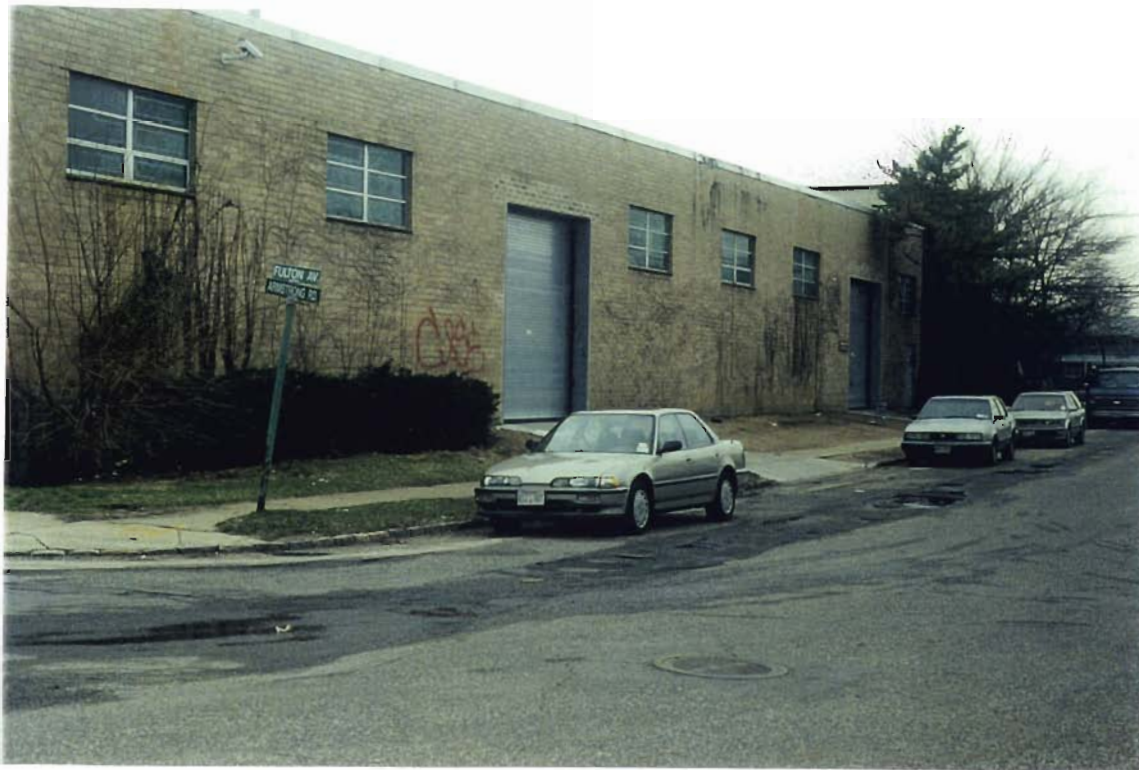
East side of building, looking northwest from Armstrong Road
