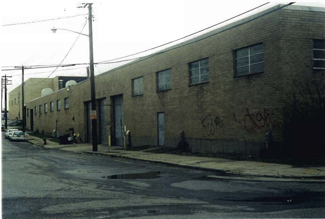
Rear (south side) of building from Armstrong Road looking west
