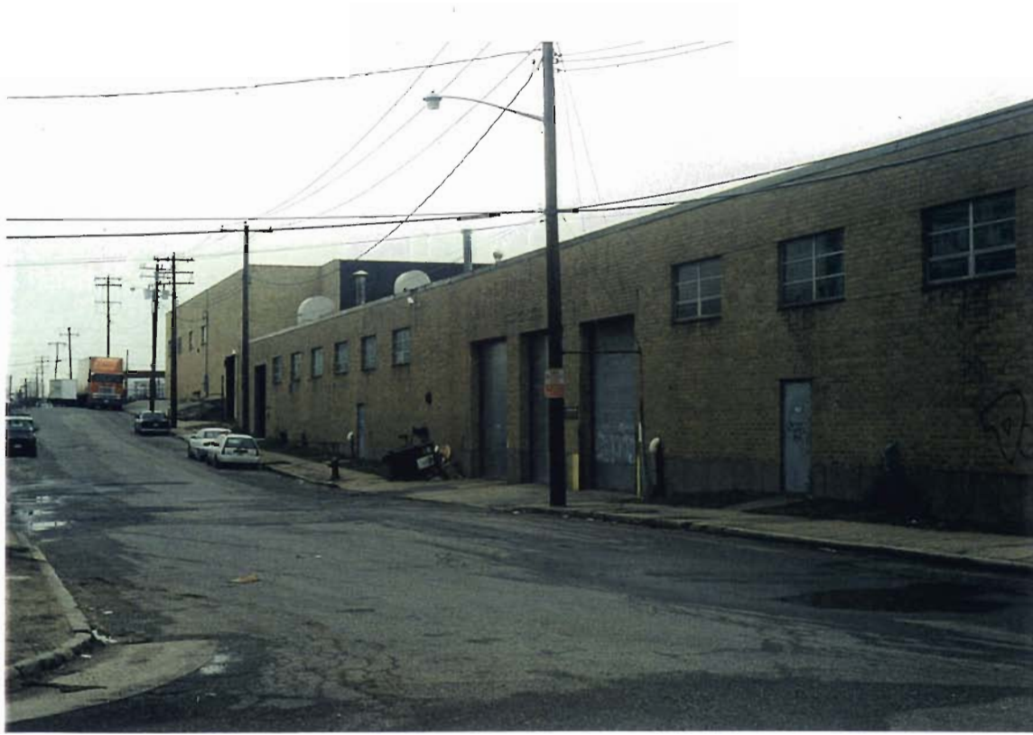
Rear (south side) of building from Armstrong Road looking west
