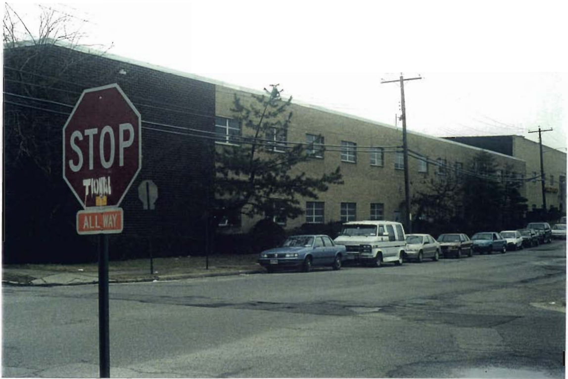
View of front of building, from Broadway looking southwest
