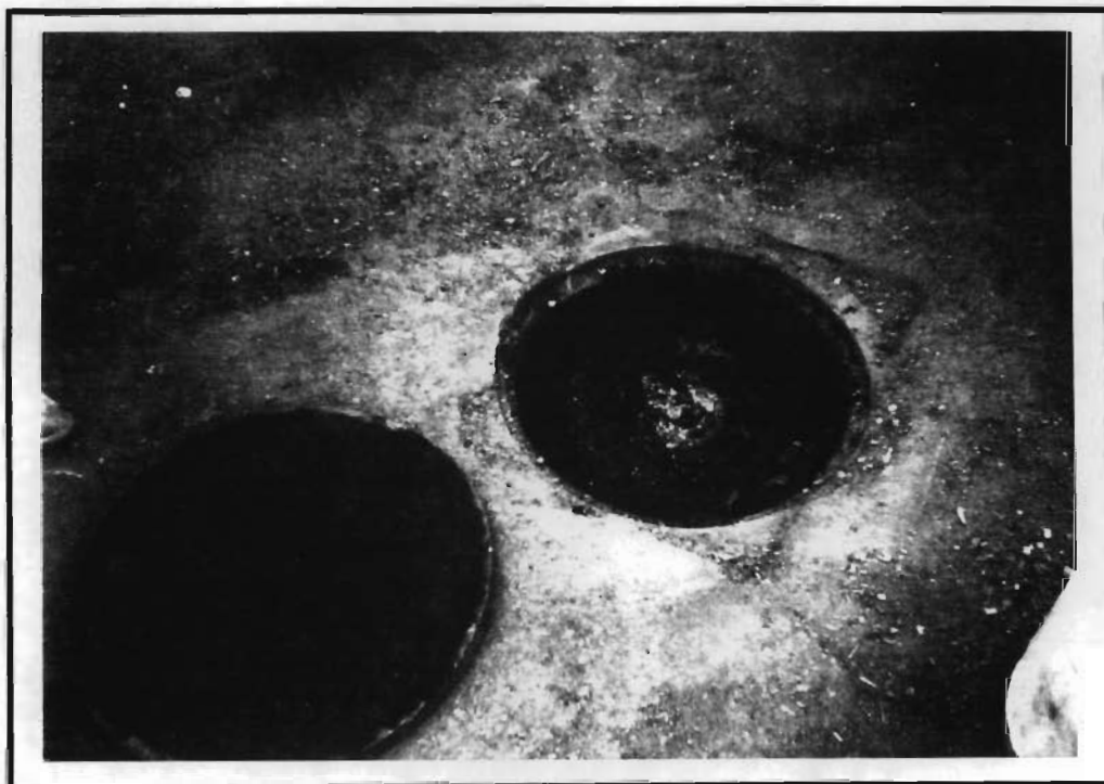
Photograph No. 4 -Dry well, DW-1, lid opened, rust-colored sand and gravel visible inside. (November 14, 1995).
