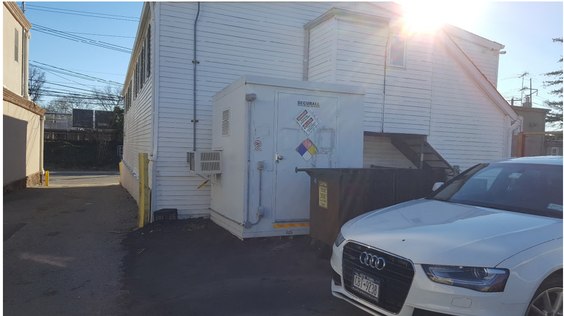
Photograph #3 – View looking south along east side of the office/garage building. Secure storage locker for pesticides located at north end of the building.
