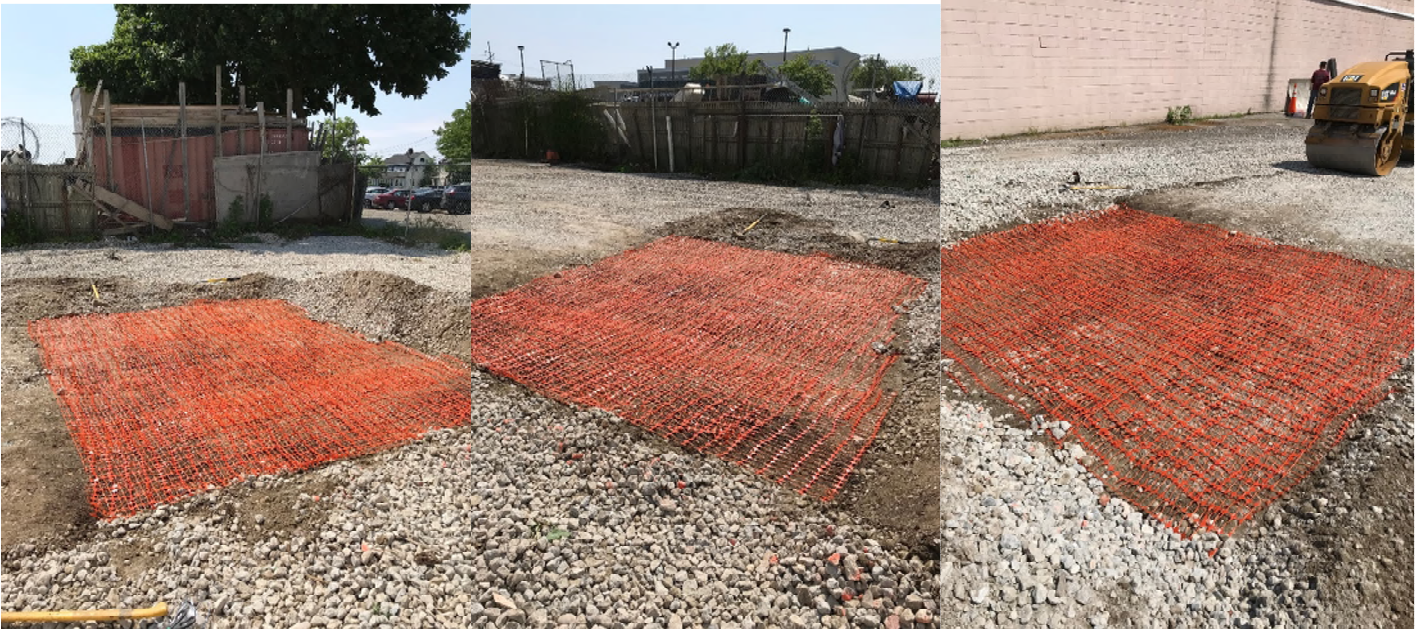
Installation of Demarcation Netting over Area SB-7
