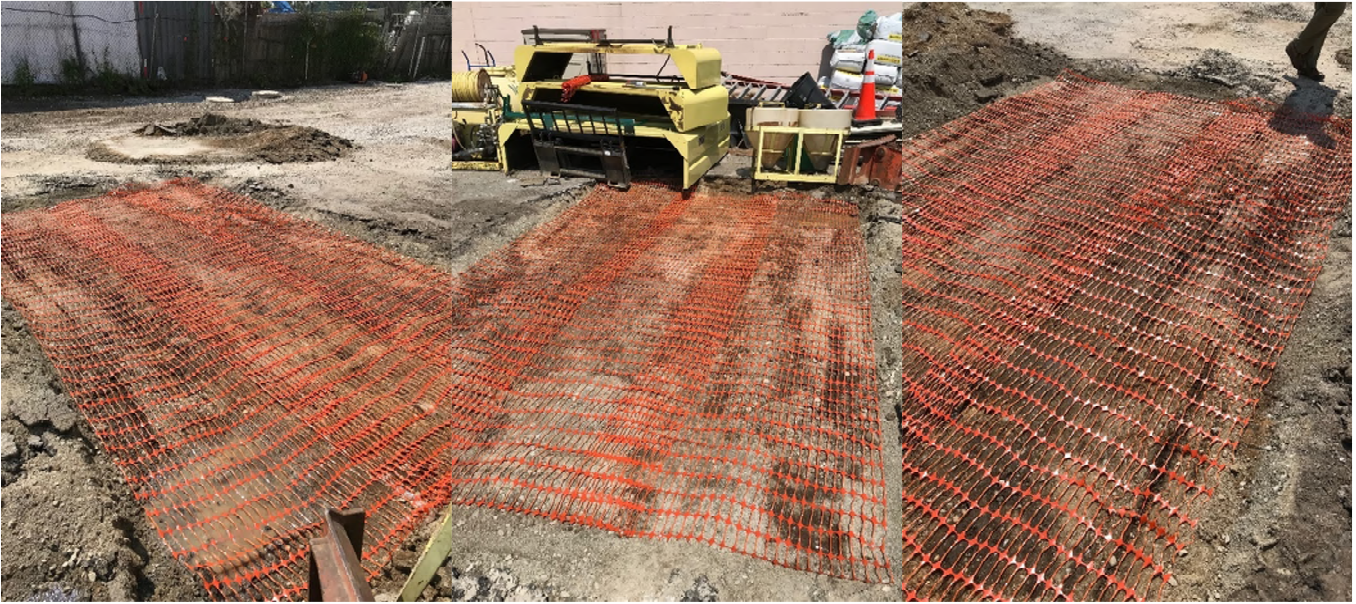
Installation of Demarcation Netting over Area SB-6
