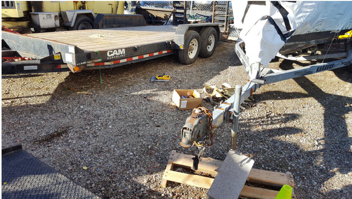
Photograph #11 – Area of remaining subsurface soil contamination in vicinity of boring SB-7 (at metal notebook and yellow tape measure). Original ground surface covered by aggregate.
