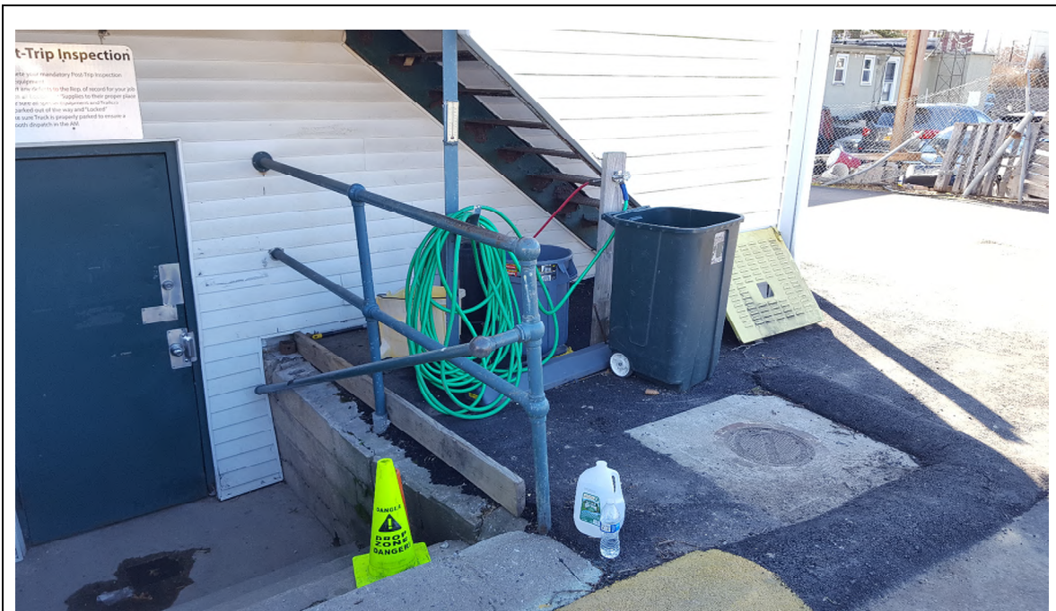
Photograph #13 – Area of remaining subsurface soil contamination, vicinity of former test pit TP-2, under wheeled trash receptacle. Area is covered by asphalt paving.
