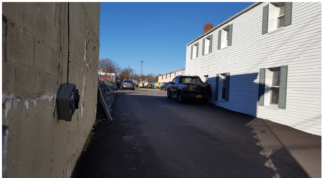
Photograph #2 – View looking north along west side of the office/garage building.
