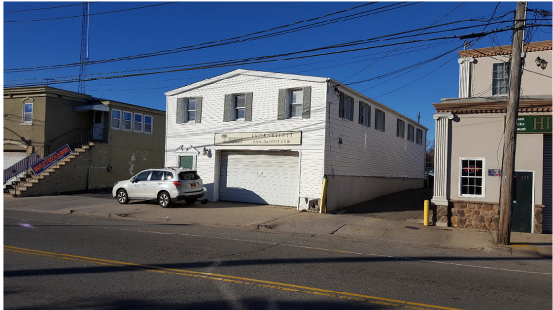
Photograph #1 – Bartlett Tree Experts office/garage building, viewed looking north from Union Avenue.
