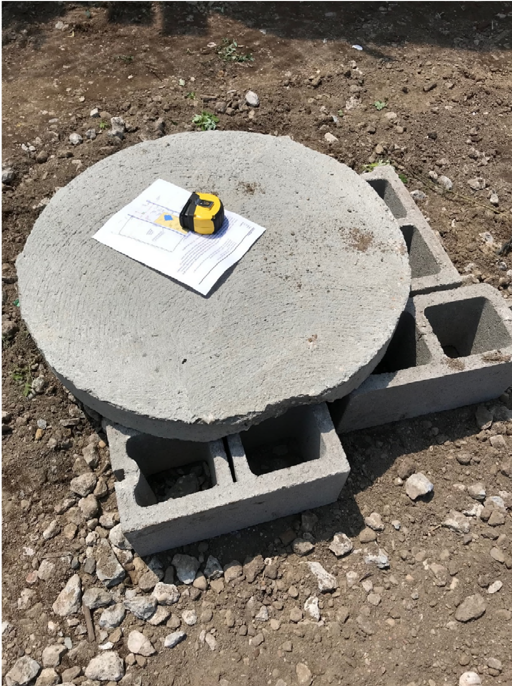
Typical Installation for Monitoring Well Protection
