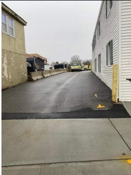
Photograph #2 – View looking north from Union Avenue along west side of the office/garage building.
