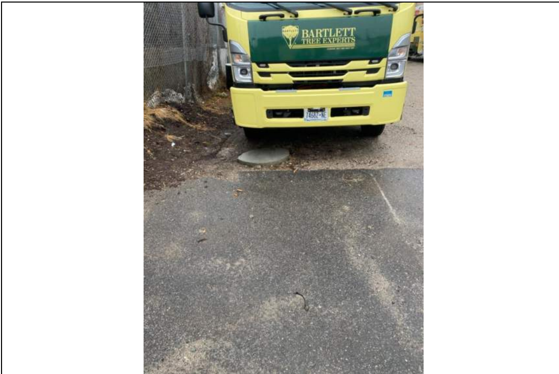
Photograph #13 – Protective metal manhole covering well vault MW-4.
