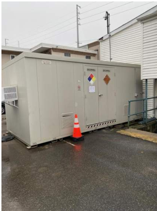
Photograph #4 – View looking southeast, north of the office/garage building. Newer secure storage locker for pesticides located at north end of the building.
