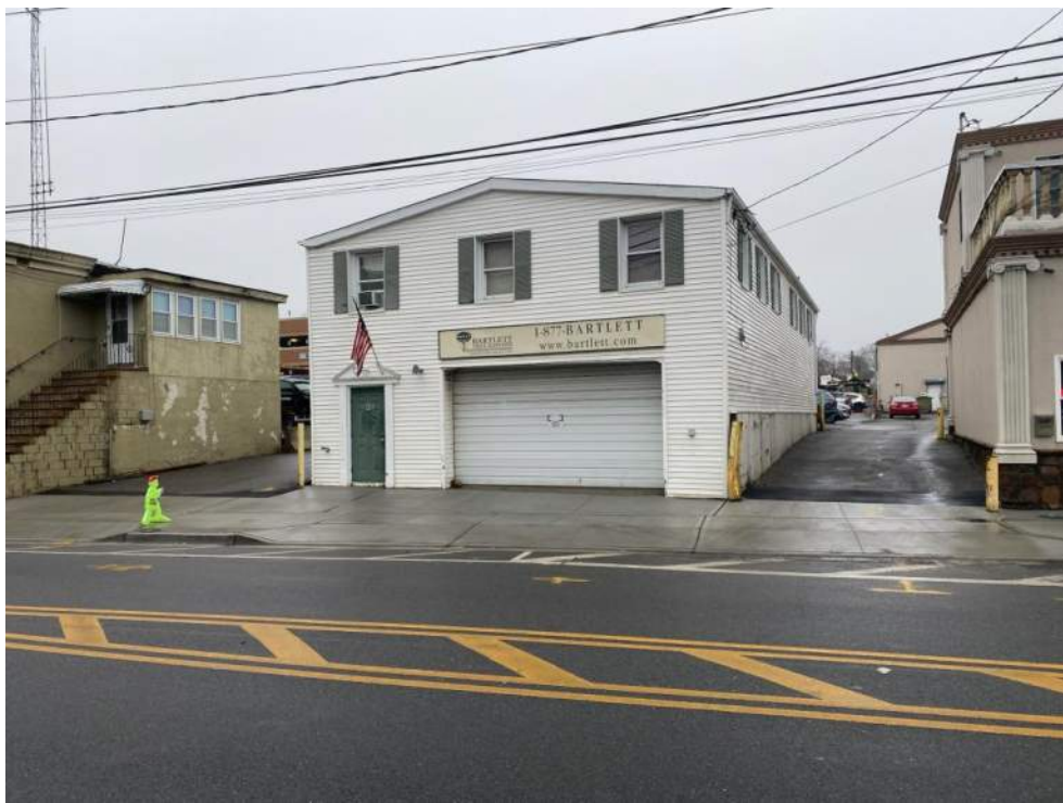
Photograph #1 – Bartlett Tree Experts office/garage building, viewed looking north from Union Avenue.
