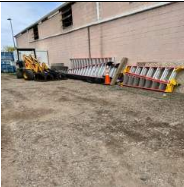
Photograph #2 – Area of remaining subsurface soil contamination in vicinity of boring SB-6. Original ground surface covered by aggregate.
