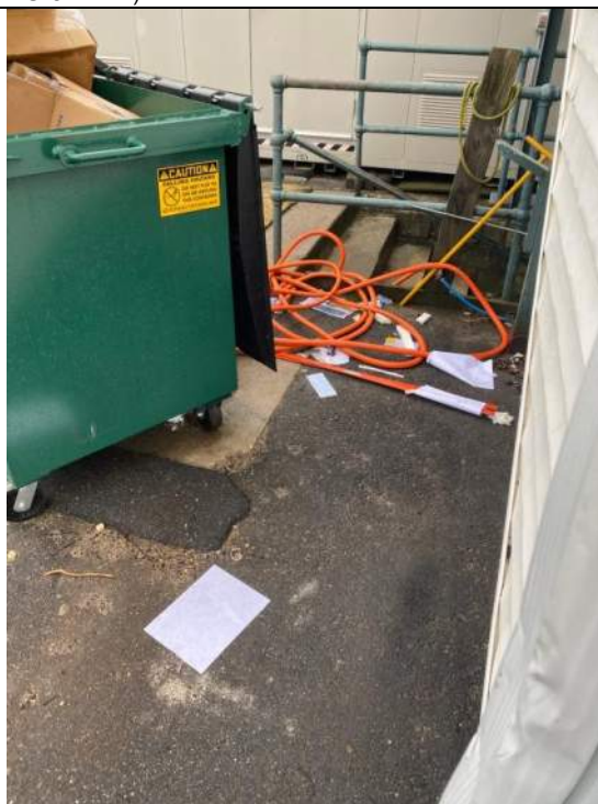
Photograph #18 – Area of remaining subsurface soil contamination, vicinity of former test pit TP-2. Area is covered by asphalt paving. During the 2008 RI, mercury was detected at this location above the Commercial SCO in the sample interval from 1-2 ft. bgs (Section 3 of PRR).
