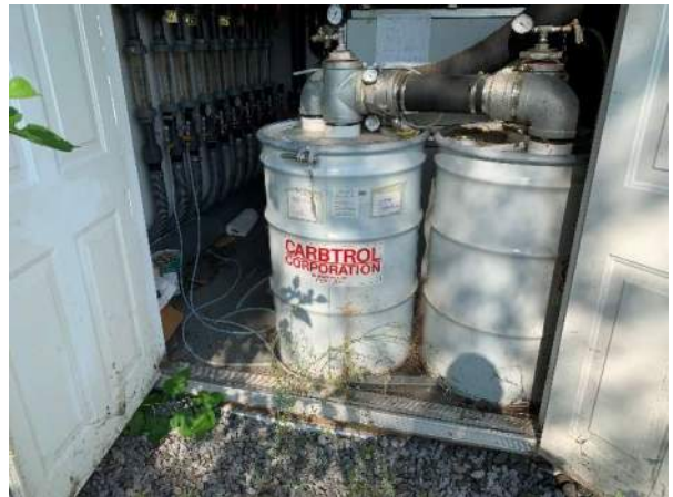
Photo 6: SVE system carbon vessels within system enclosure.
