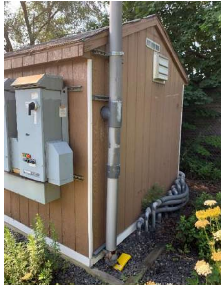
Photo 4: SVE system enclosure exterior with control panels and electrical components (left) and soil vapor recovery piping (right), facing southeast.
