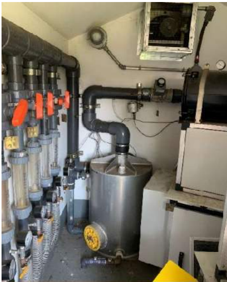
Photo 5: SVE system influent piping manifold (left), moisture knock-out tank (center) and blower (right) within system enclosure.
