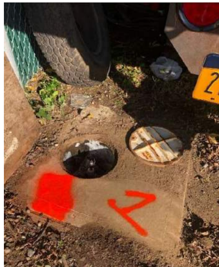
Photo 8: Soil vapor monitoring well (SVM-1).
