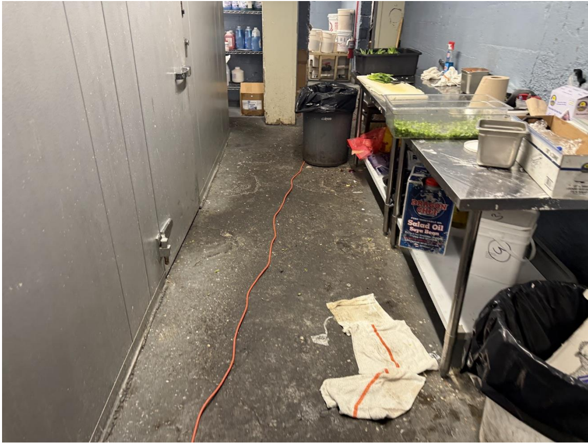
Photo 6, Basement of Restaurant
