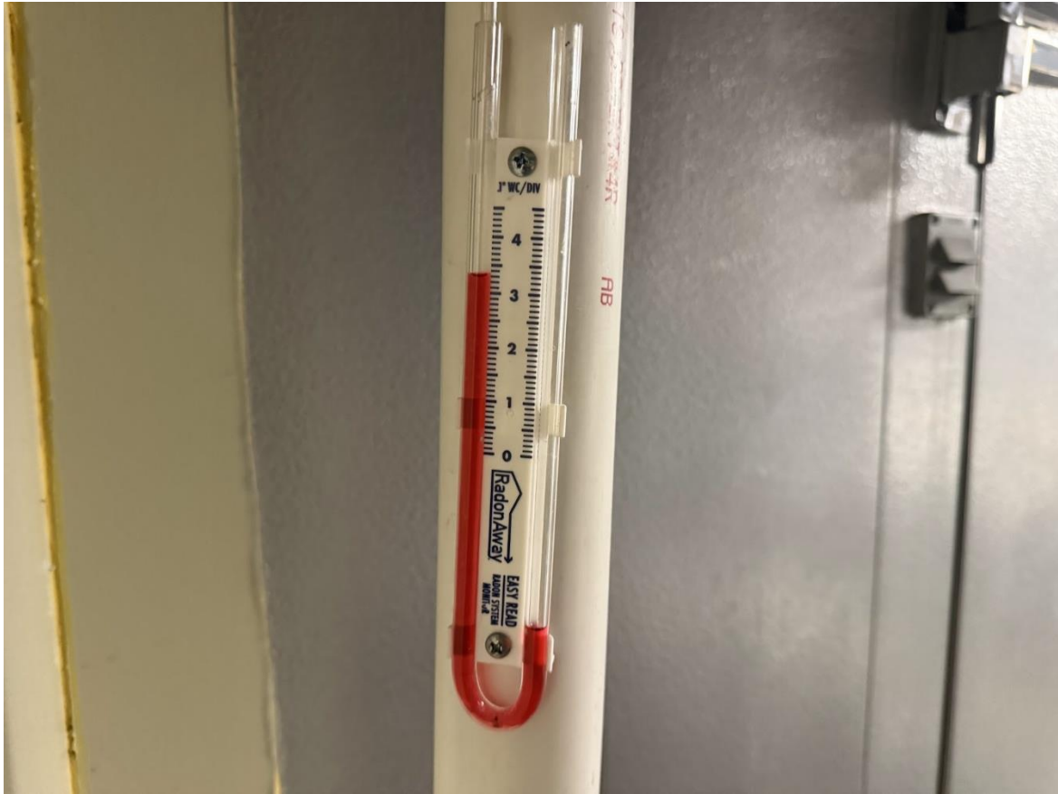
Photo 4, Basement of Restaurant
