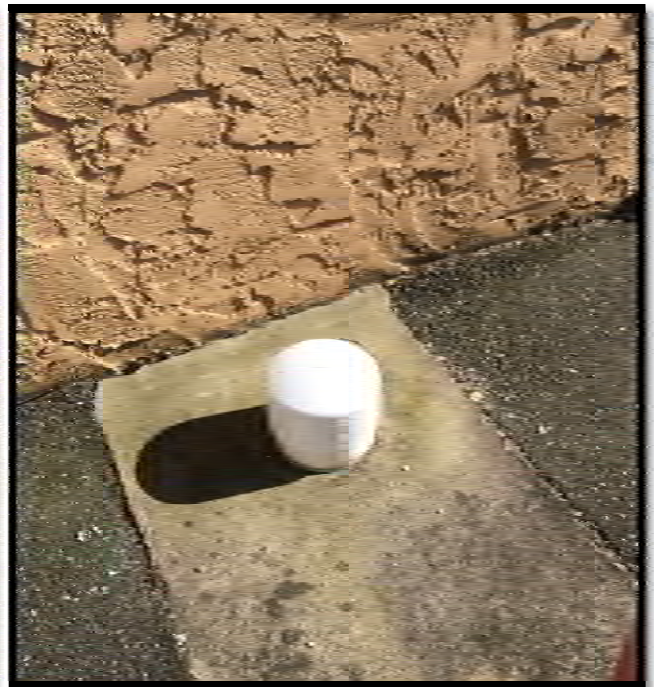
SVTT1 removed and capped
