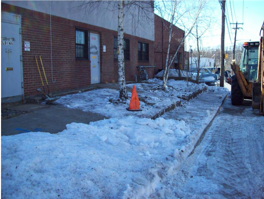
Photo 5. North side of building during site preparation.
