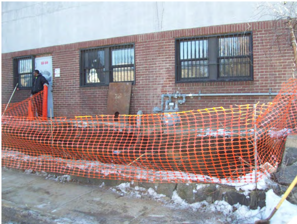
Photo 14. Southward view of western excavation.
