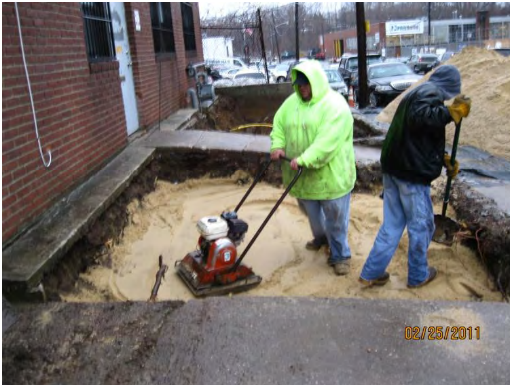
Photo 39. Backfill of central excavation area.
