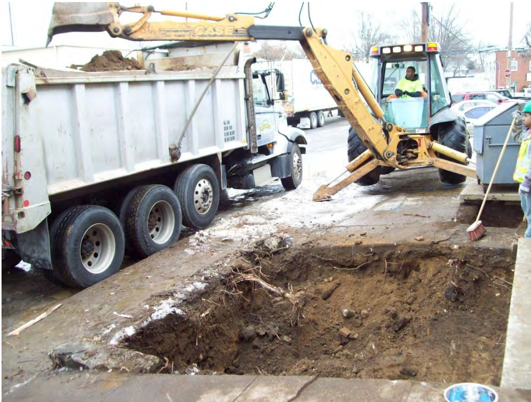
Photo 17. Eastward view of excavation area.
