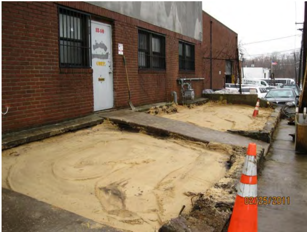
Photo 41. Backfill of central and western excavation areas.
