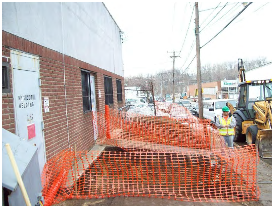
Photo 22. Westward view of excavation.
