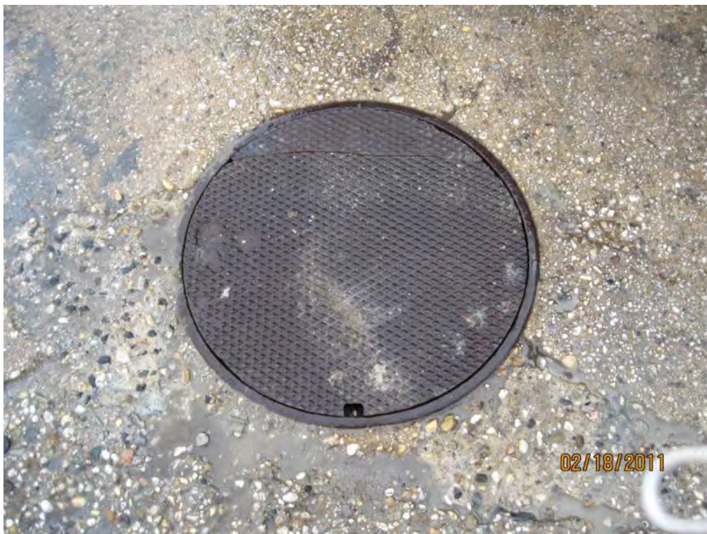
Photo 31. Cesspool following backfill.
