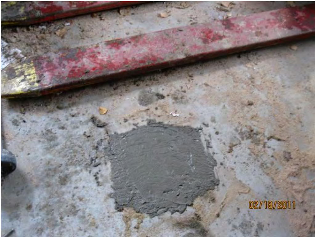
Photo 35. PZ-4 following decommissioning.
