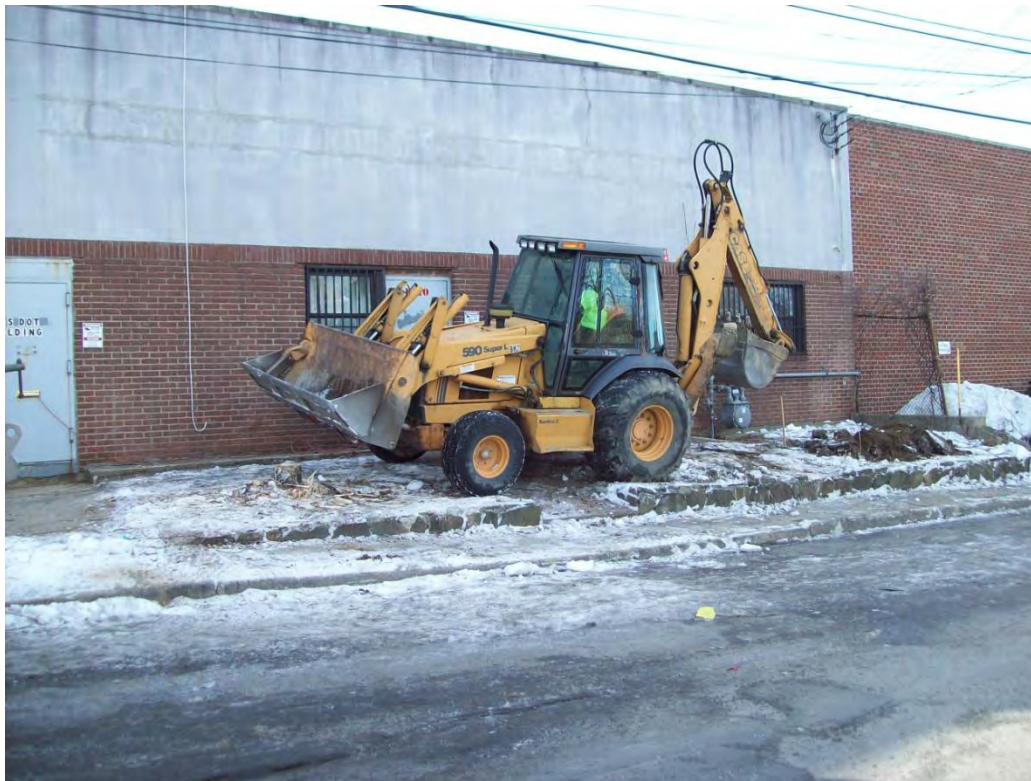
Photo 7. Excavation of soil on north side of building.
