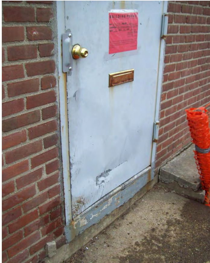
Photo 21. Door after repair.
