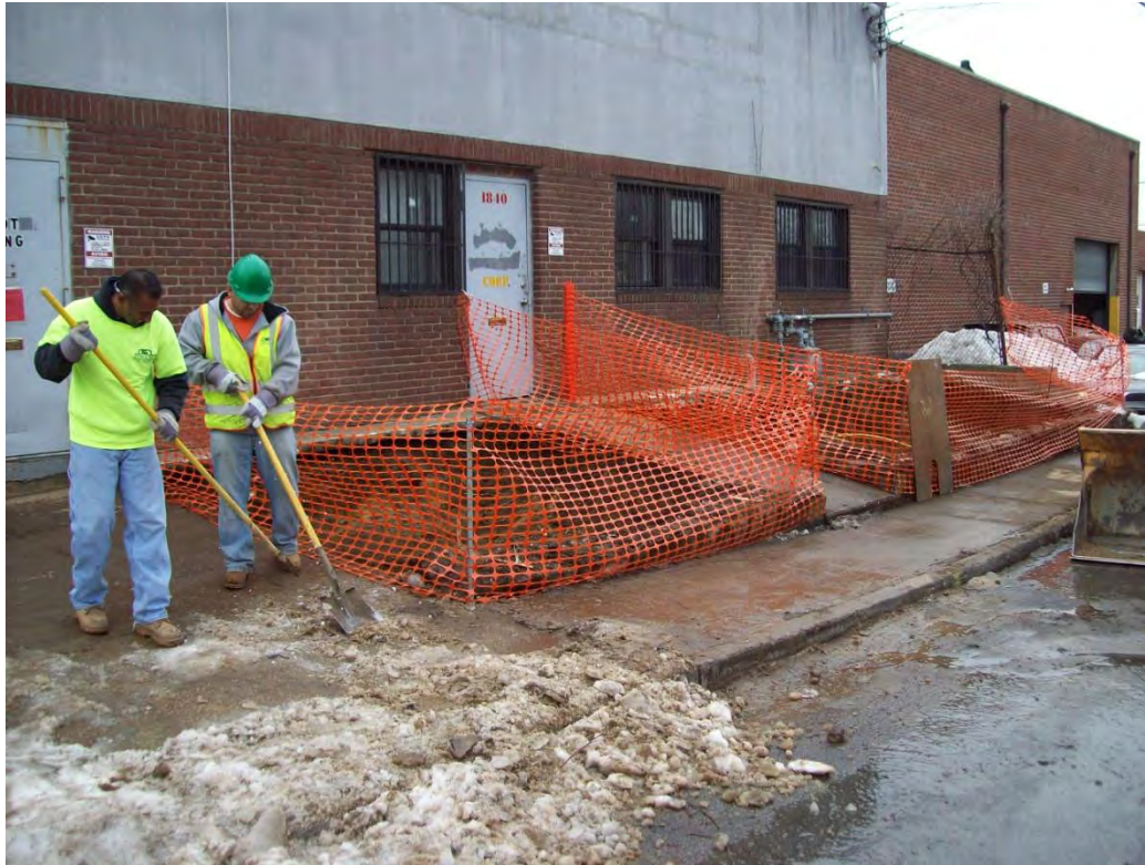
Photo 23. Western excavation area.
