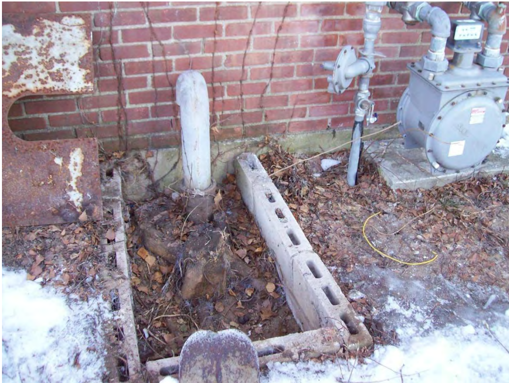
Photo 3. Sewer connection on north side of building.
