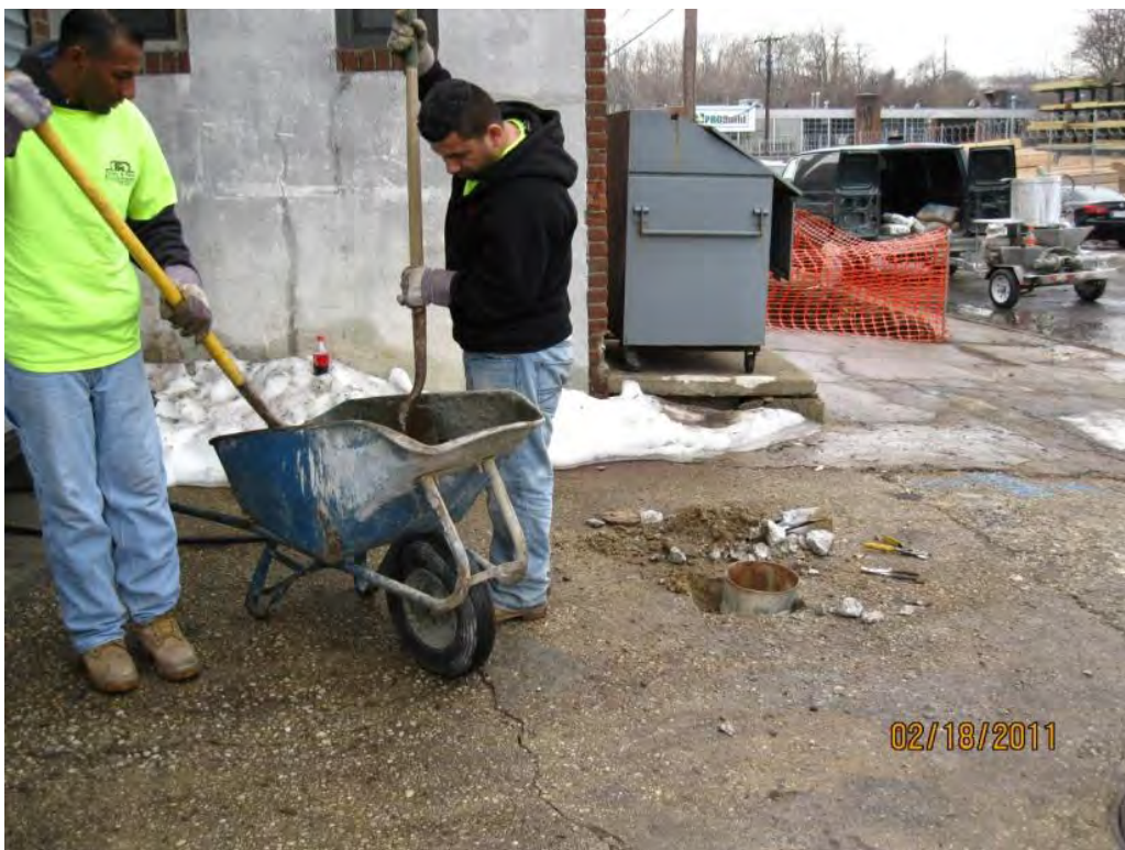
Photo 32. Decommissioning of PZ-2.
