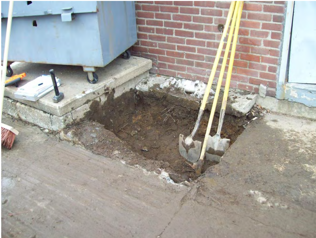
Photo 19. Easternmost excavation area, possible former flower bed.
