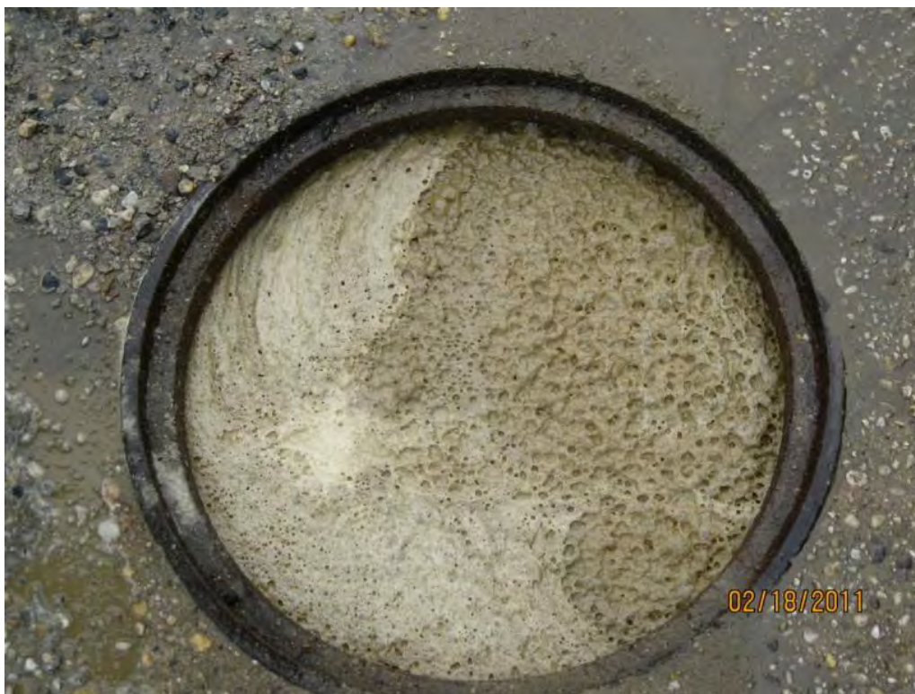
Photo 30. Cesspool backfilled to grade.
