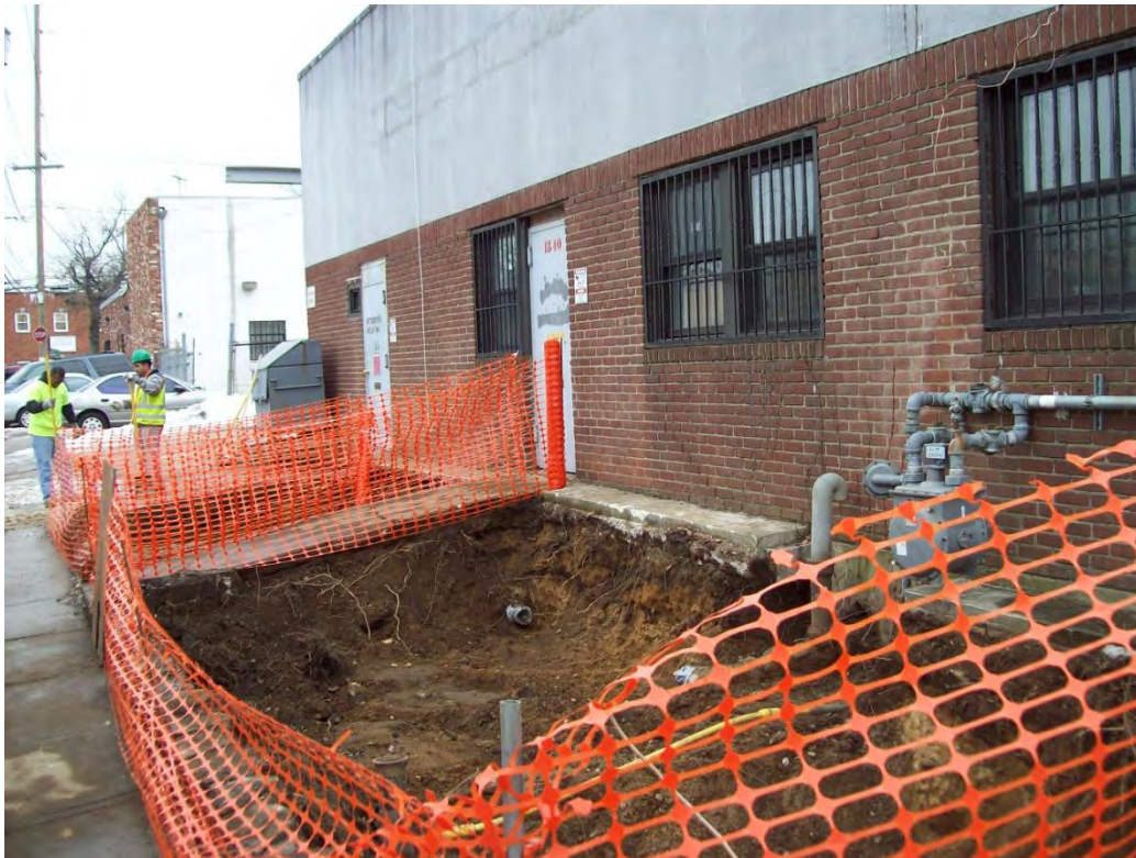
Photo 24. Western excavation area.
