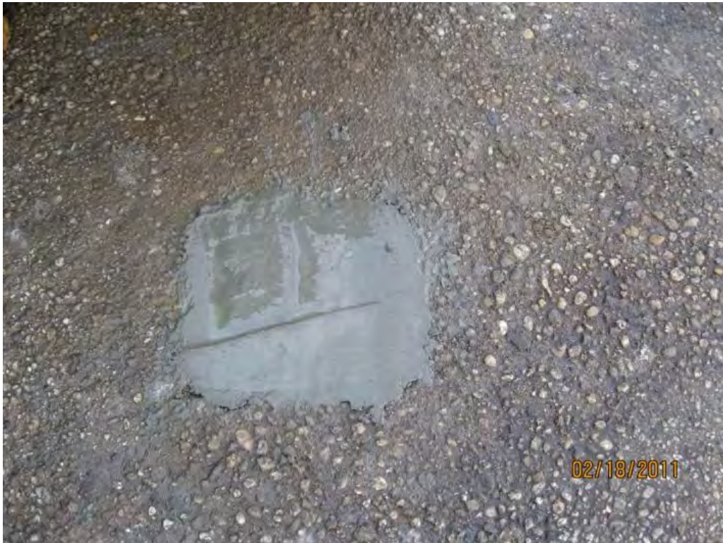
Photo 33. PZ-2 area following decommissioning.
