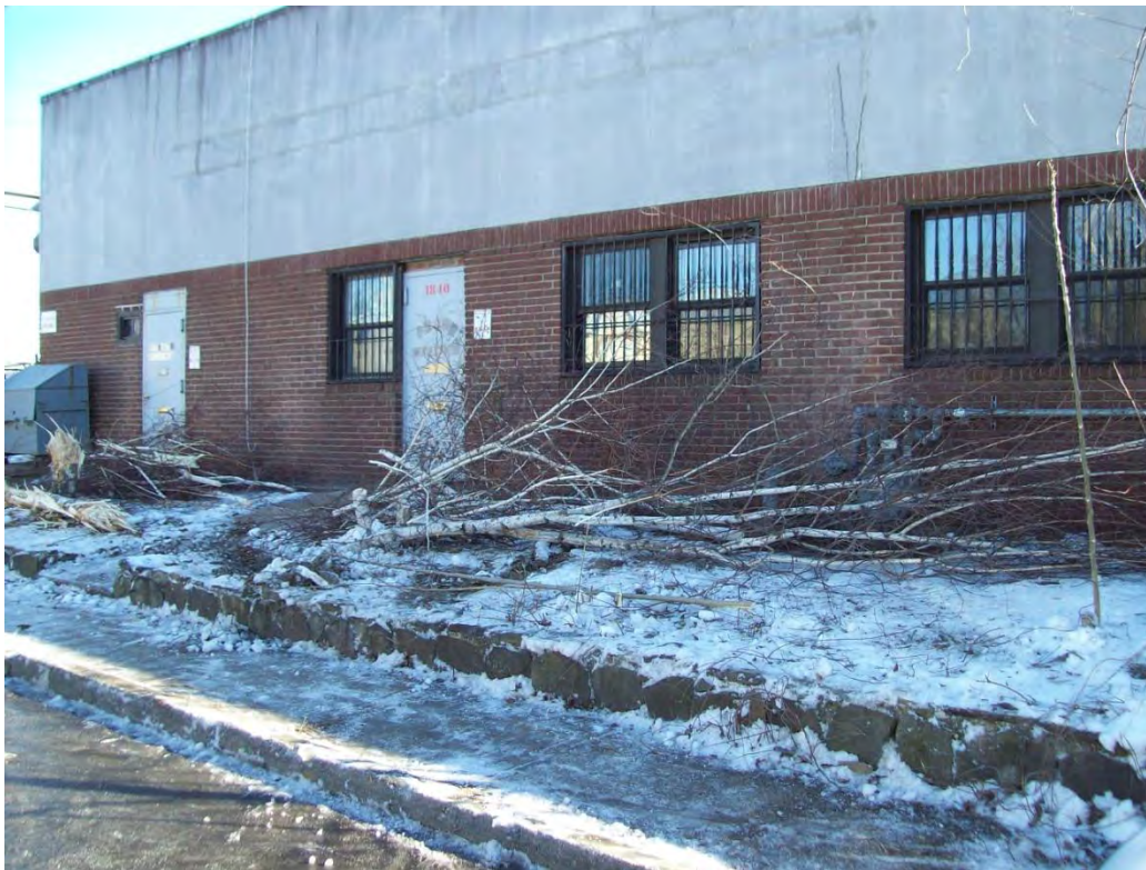
Photo 6. Removal of trees during site preparation.
