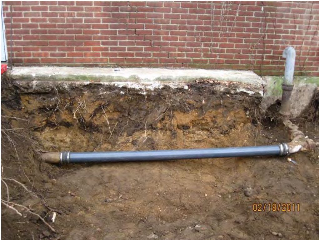
Photo 37. Repaired sewer line in western excavation.
