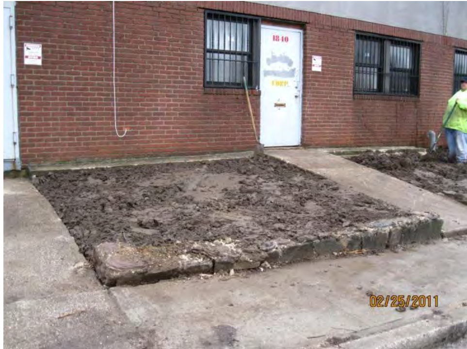
Photo 43. Completed backfill and restoration of excavation areas.
