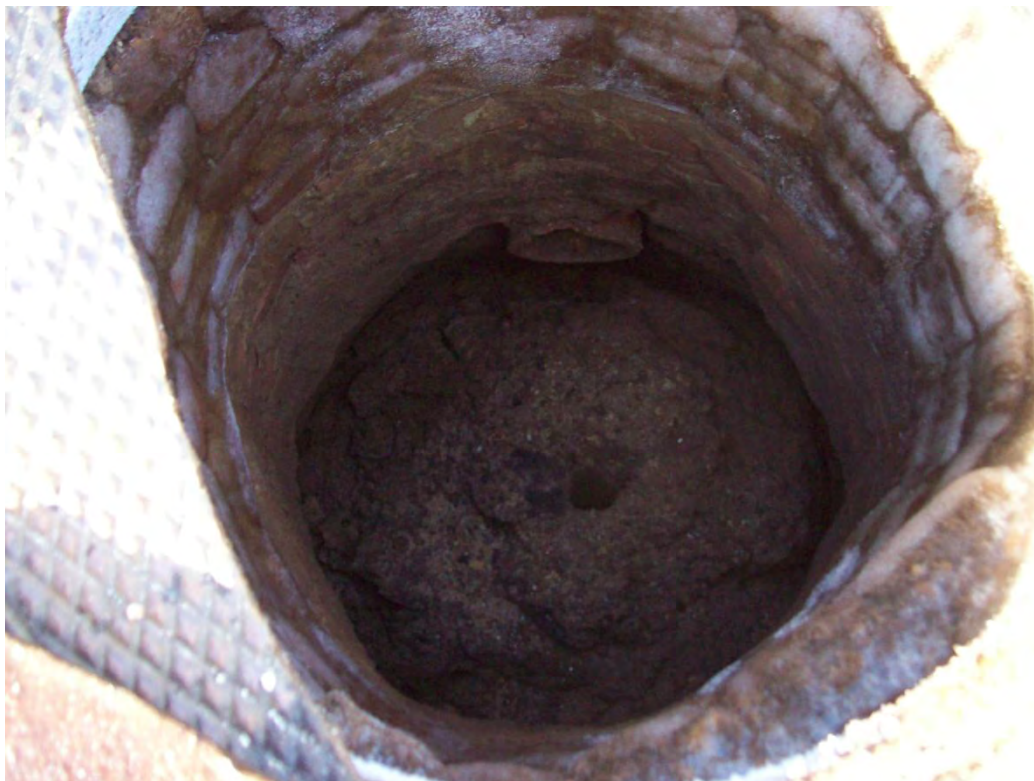
Photo 28. Inside of cesspool.
