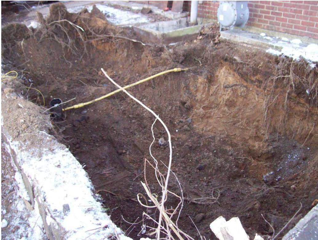
Photo 11. Gas line in western excavation area.
