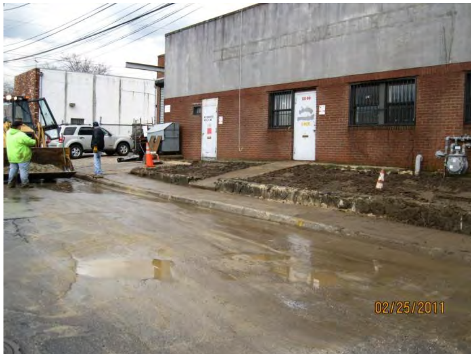
Photo 45. Completed backfill and restoration of excavation areas and street.
