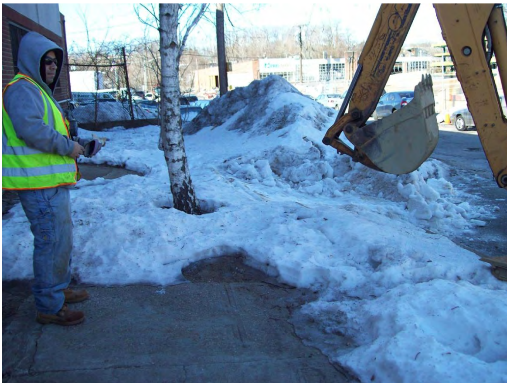
Photo 1. Snow removal during site preparation.
