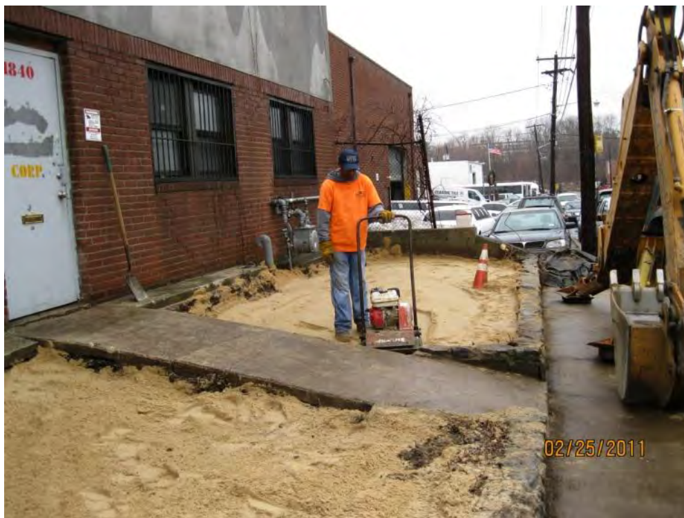
Photo 40. Backfill of western excavation area.
