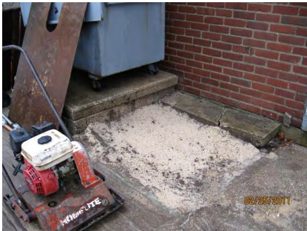
Photo 42. Backfill of eastern excavation area.
