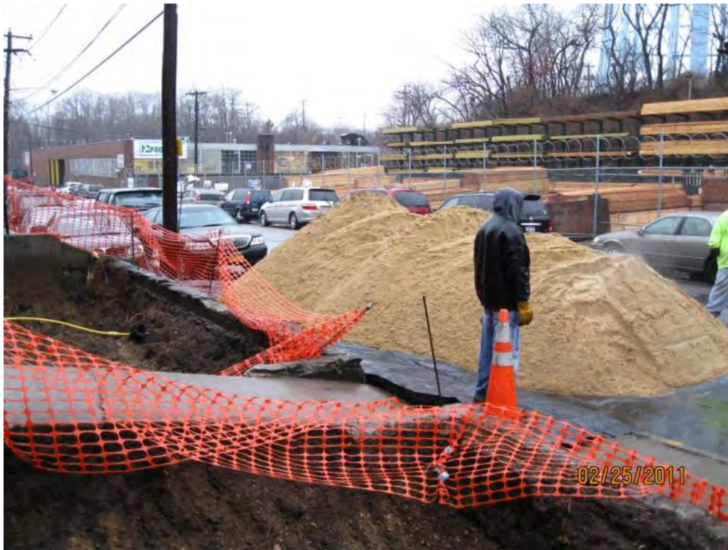
Photo 38. Backfill sand stockpiled on polyethylene sheeting.
