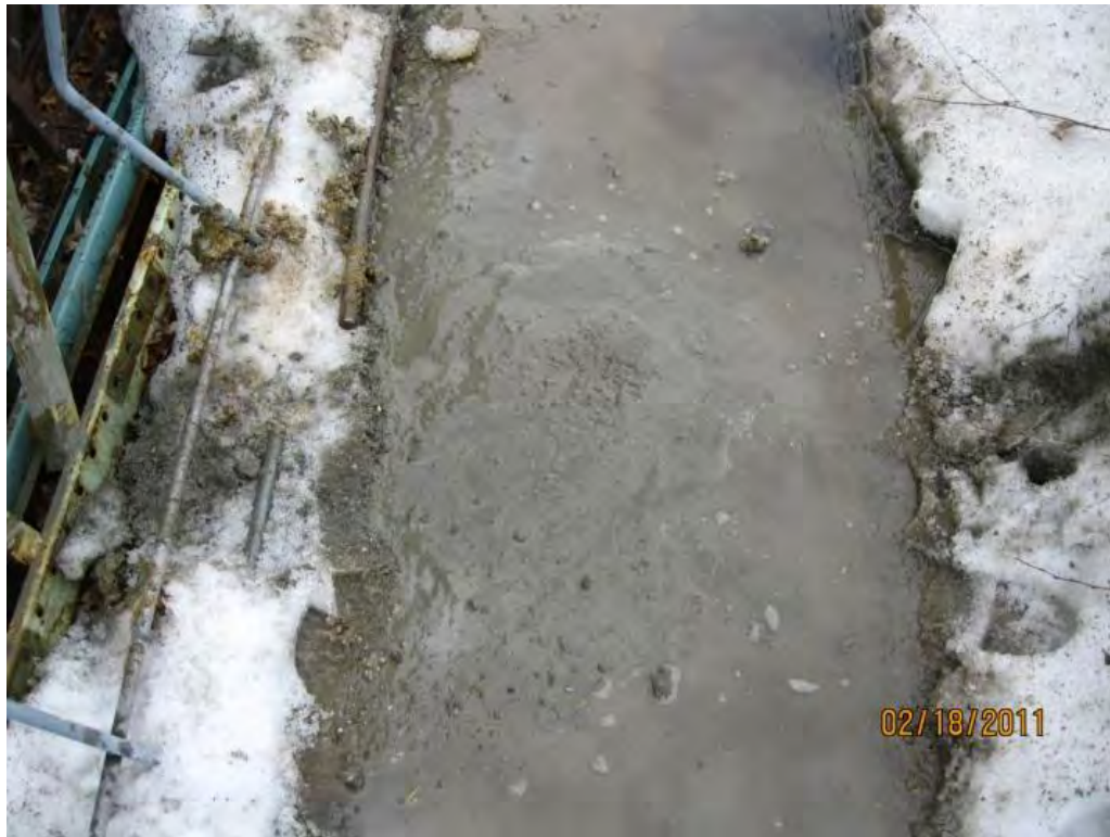
Photo 34. PZ-3 area following decommissioning.
