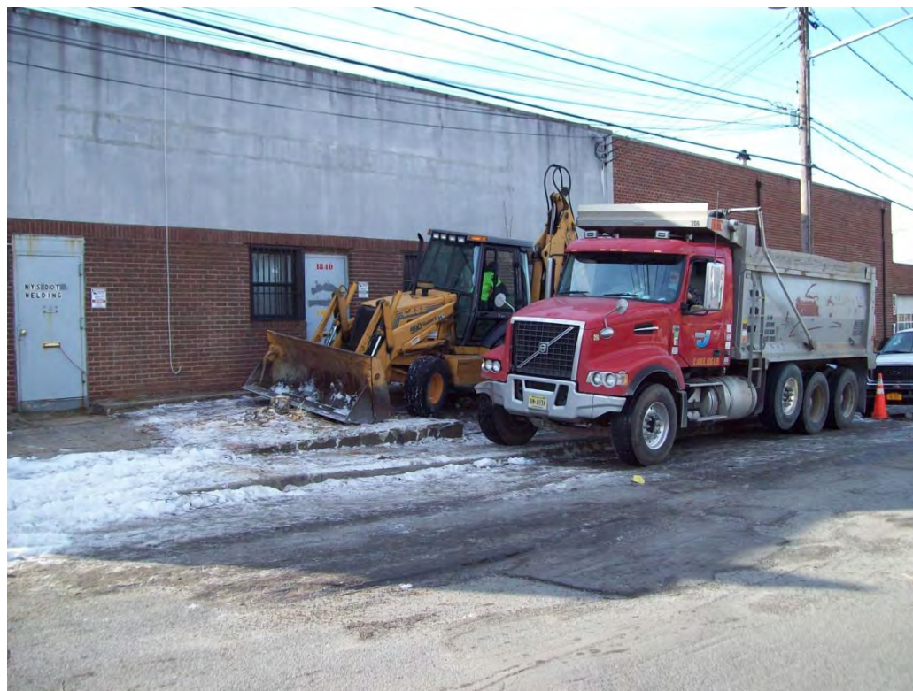
Photo 8. Loading of excavated soil for transport and disposal.
