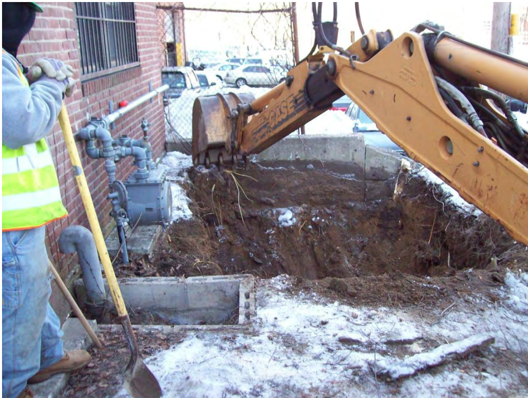
Photo 10. Westward view of the excavation area.
