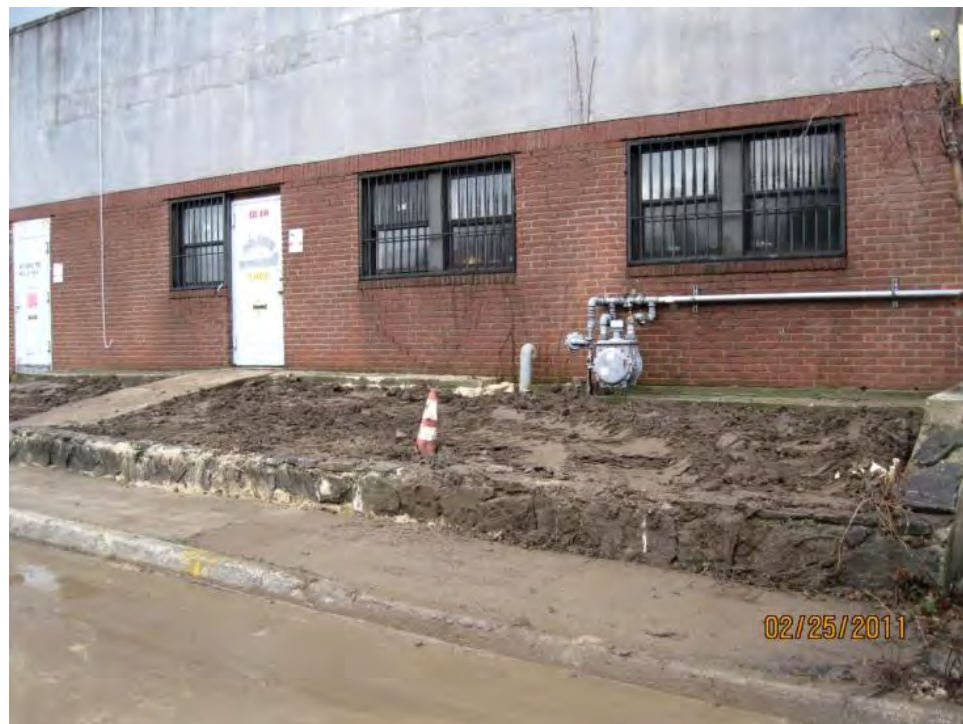
Photo 44. Completed backfill and restoration of excavation areas.
