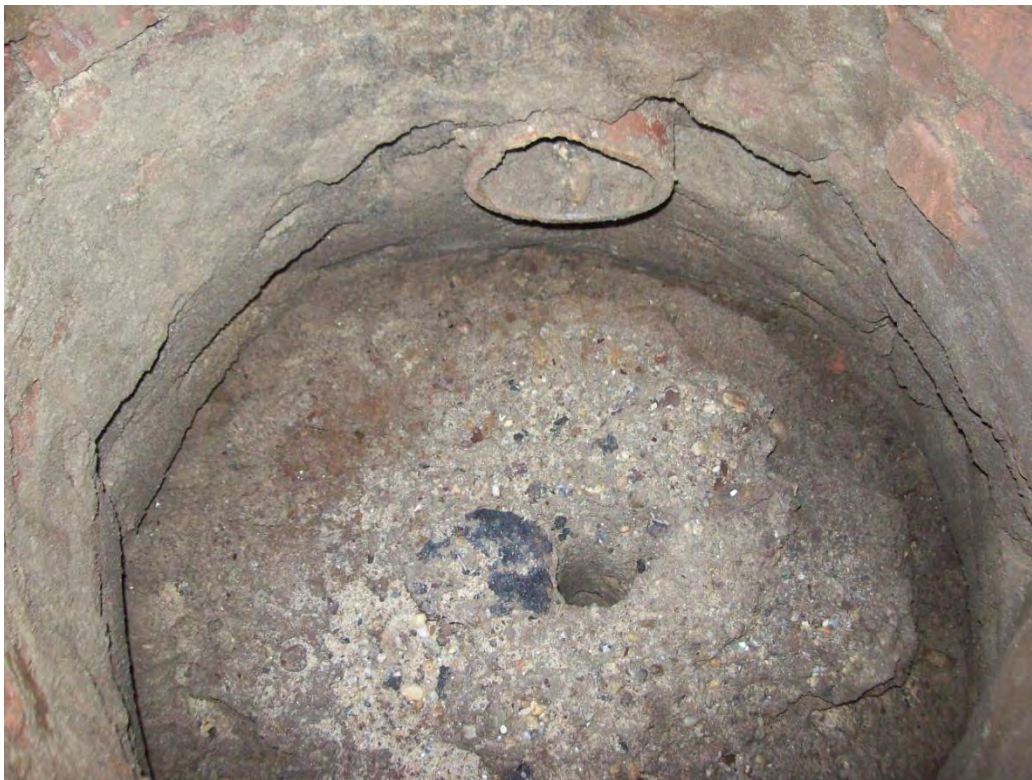
Photo 29. Inside cesspool. Apparent former soil borehole present.
