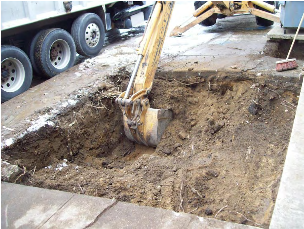
Photo 18. Eastward view of excavation area.
