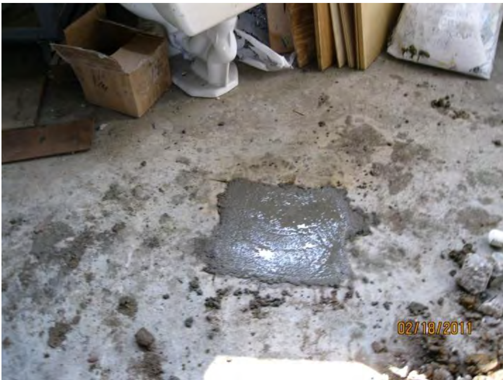
Photo 36. PZ-5 following decommissioning.
