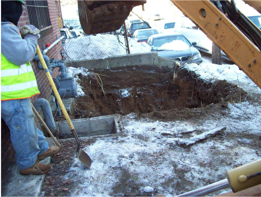
Photo 9. Excavation of site soil.
