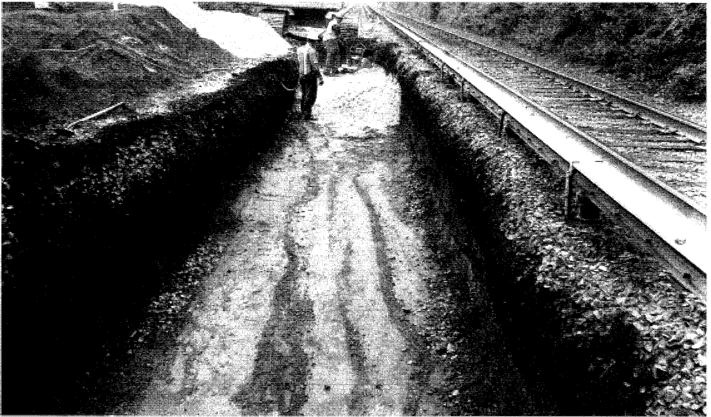
7. Backfilling of excavation (east side).
