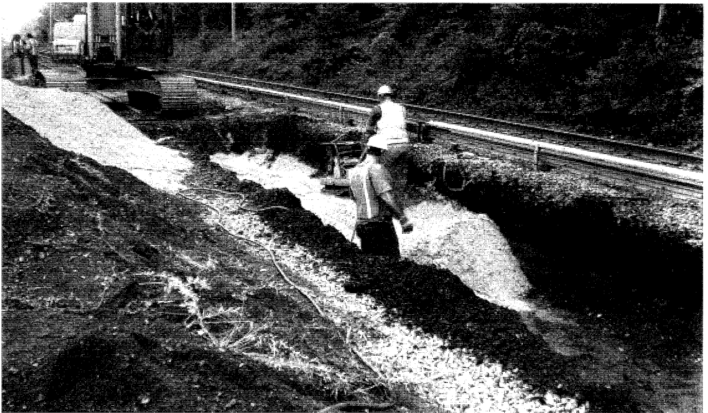
8. Backfilling of excavation (east side).
