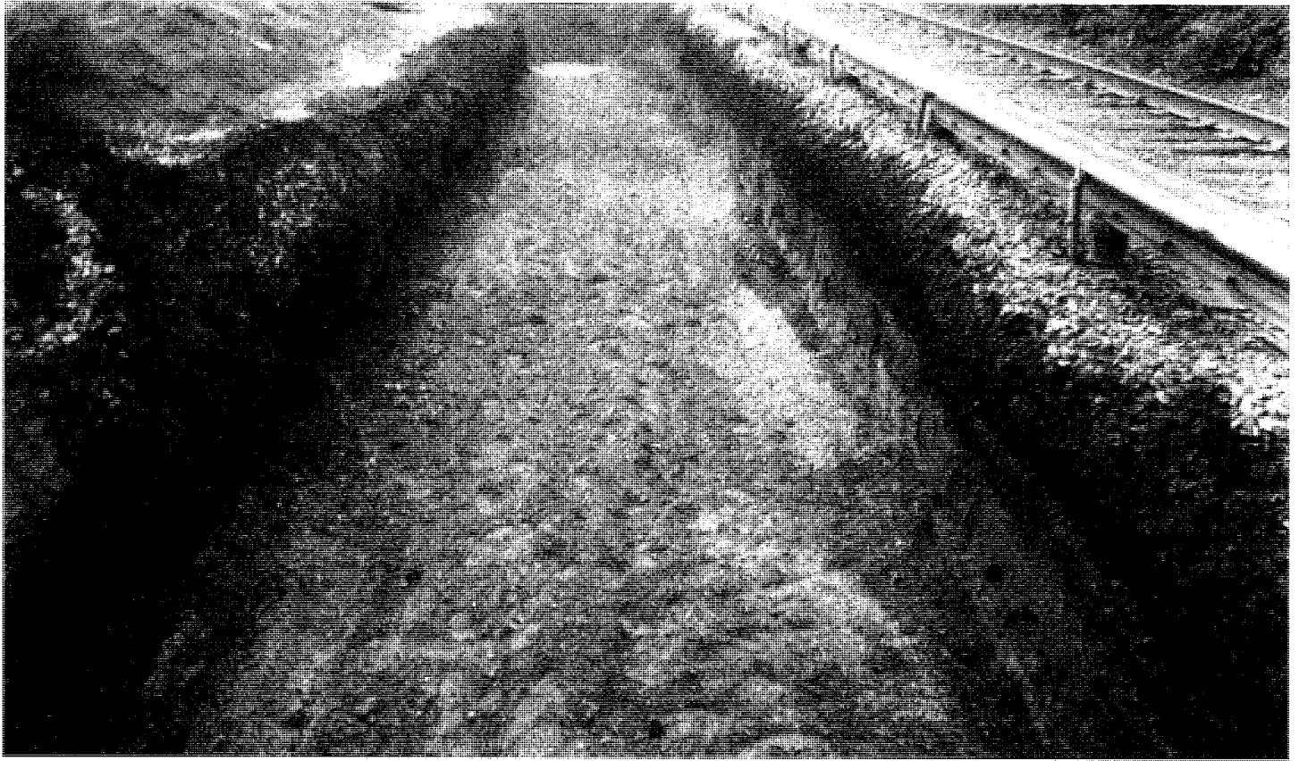
5. Completed excavation (east side).
