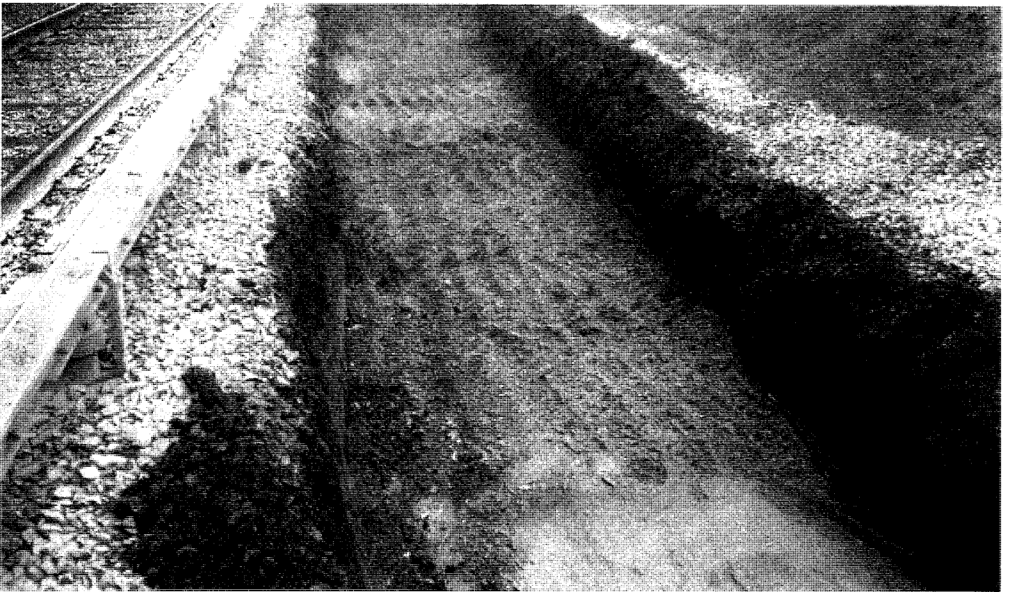
6. Completed excavation (west side).
