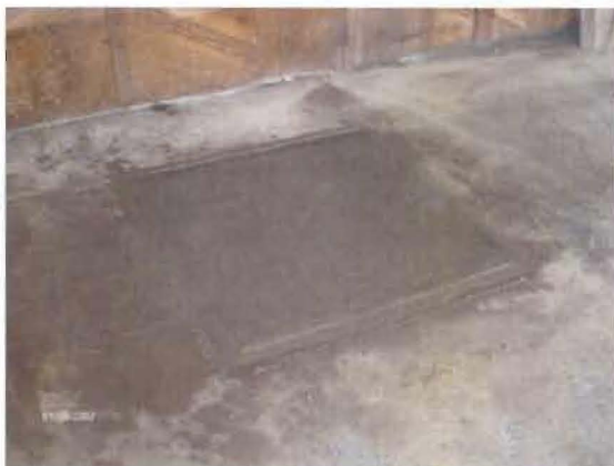
No. 6 View of concrete floor restoration.
