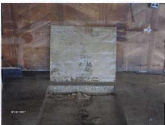
No. 3 View of moisture barrier and soils beneath concrete slab.
