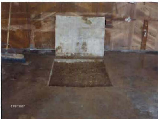
No. 5 Backfilled test pit and soil boring.
