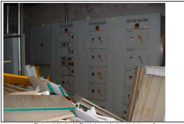
Photograph Number 11: Electrical room also has old shelving on floor as a possible hazard
