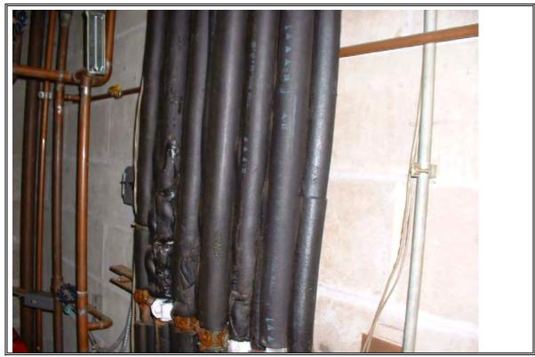
Photograph Number 4 typical pipe insulation of fiberglass foam material – south
