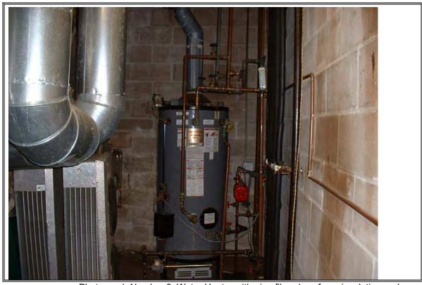
Photograph Number 3: Water Heater with pipe fiberglass foam insulation and rust staining on walls – looking East
