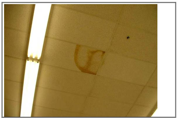
Photograph Number 18: typical ceiling tile with water staining in main shopping area – looking North
