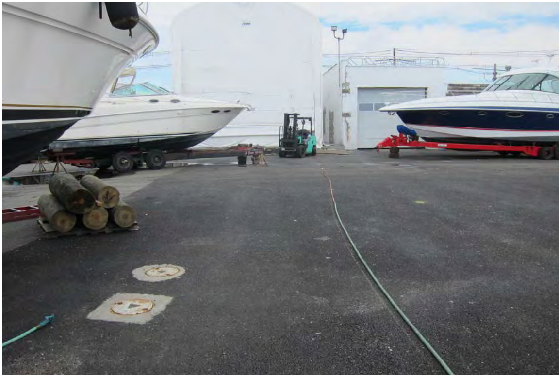
Overview of porous pavement- limited ponding
