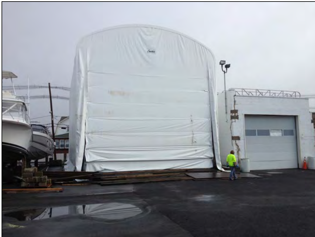
New sprung structure with an approximately 12" concrete slab on top of the existing asphalt. A boat was inside in the process of being repainted.
