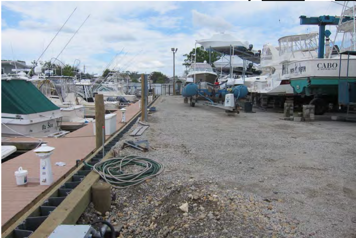
Southeastern piling system
