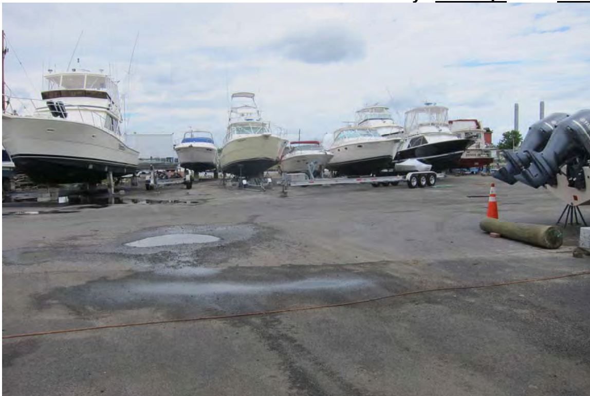
Southeastern corner area
