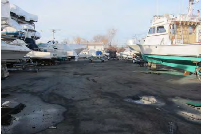
General site condition
