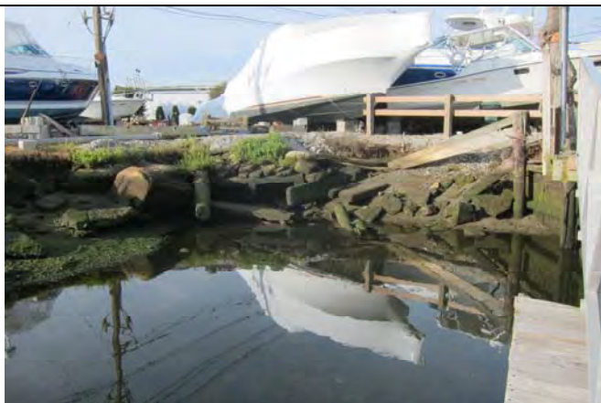
Storm drain on east side of site
