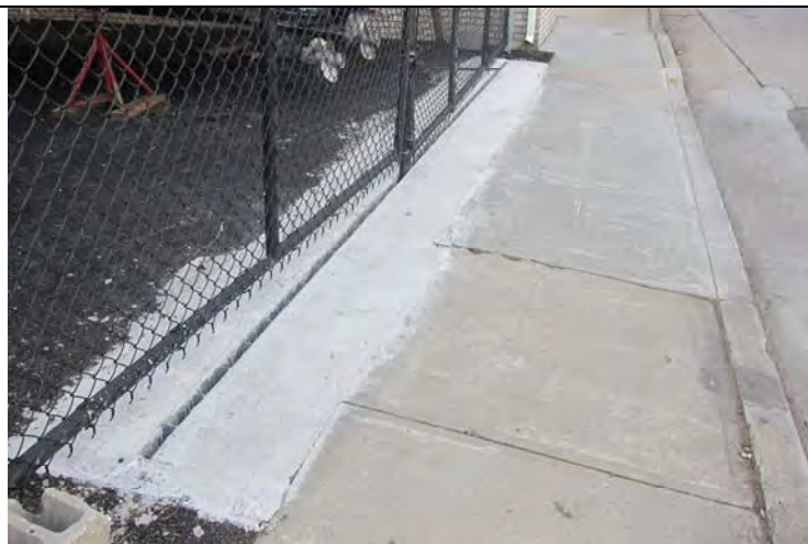
West storm drain
