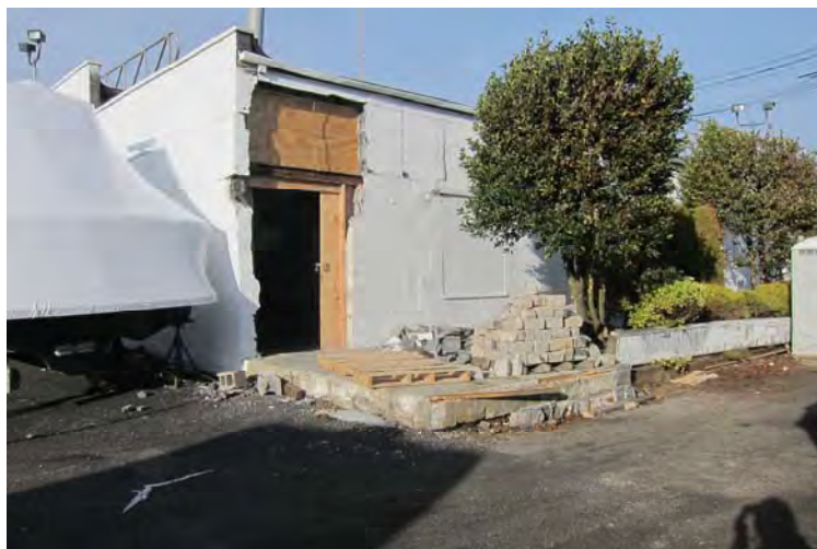
East side of warehouse building
