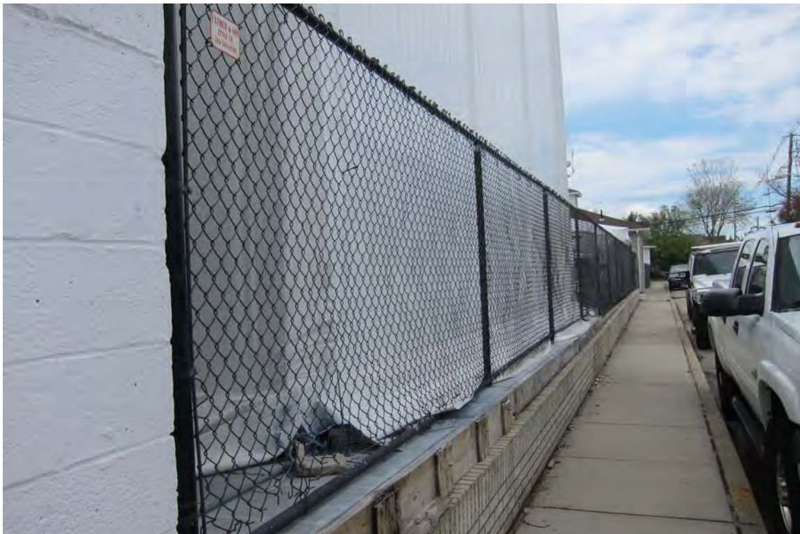
Perimeter fence is intact
