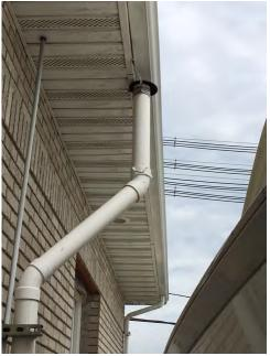
Crack in exhaust pipe of SSDS;
