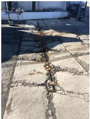
Cracked concrete around storm drain next to warehouse building.
