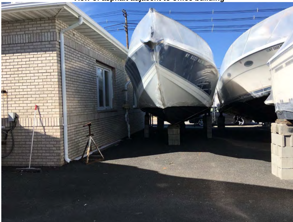
View of asphalt adjacent to office building
