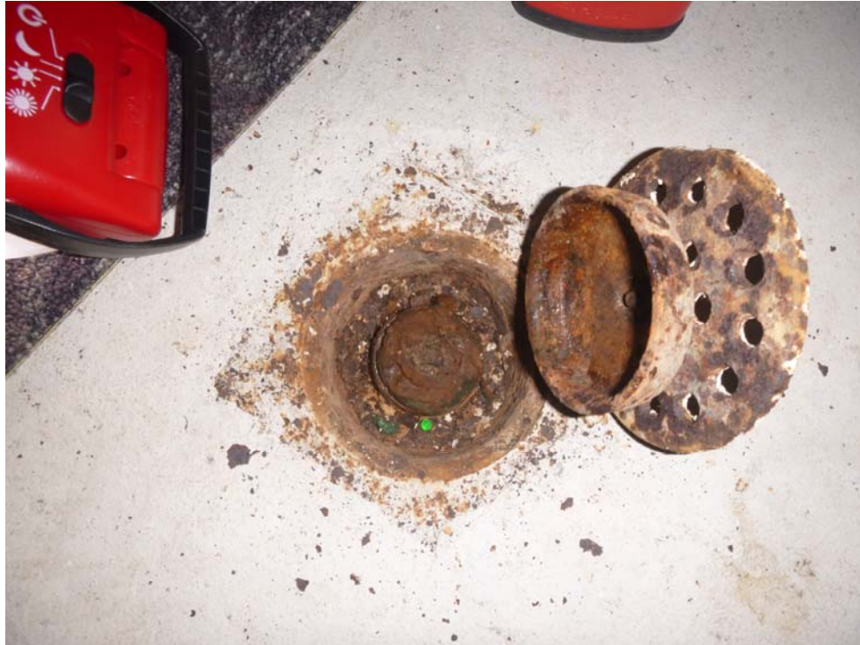
Photo 3: Opened metal drain plate with drain cap in bomb shelter.
