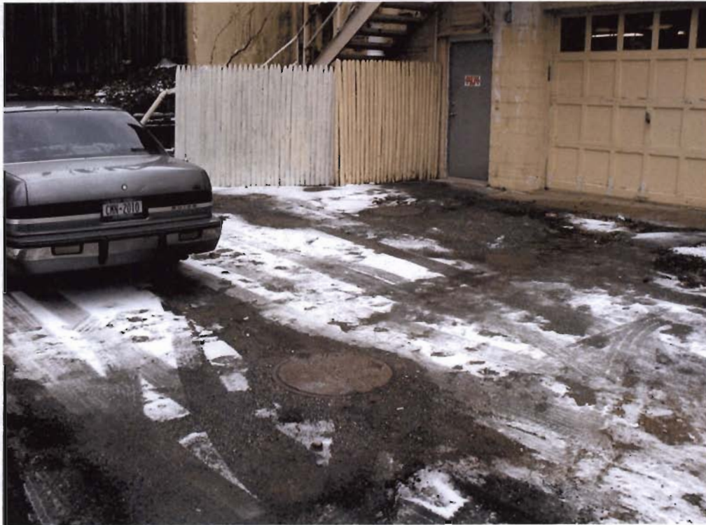
Figure 5 – Rear of 22-26 Railroad Avenue, location of septic system distribution box, septic tanks and cesspools, within paved parking area.
