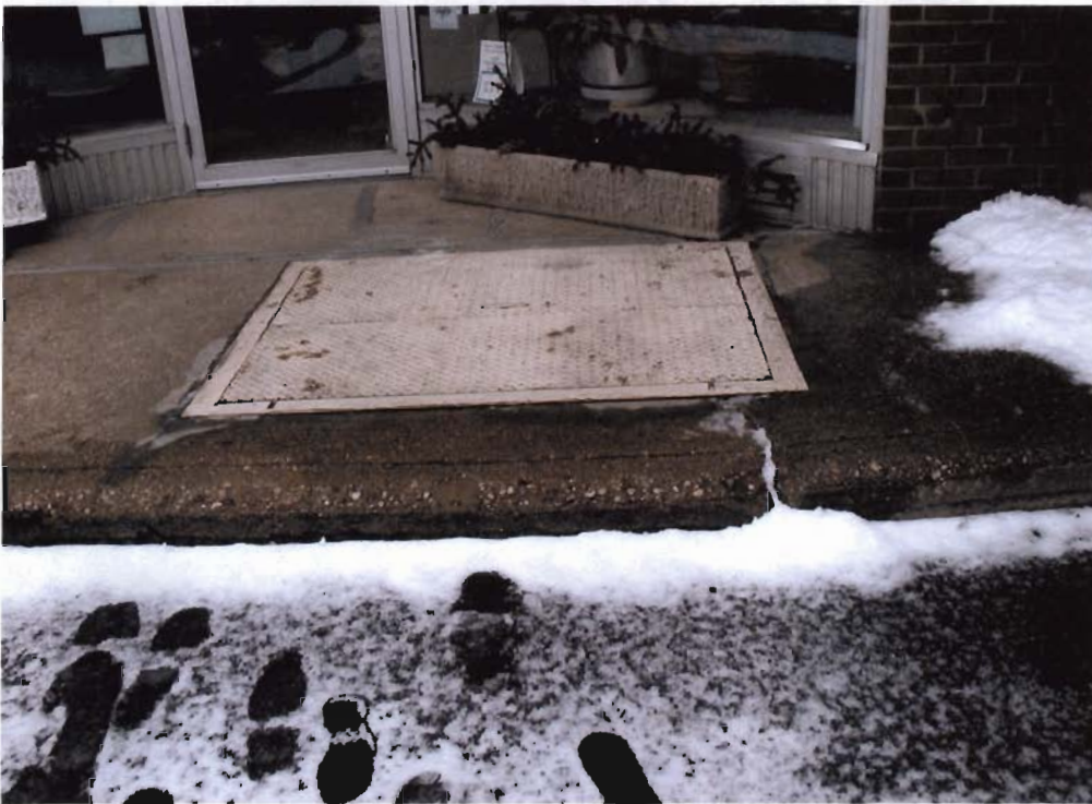
Photograph No. 2 – Access to partial basement at 26 Railroad Avenue (House DeGau).
