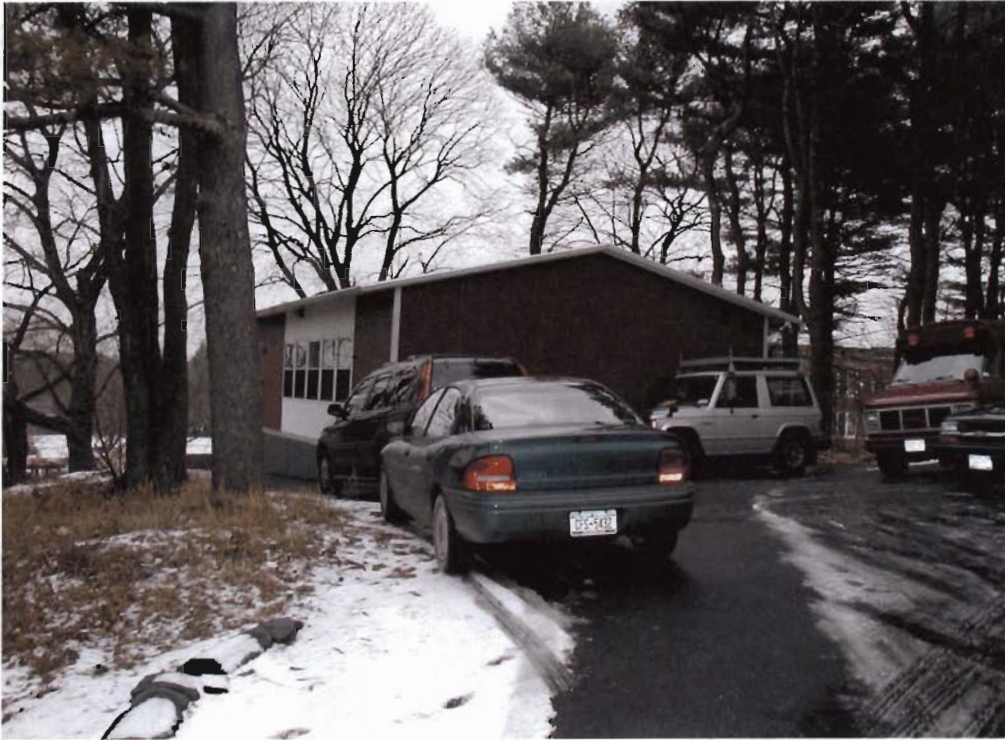
Figure 7 – Rear paved parking area with four storm water dry wells. Area formerly wooded undeveloped land. Abuts location of school maintenance building.
