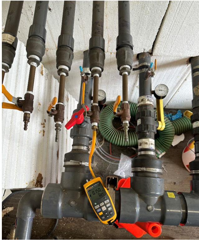
Photograph 3: View of the vacuum measurement from MP-2.
