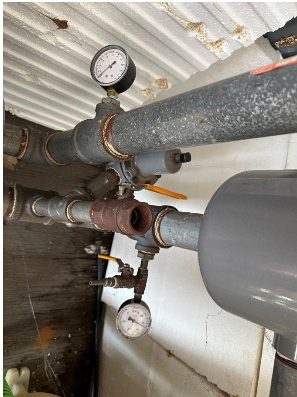
Photograph 2: View of the blower vacuum gauge.
