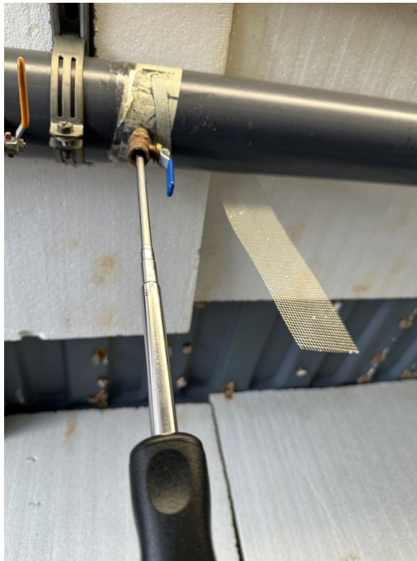
Photograph 6: View of the blower discharge port.
