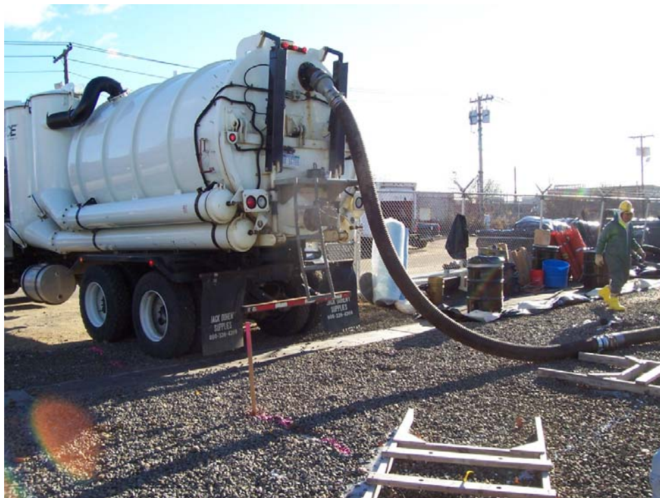
Guzzler truck, used to excavate contaminated soil.
