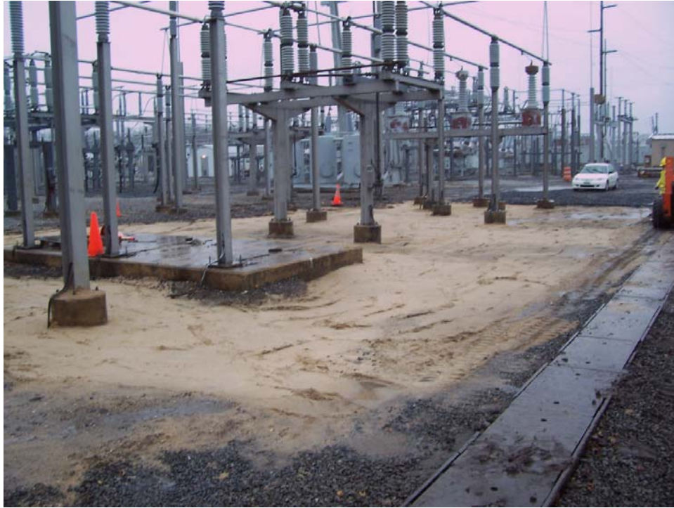
Northeast corner area, prior to completion of backfill installation and compaction.
