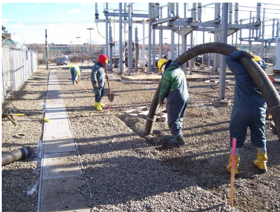
Excavation of perimeter trench.
