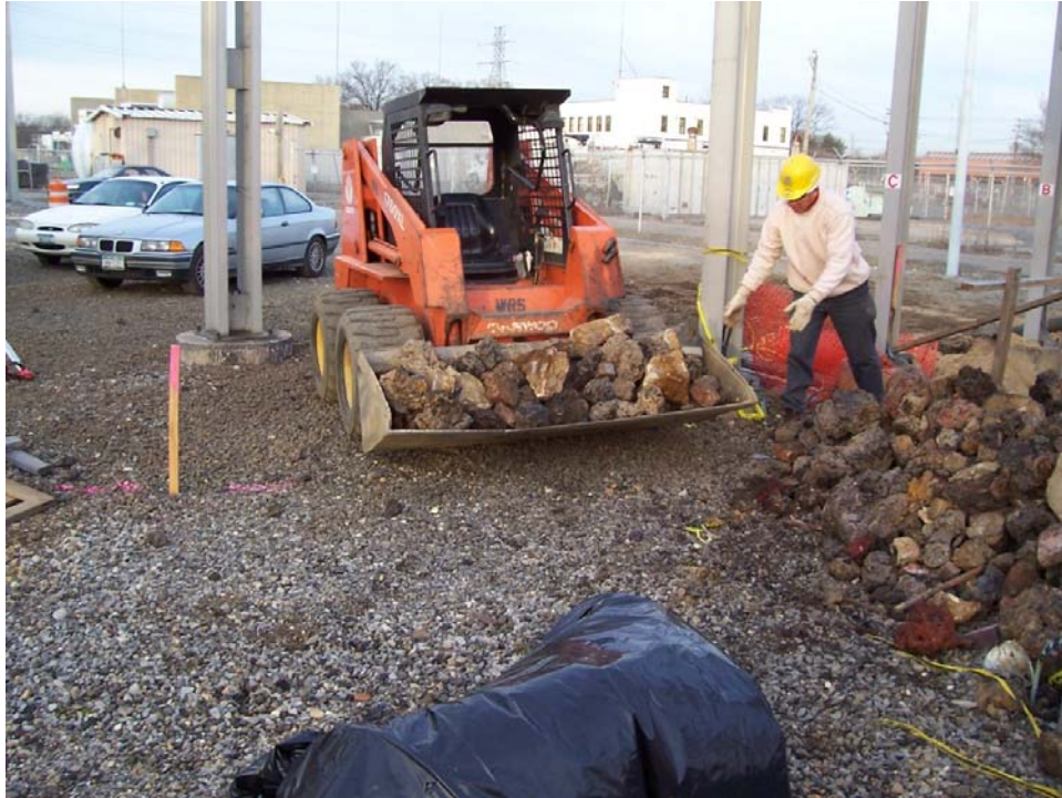
Removal of slag and brick material, utilizing a Bobcat.
