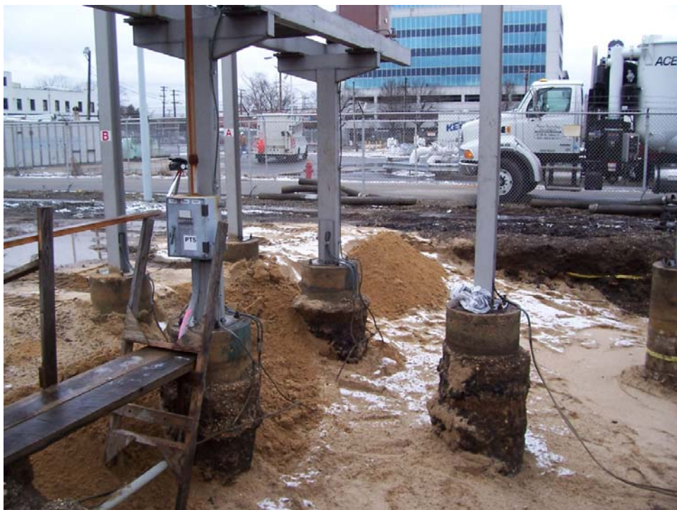
Backfilling of the western portion of the excavated area.
