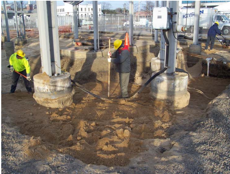
Installation and compaction of clean fill in the eastern portion of the excavated area.
