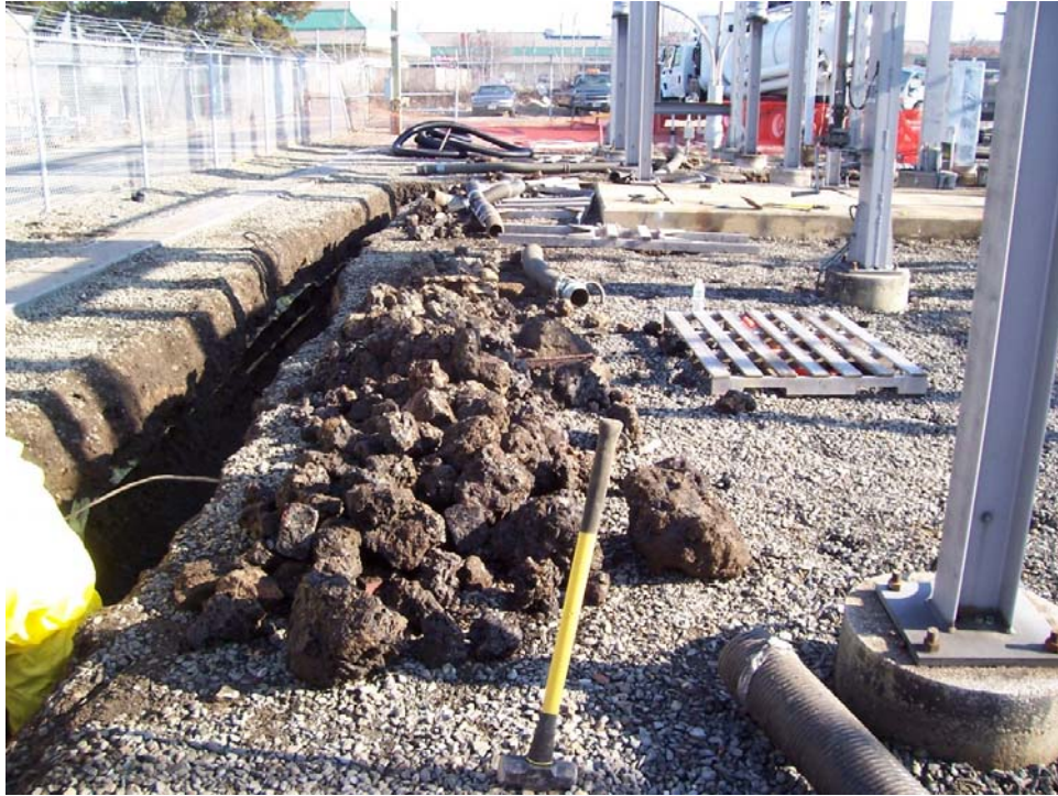
Excavation of perimeter trench, showing a high percentage of slag and brick material, observed throughout the excavation area.
