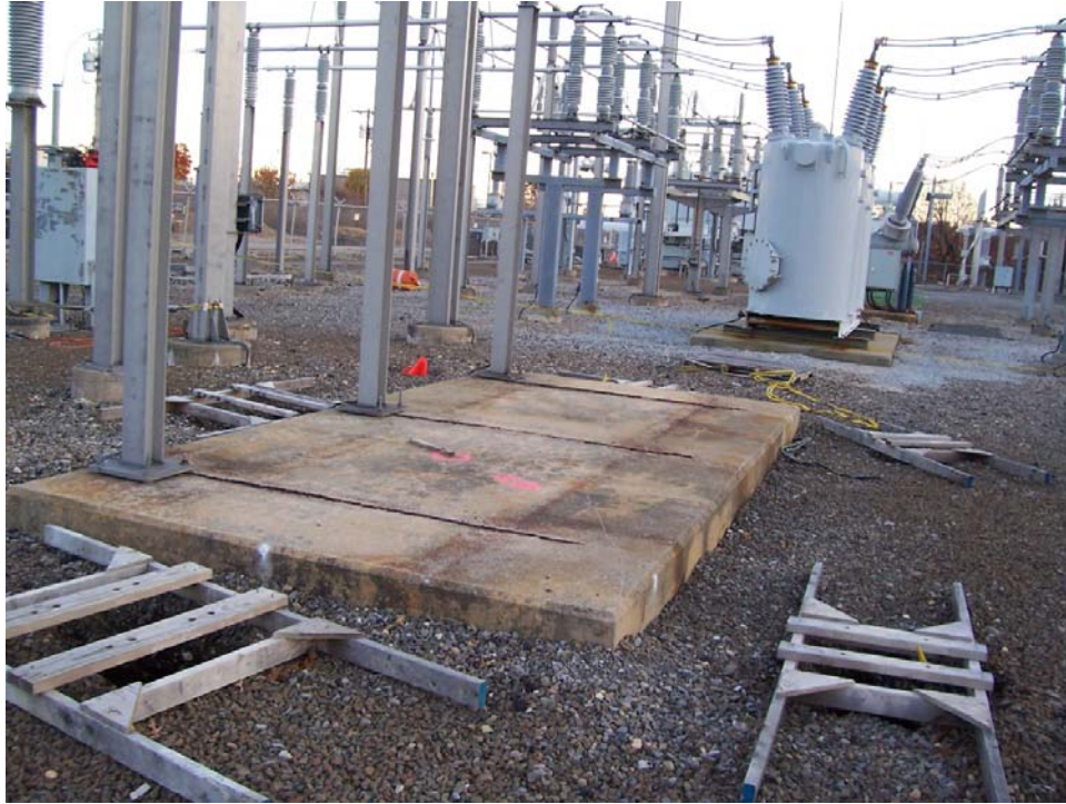
Northeast corner of the East Garden City Substation, prior to IRM activities.
