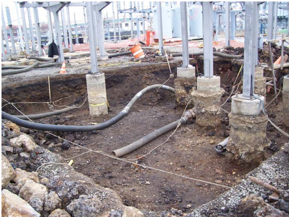
Western portion of excavated area, showing the protected grounding grid, left in place.
