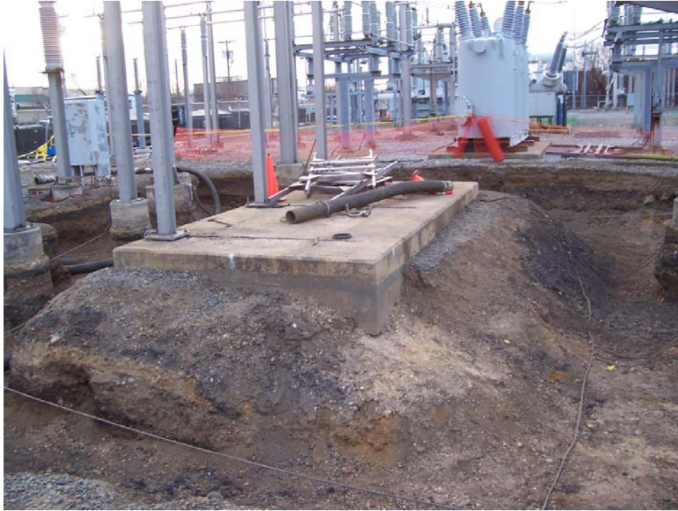
Sloped sides of the excavation, surrounding the load-bearing concrete pad.
