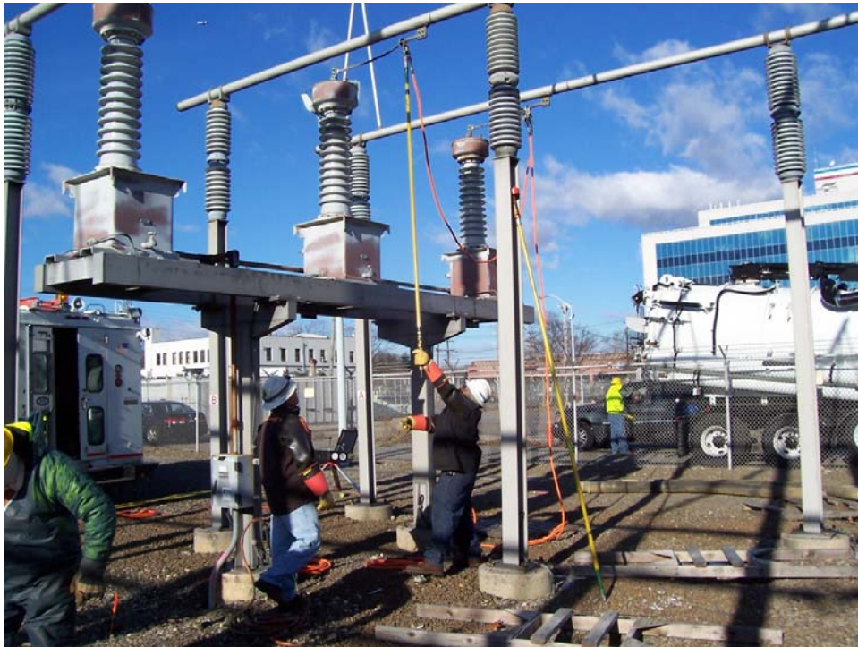
Installation of grounding cables, prior to initiation of IRM activities.
