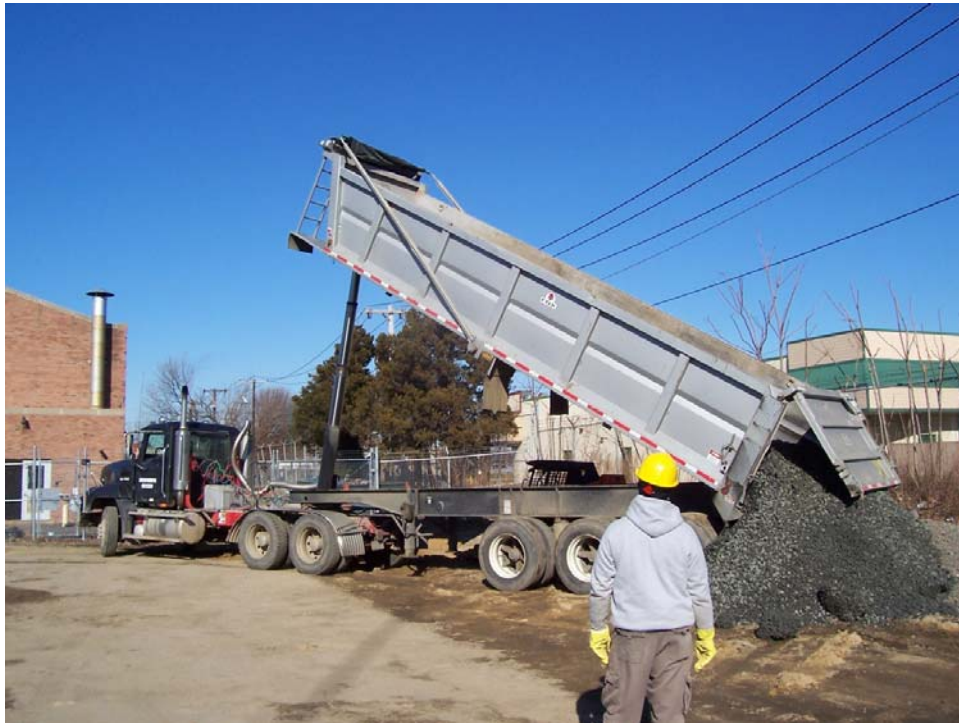
Delivery of crushed stone, to be installed subsequent to substation upgrade activities.
