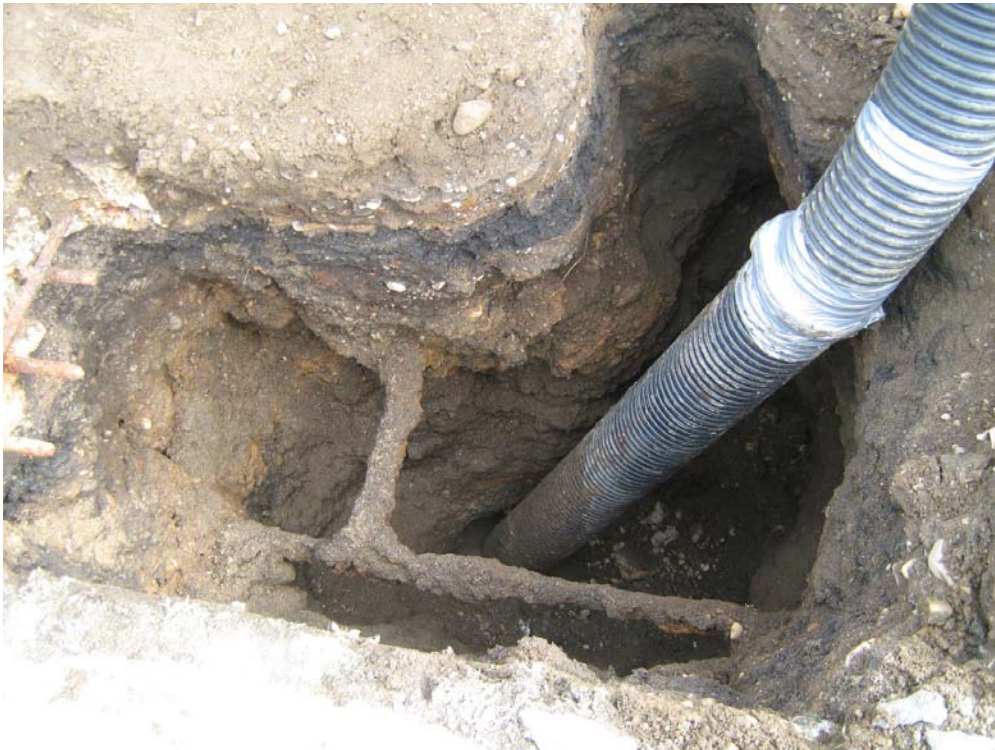
Photo 4: Test pit EGCTP-01 excavation showing black stained soil
