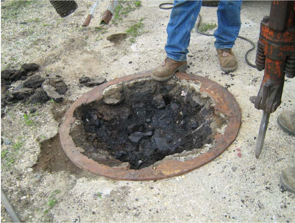
Photo 9: Solidified tar and sediment in the gas holder foundation suspected gas distribution pipe.
