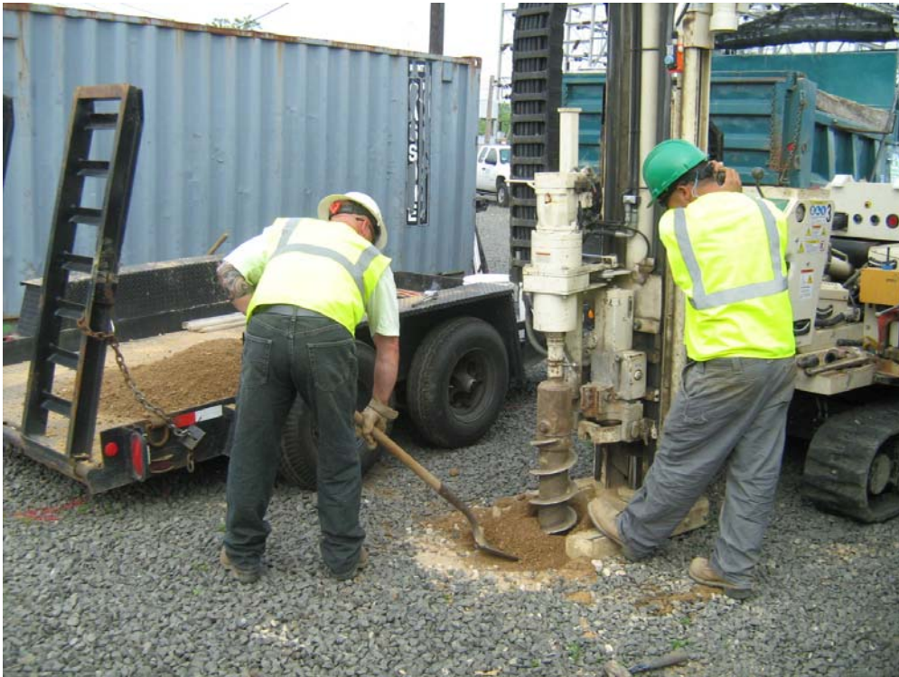
Photo 10: Installation of groundwater monitoring well EGCMW-05 utilizing a hollow stem auger rig
