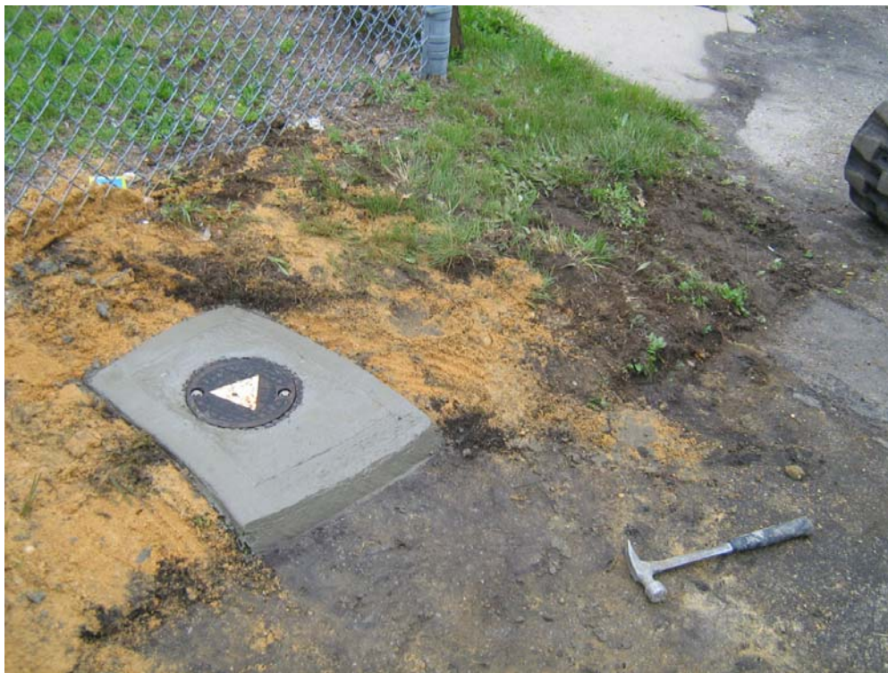
Photo 11: Completed groundwater monitoring well EGCMW-02
