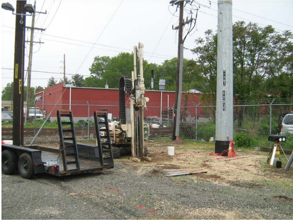
Photo 7: Geoprobe soil sampling at soil boring/monitoring well location EGCMW-07
