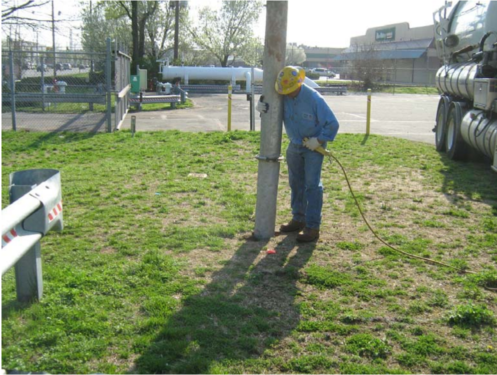
Photo 5: Vacuum excavation of soil boring in the northern portion of the Site
