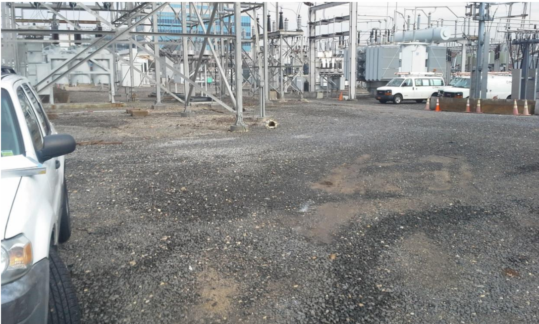
Northern area of proposed trench location showing Breaker 6100.
