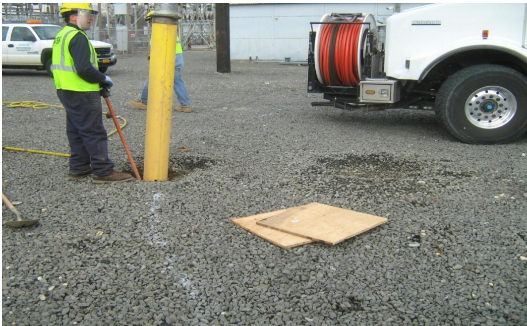
Vacuum excavation of soil borings at the westernmost area of proposed cable trench.
