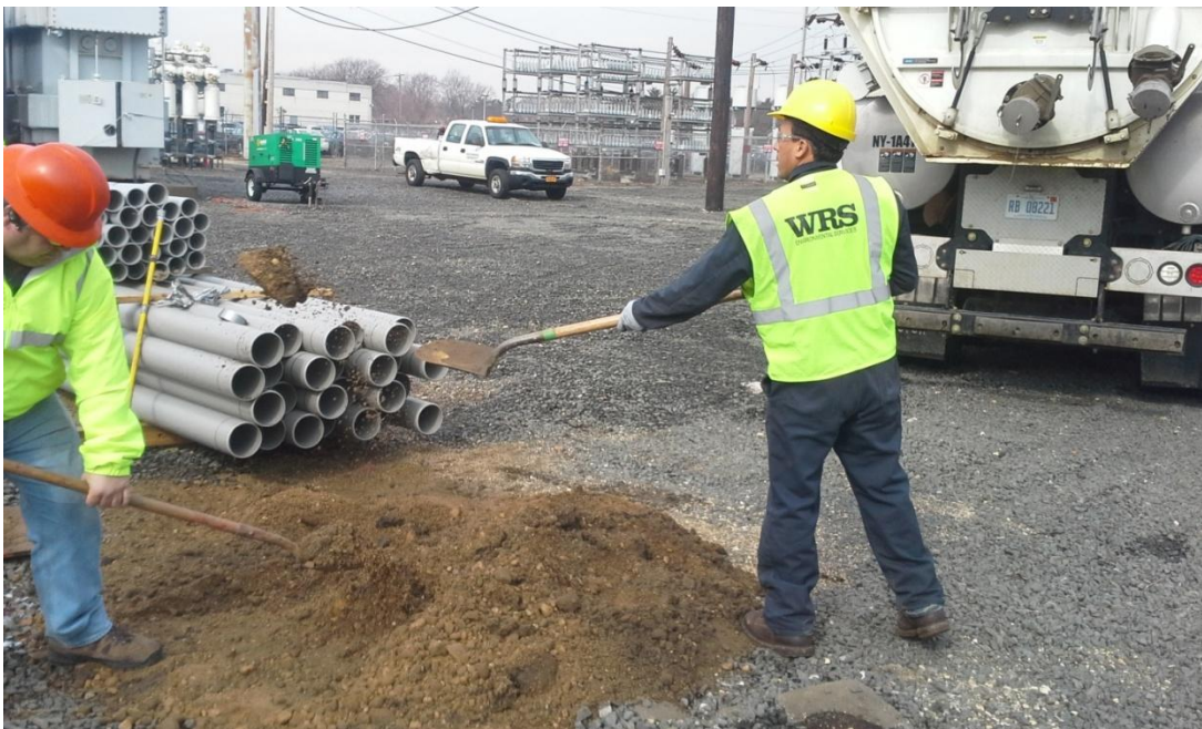
Backfilling of soil boring locations following soil sample collection.
