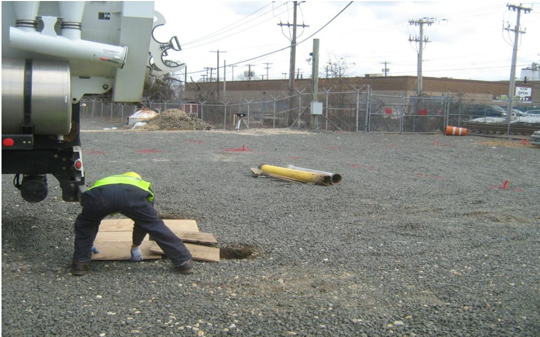
Workers temporarily covering soil boring prior to backfilling.
