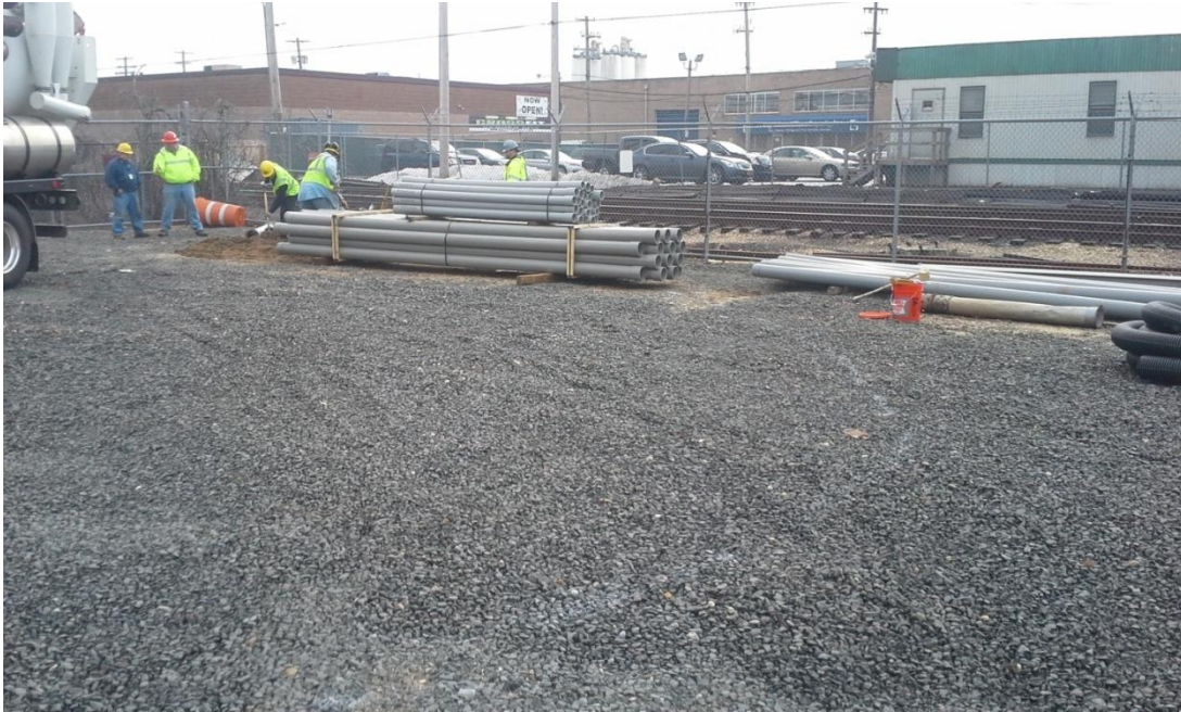
Southern area of proposed cable trench mark-out.
