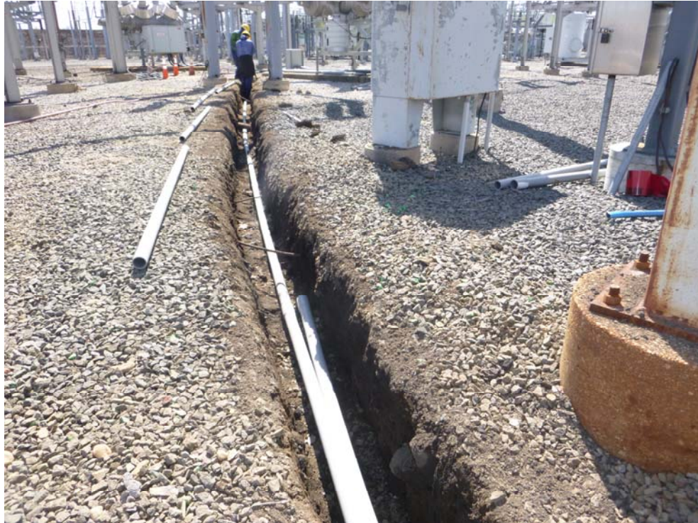
Photo 2: Installation of conduit and new below-grade electric cable within excavation.
