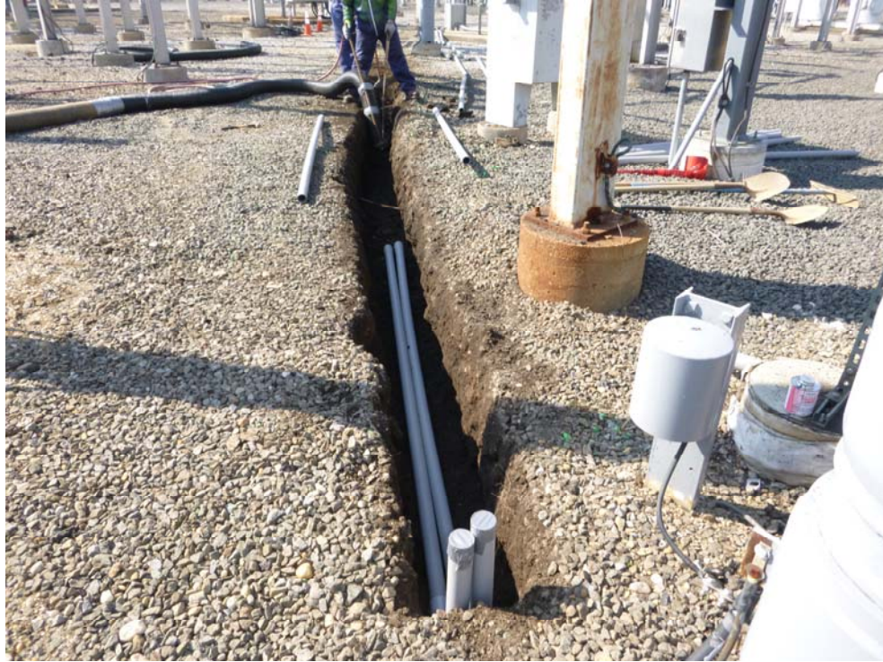
Photo 1: Excavation of the northeast cable trench utilizing guzzler vacuum extraction technology.
