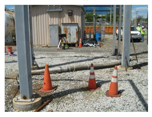
Photo 2: Downwind air monitoring station and vacuum extraction piping
