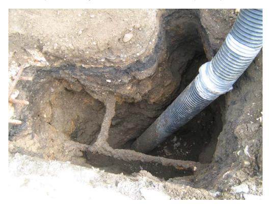
Photo 4: Test pit EGCTP-01 excavation showing black stained soil
