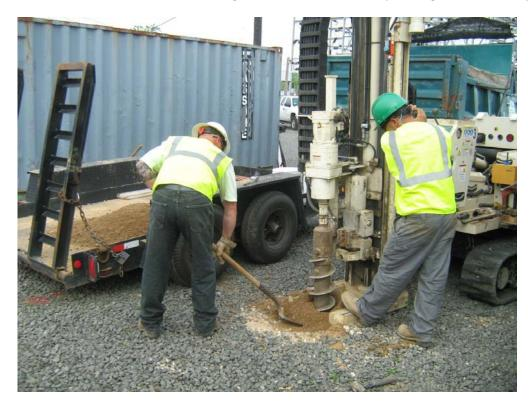
Photo 10: Installation of groundwater monitoring well EGCMW-05 utilizing a hollow stem auger rig
