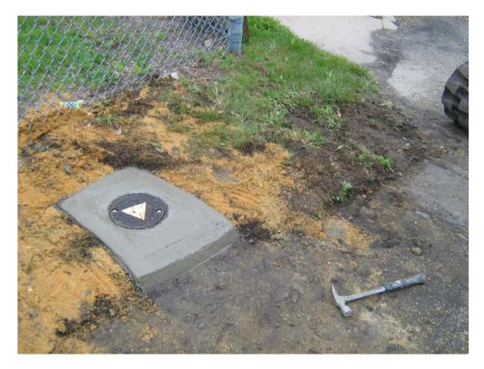
Photo 11: Completed groundwater monitoring well EGCMW-02
