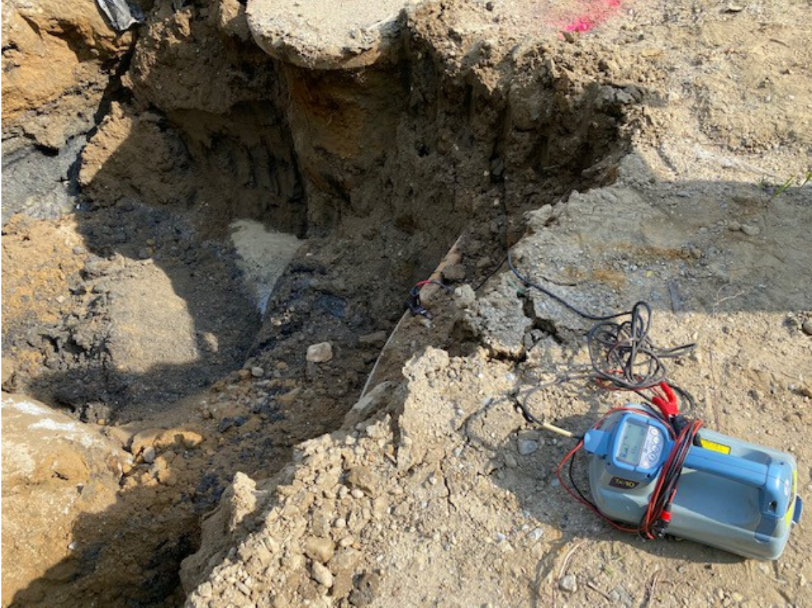
Figure 2: 36" diameter pipe at approximately 3' and a 2" diameter steel pipe at 1ft.
