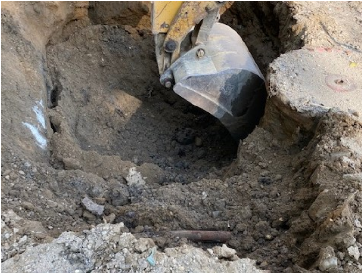
Figure 1: 36" diameter pipe at approximately 3' and a 2" diameter steel pipe at 1ft.
