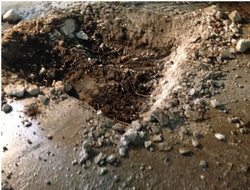
Figure 8, View of north excavation top of contamination
