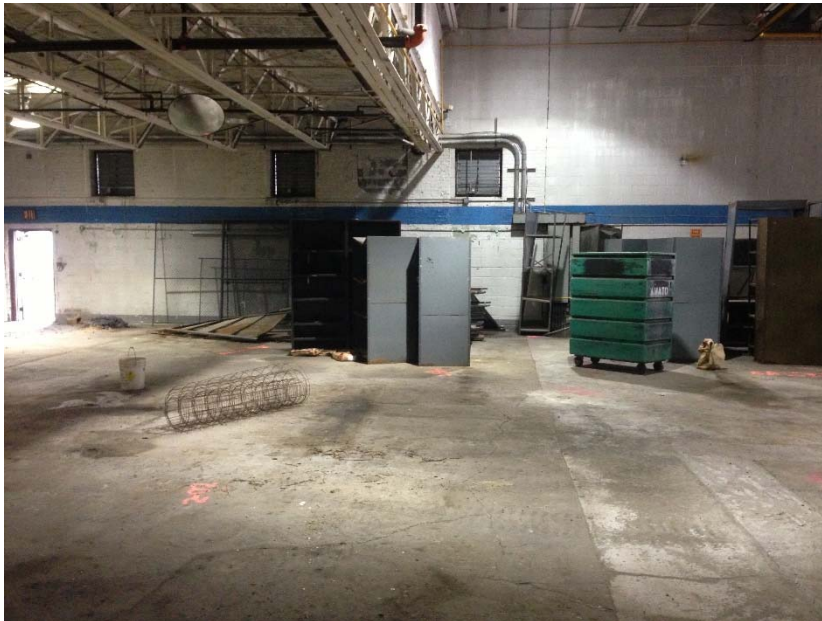
Figure 1, View of south hot spot prior to excavation
