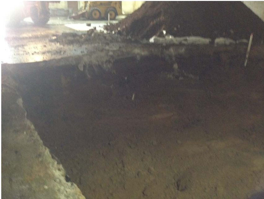
Figure 5, View of south excavation looking north
