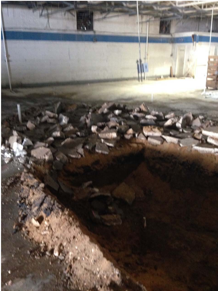
Figure 3, View of south excavation
