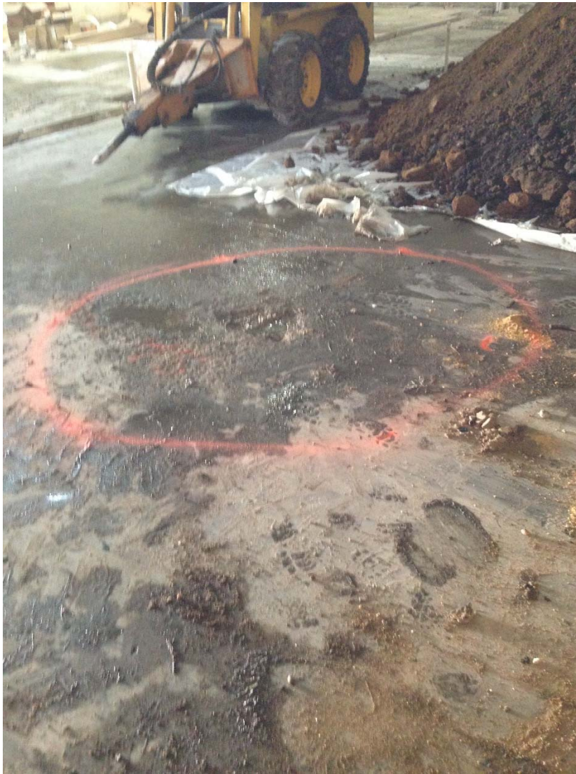
Figure 7, View of north hot spot prior to excavation
