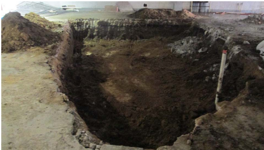
Figure 6, View of south excavation completed
