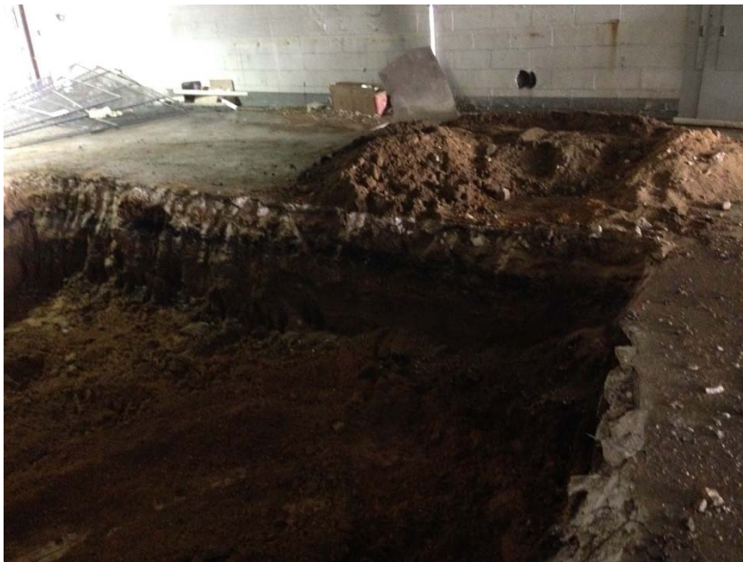
Figure 4, View of south excavation looking west
