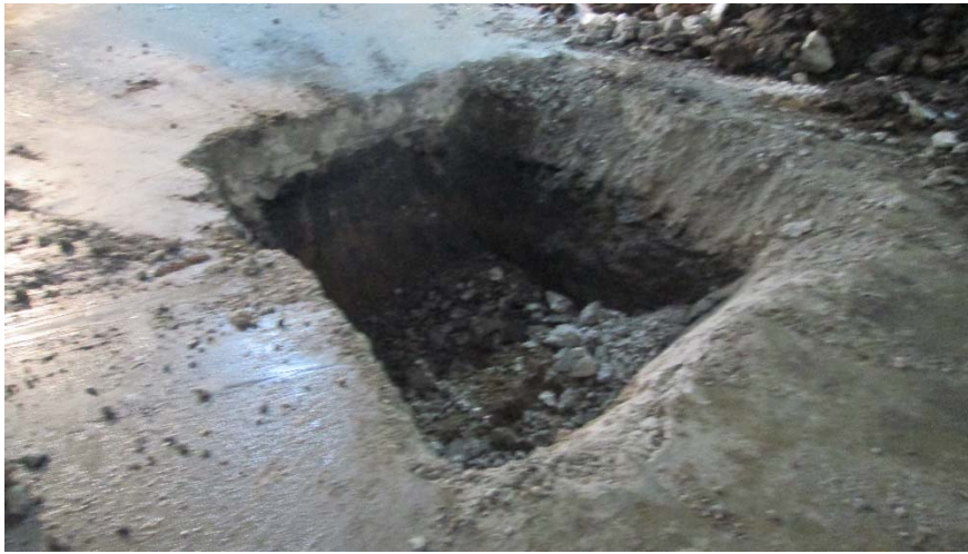
Figure 9, View of north excavation completed
