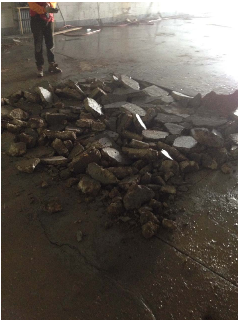
Figure 2, View of south excavation, concrete removal
